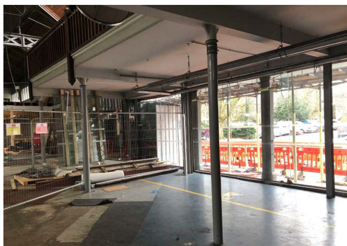
Figure 90: Examples of the c1909 cast iron mezzanine columns to the south elevation.
