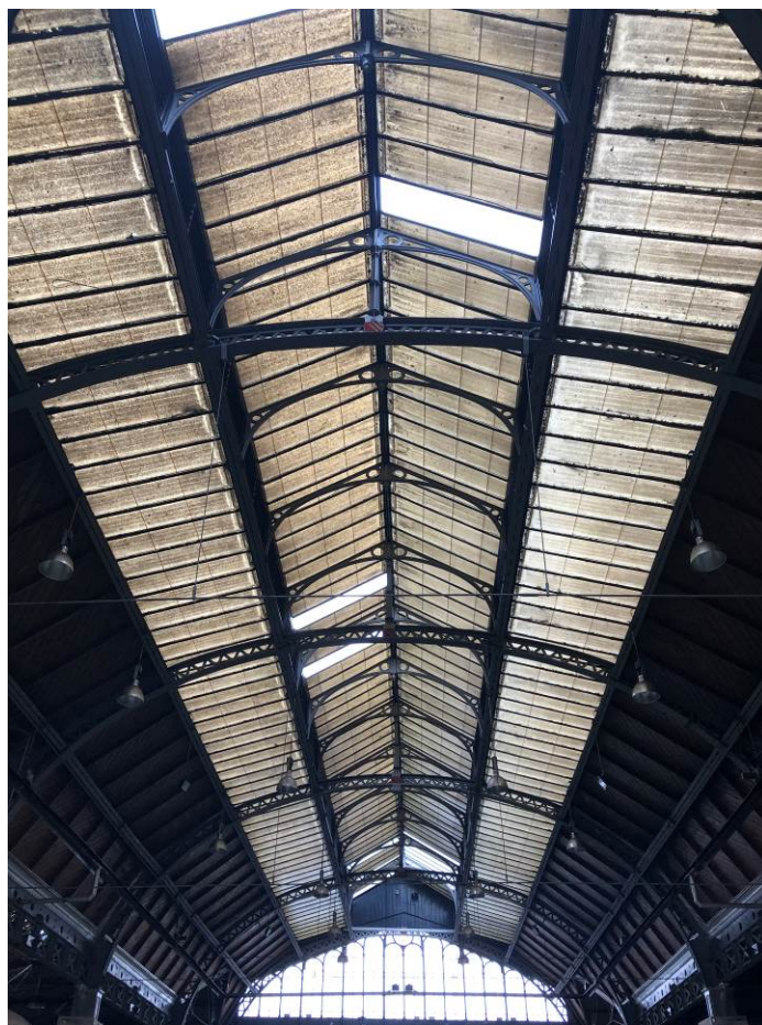
Figure 105: Looking west along the length of the roof structure.
