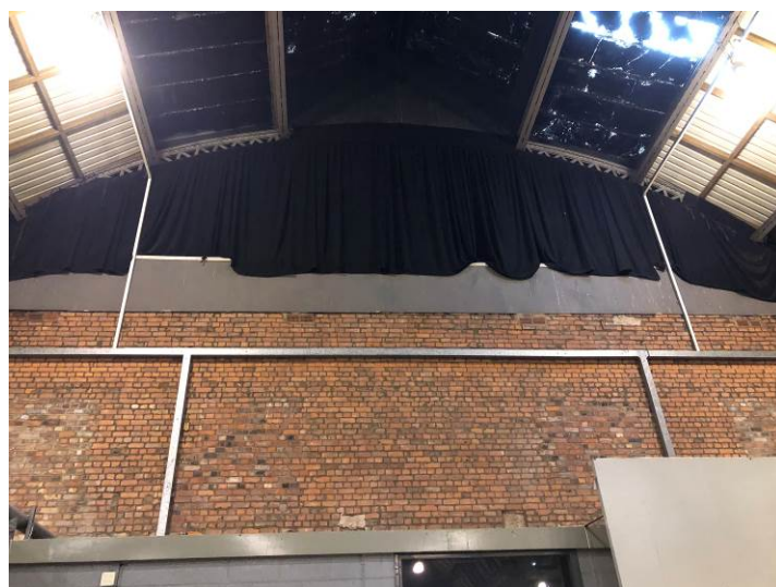
Figure 71: The upper part of the east elevation, showing the modern curtains concealing the original glazed gable.
