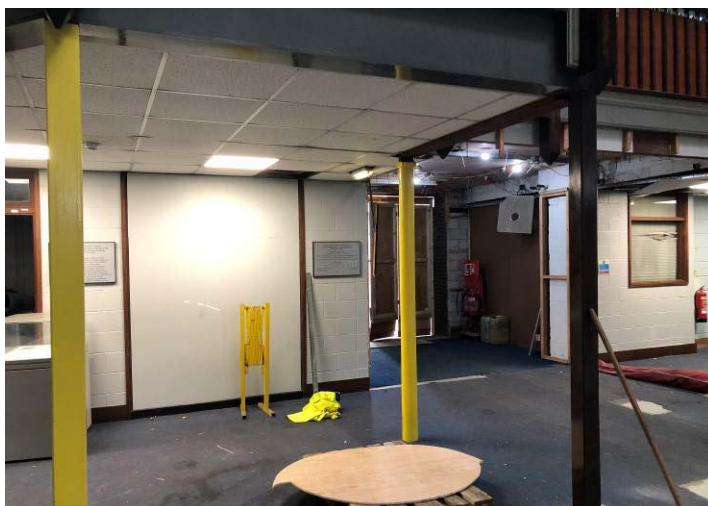
Figure 99: Modern 1980s structures along the east elevation.
