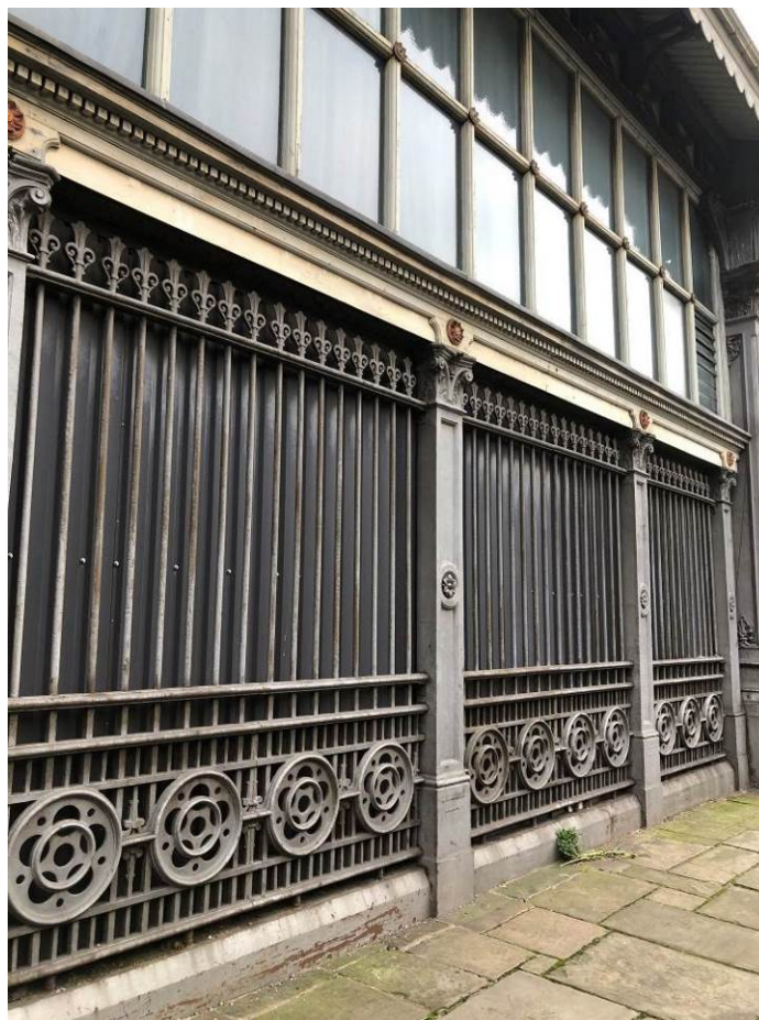
Figure 50: The southern section of the west elevation on Barton Street, showing the only examples of surviving original cast iron railings to the bottom parts.
