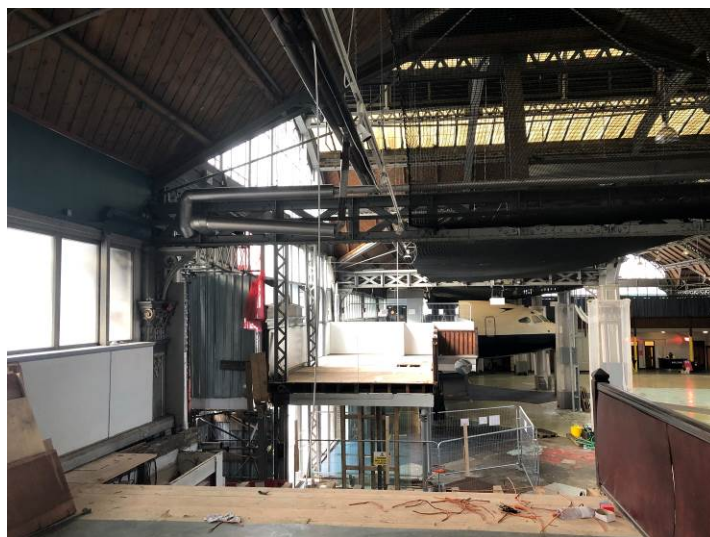
Figure 106: Looking west along the southern mezzanine
