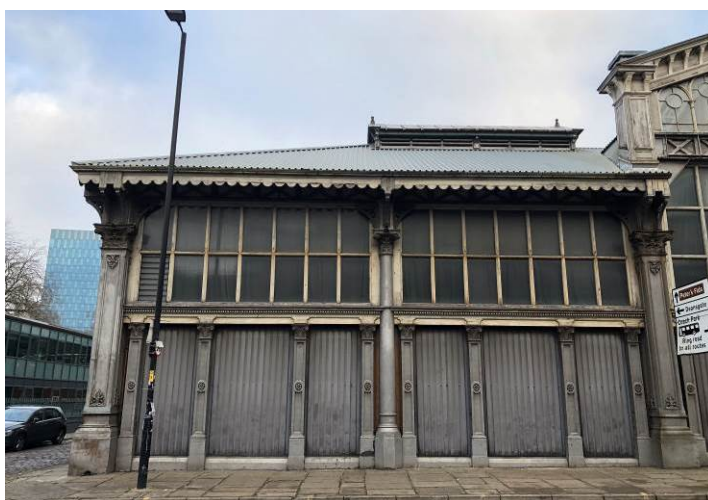
Figure 42: The western section of the south elevation, showing the original cast iron structure and glazed upper framework. The lower parts have had their cast iron railings removed and replaced with modern corrugated metal sheeting.
