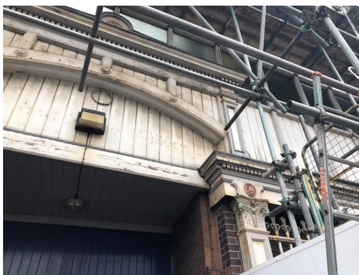
Figure 82: The lower parts of the west elevation.
