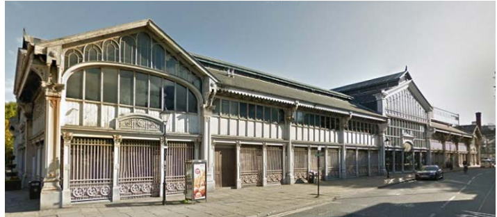
Figure 76: The southern elevation of the Lower Campfield Market as seen from Liverpool Road. (2018)
