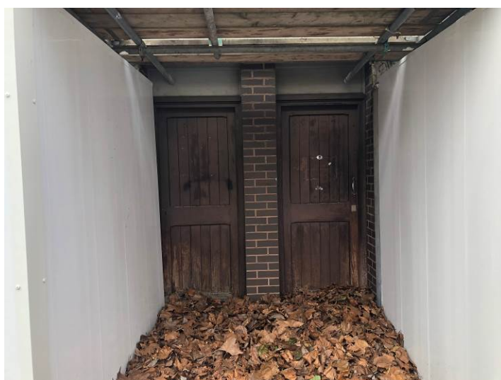
Figure 86: Examples of 1980-3 doors to the east elevation.
