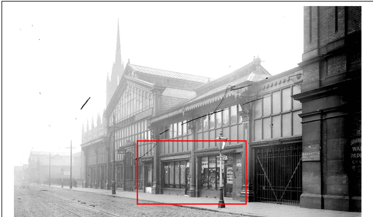
Figure 16a: The Upper Campfield Market as seen from Liverpool Road in 1914, showing the three ground floor shop units (outlined) which were constructed under the new Commercial Produce Auction Sales Room in 1894 (Source: Manchester Archives).
