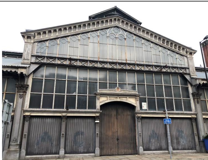
Figure 43: The central section of the south elevation, showing the original glazed framework with modern corrugated metal sheeting and gates.
