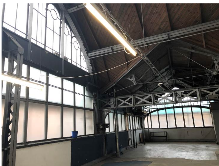
Figure 111: Looking north along the western mezzanine.
