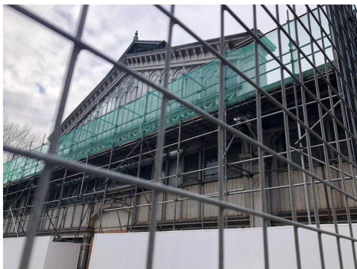
Figure 85: The east elevation.
