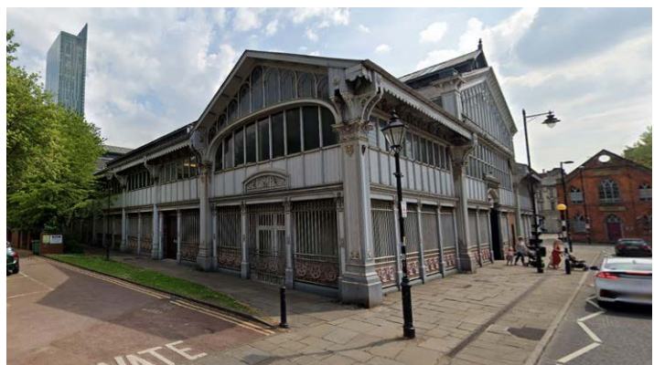
Figure 78: The north elevation as seen from Lower Byrom Street. (2018)
