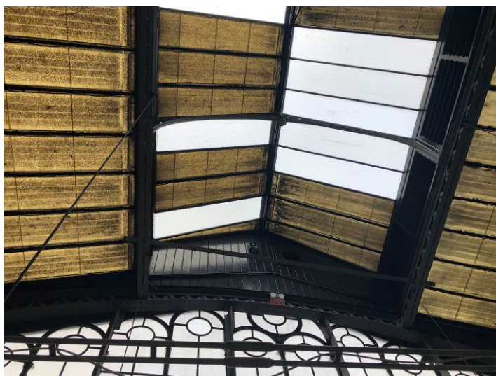
Figure 103: An example of the modern 1980s fibreglass panels (discoloured) and more recent clear coverings.
