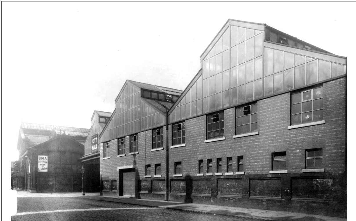
Figure 31: The newly completed City Hall extension (right) seen looking south from Byrom Street in c1927. The original part of the City Hall can be seen to the far left. (Source: Manchester Archives)
