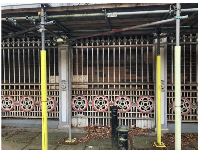
Figure 79-80: Examples of the original sliding gates to the north elevation. Note the wheels (bottom) and lock protection plates (centre).
