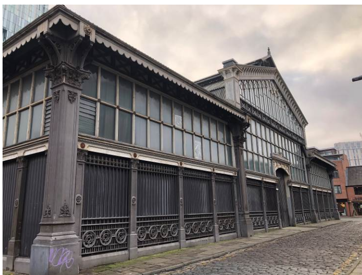
Figure 48: The west elevation on Barton Street, showing the only examples of surviving original cast iron railings to the bottom parts.
