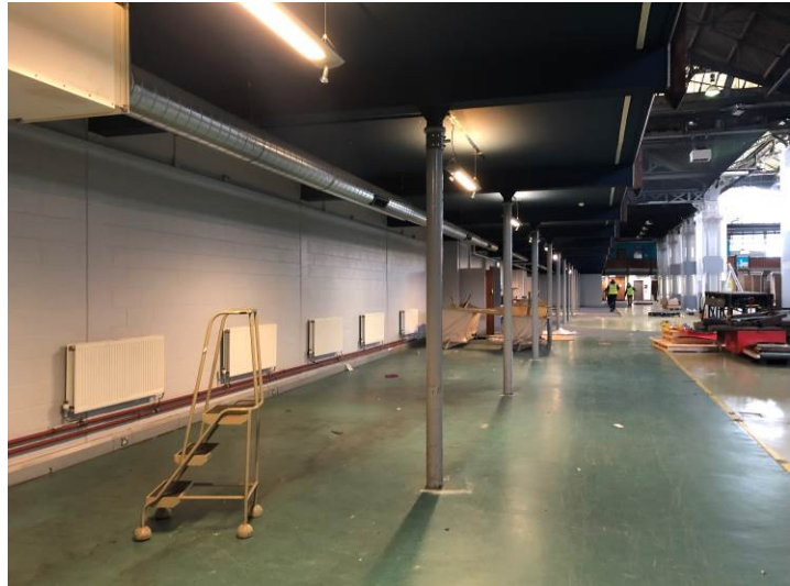
Figure 93: Looking east along the northern elevation beneath the mezzanine.
