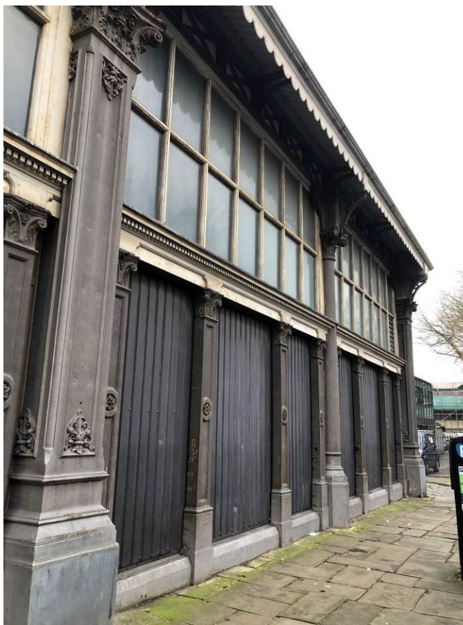
Figure 47: The western part of the north elevation, showing the modern corrugated sheeting replacing the original cast iron railings, with original timber and glazed framework above.
