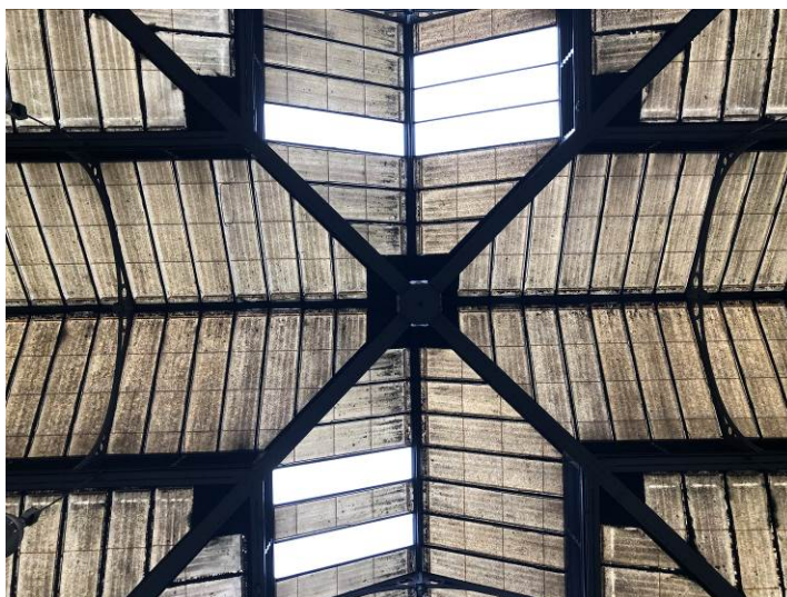
Figure 104: An example of the modern 1980s fibreglass panels (discoloured) and more recent clear coverings to the centre of the roof.
