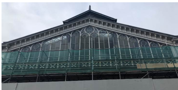
Figure 82: The central glazed Venetian windows to the east elevation.
