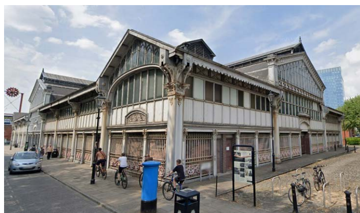
Figure 84: The south elevation (left) and east elevation (right) (2018)
