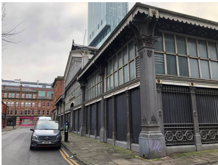
Figure 45: Looking east along Tonman Street along the northern elevation of the building.
