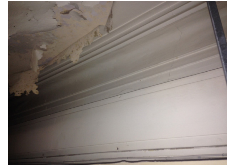
existing cornices hidden above suspended ceiling
