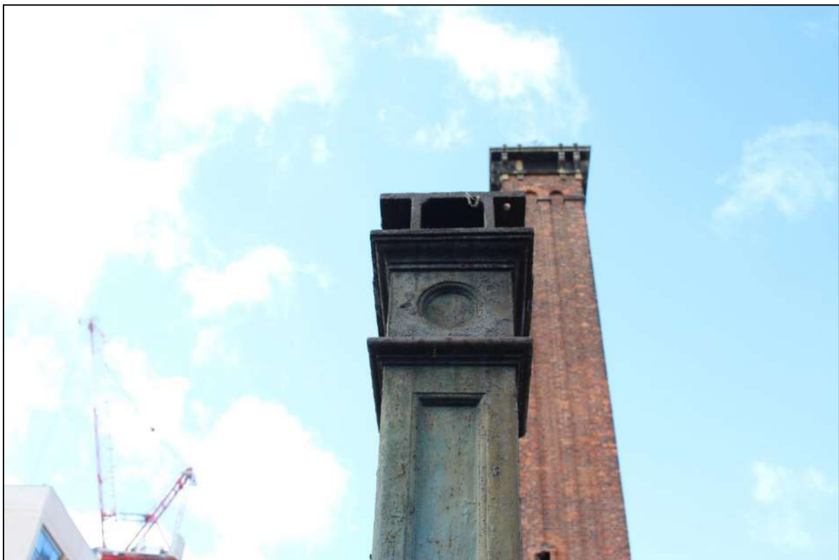
Plate 28: Detail of one of the capitals to the columns
