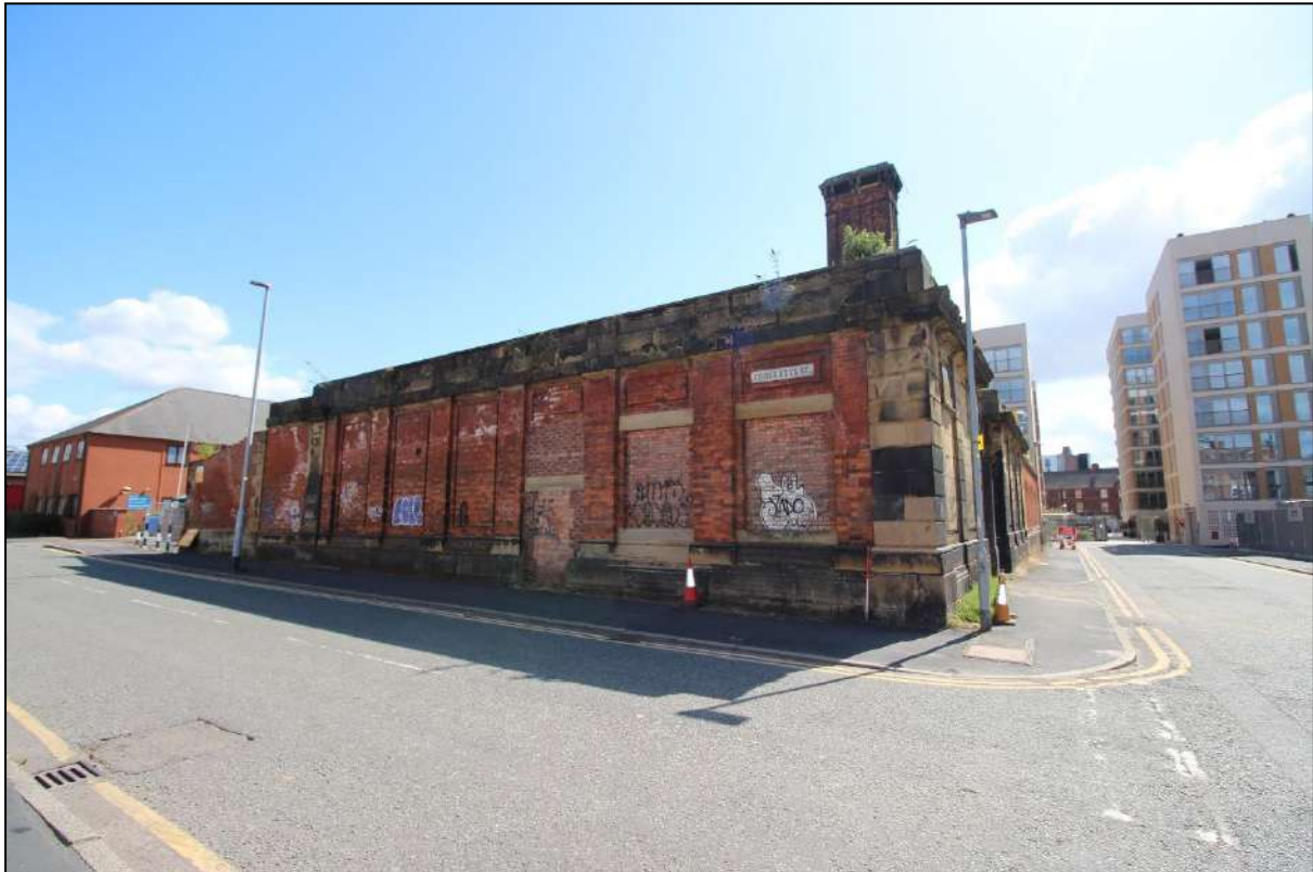
Plate 16: General view north-west elevation fronting Cross Keys Street
