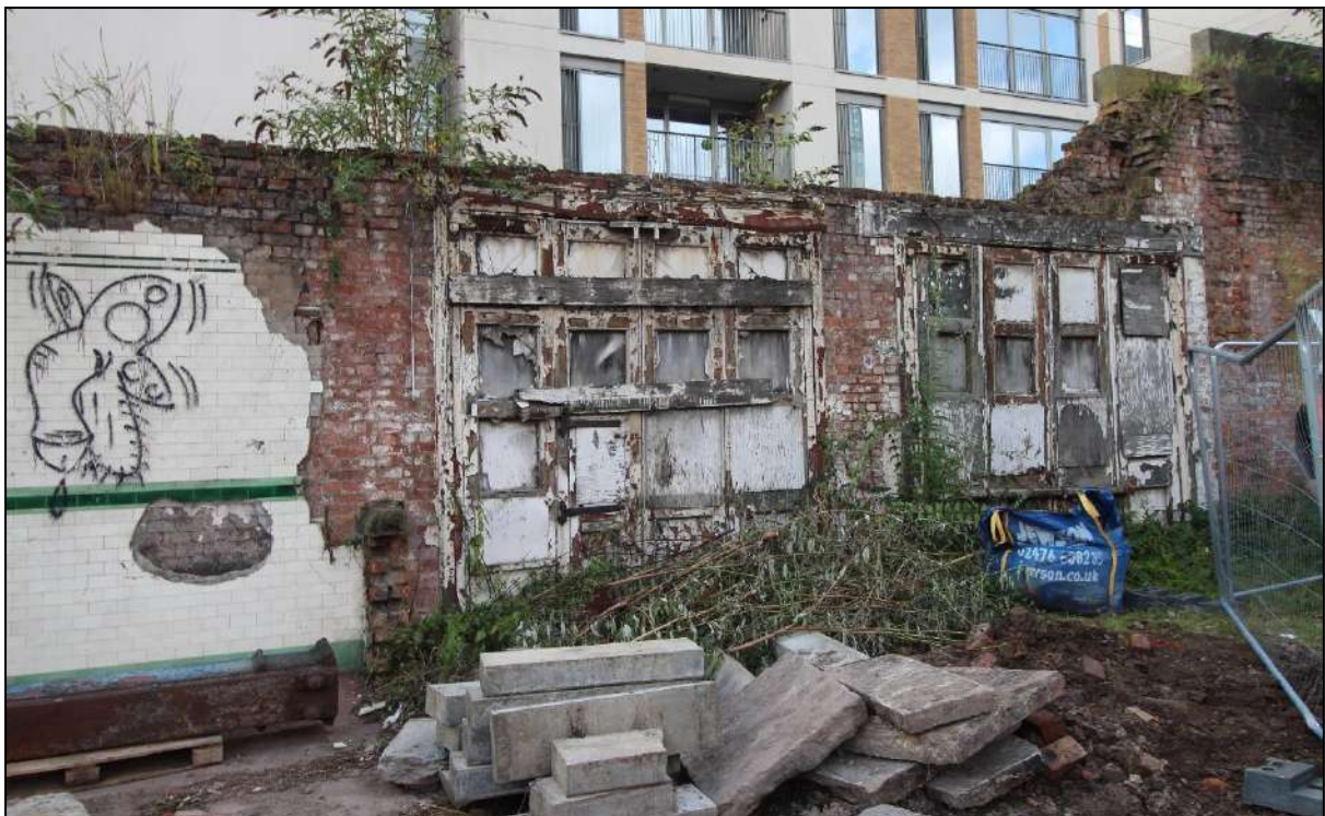
Plate 38: The large vehicle doorways at the centre of the south-east wall
