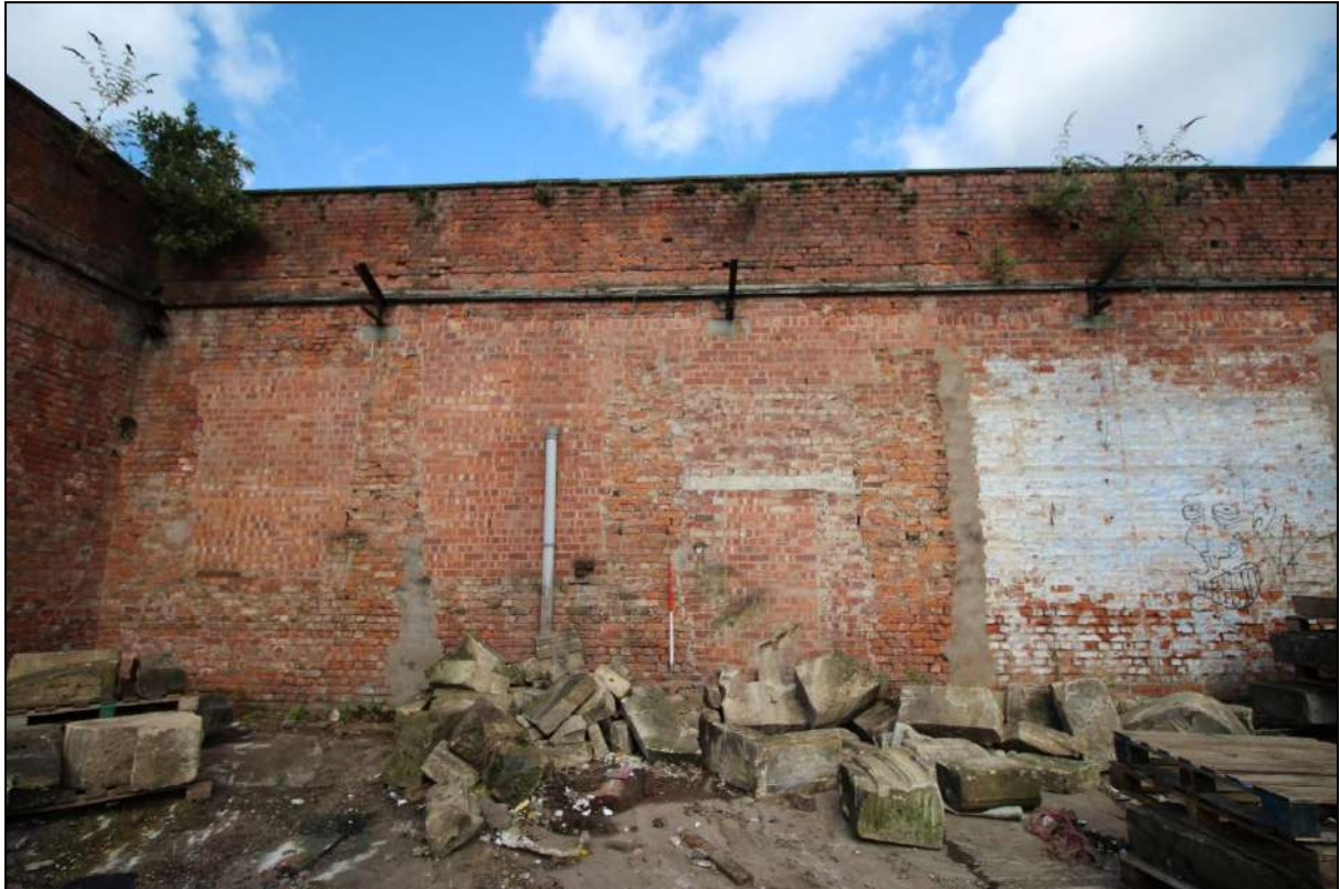
Plate 41: Detail of the blocked doorway and windows within the north-western wall
