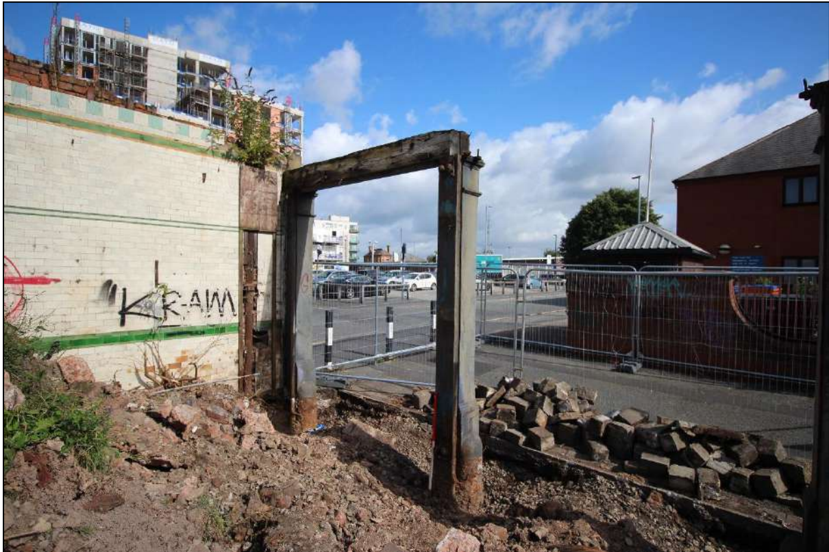
Plate 29: The two columns at the north-western end with the only surviving timber lintel
