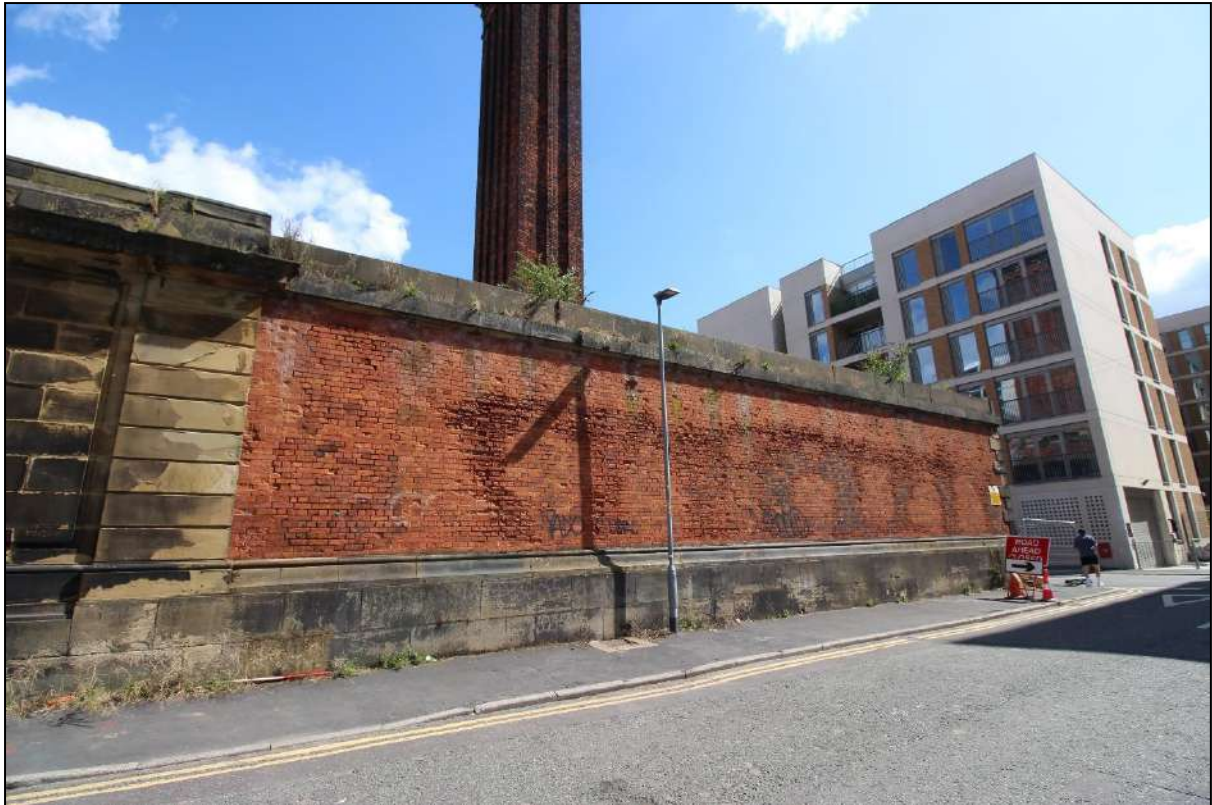
Plate 21: The English bond brick section at the south-eastern end of the elevation
