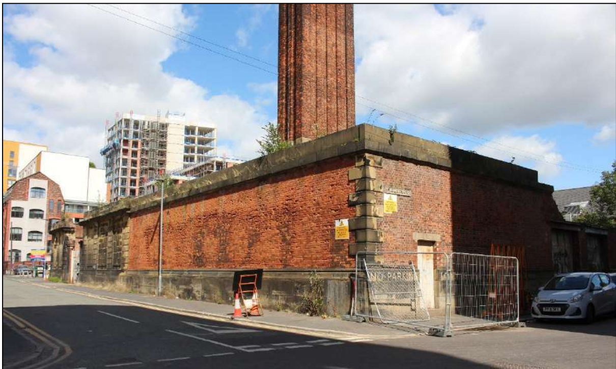
Plate 18: General view south-west elevation fronting Goulden Street
