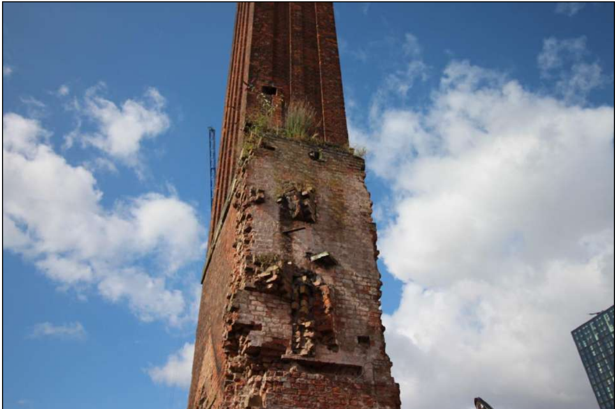
Plate 31: Detail of the remains of the fireplaces on the first-floor level to the north-east elevation
