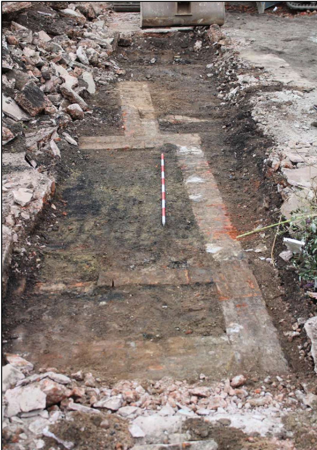
Plate 43: A general shot of Trench 2, illustrating several of the brick walls exposed in-plan. Photograph looking southeast with a 2m scale
