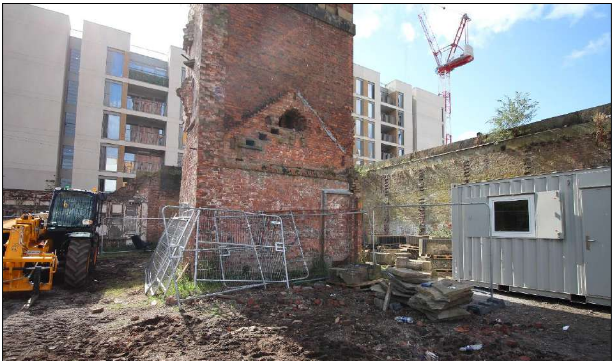
Plate 32: The north-western elevation of the chimney
