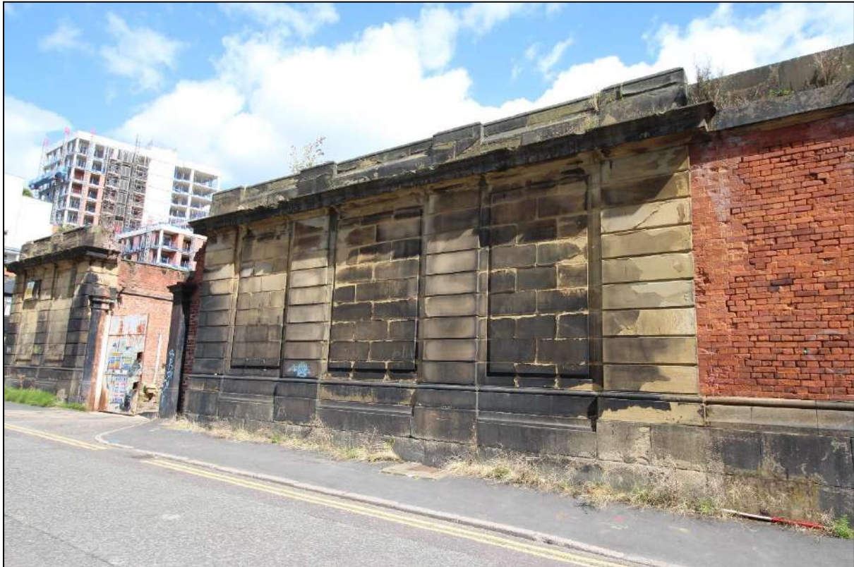
Plate 19: The sandstone recessed panels to the north-western end of the elevation
