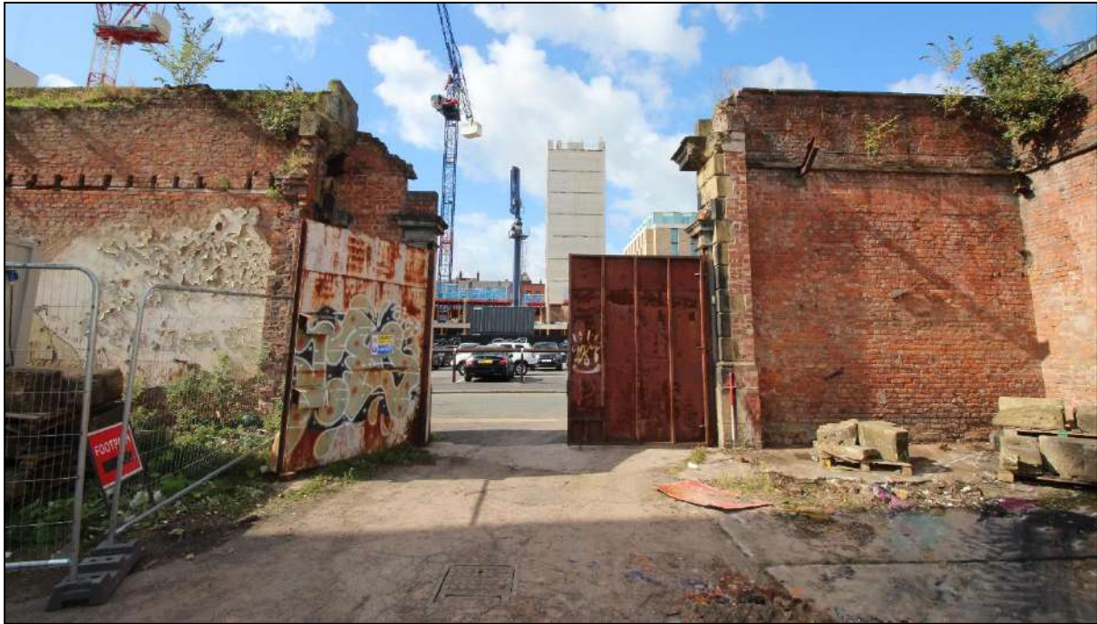
Plate 35: The principal entrance into the station
