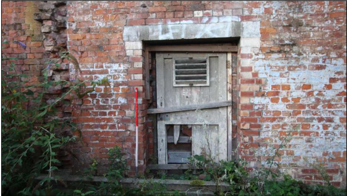
Plate 37: The south-western doorway within the south-east wall
