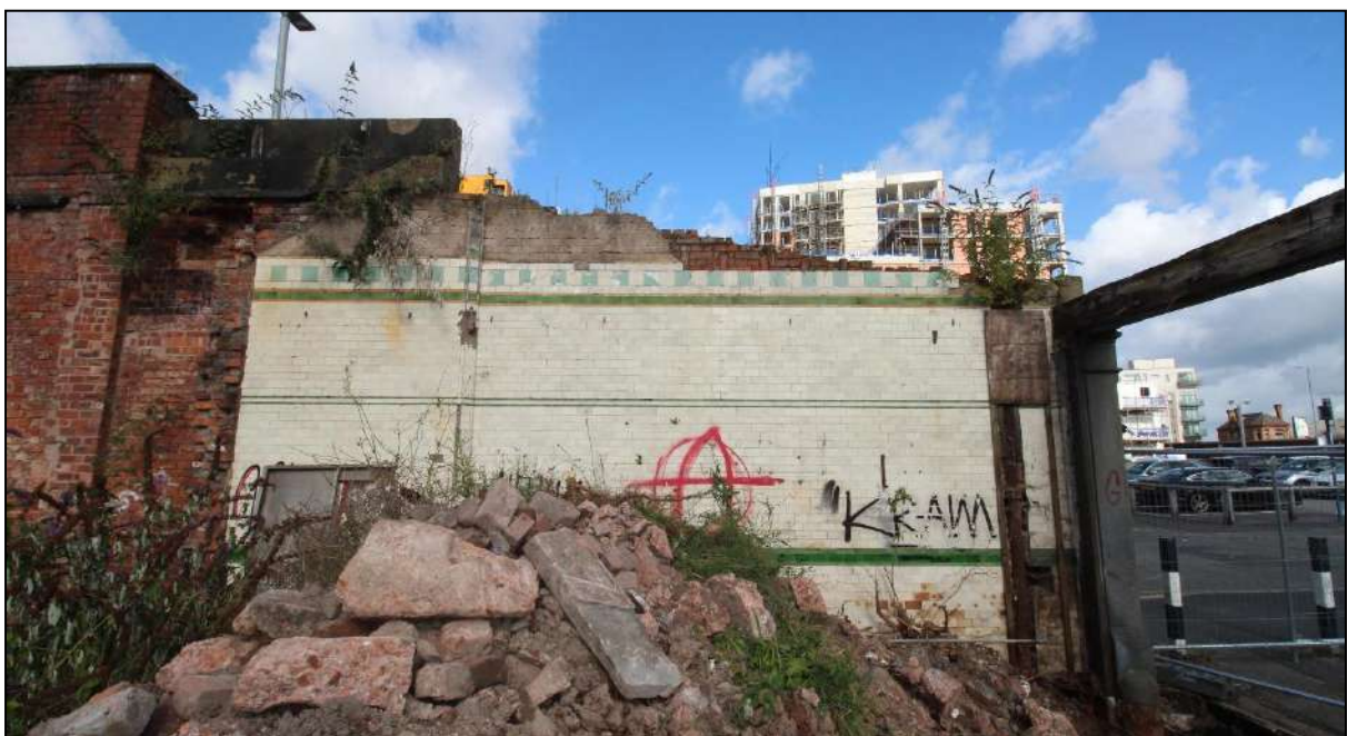
Plate 40: The north-eastern end of the north-west wall
