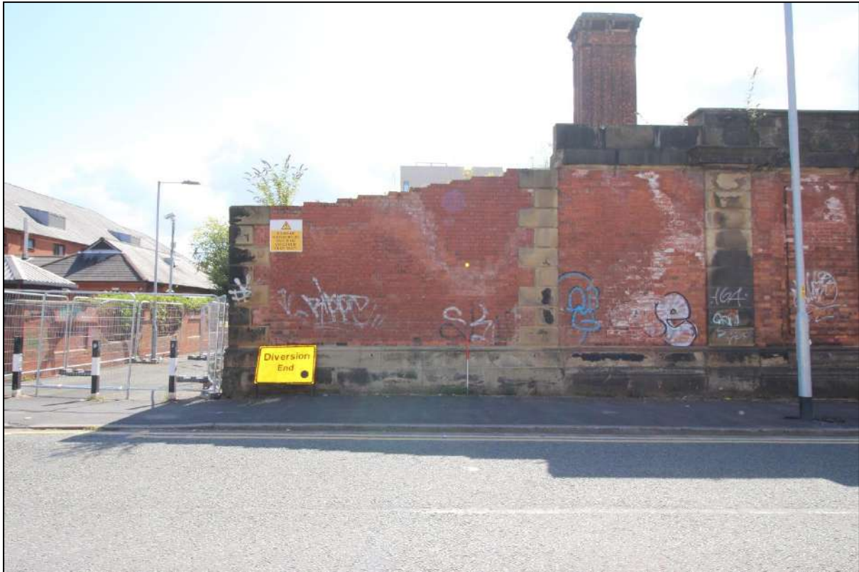
Plate 17: Detail of the remains of the Engine and Stable north-west gable
