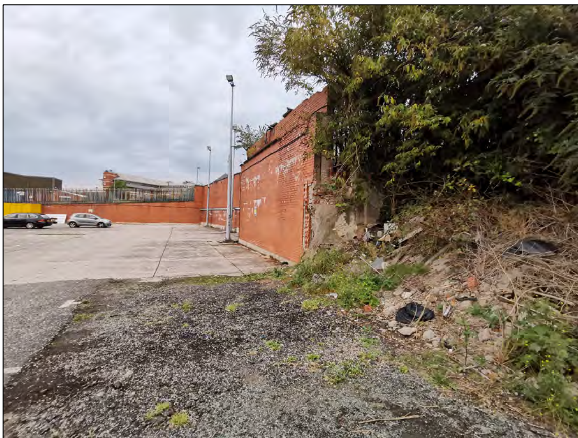
Plate 21: Remnants of 20 th -century walls to the north-east of the Site
