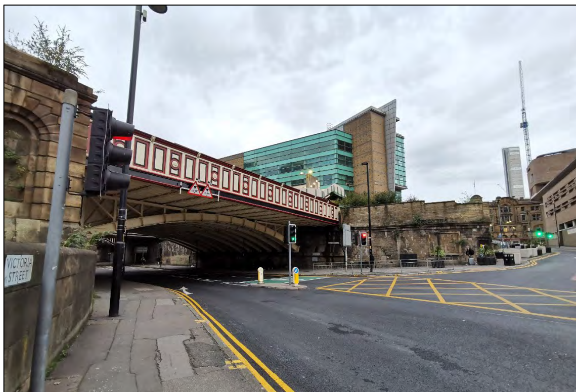
Plate 40: View of Stephenson Bridge from Victoria Street and Victoria Station to the right, looking north-east
