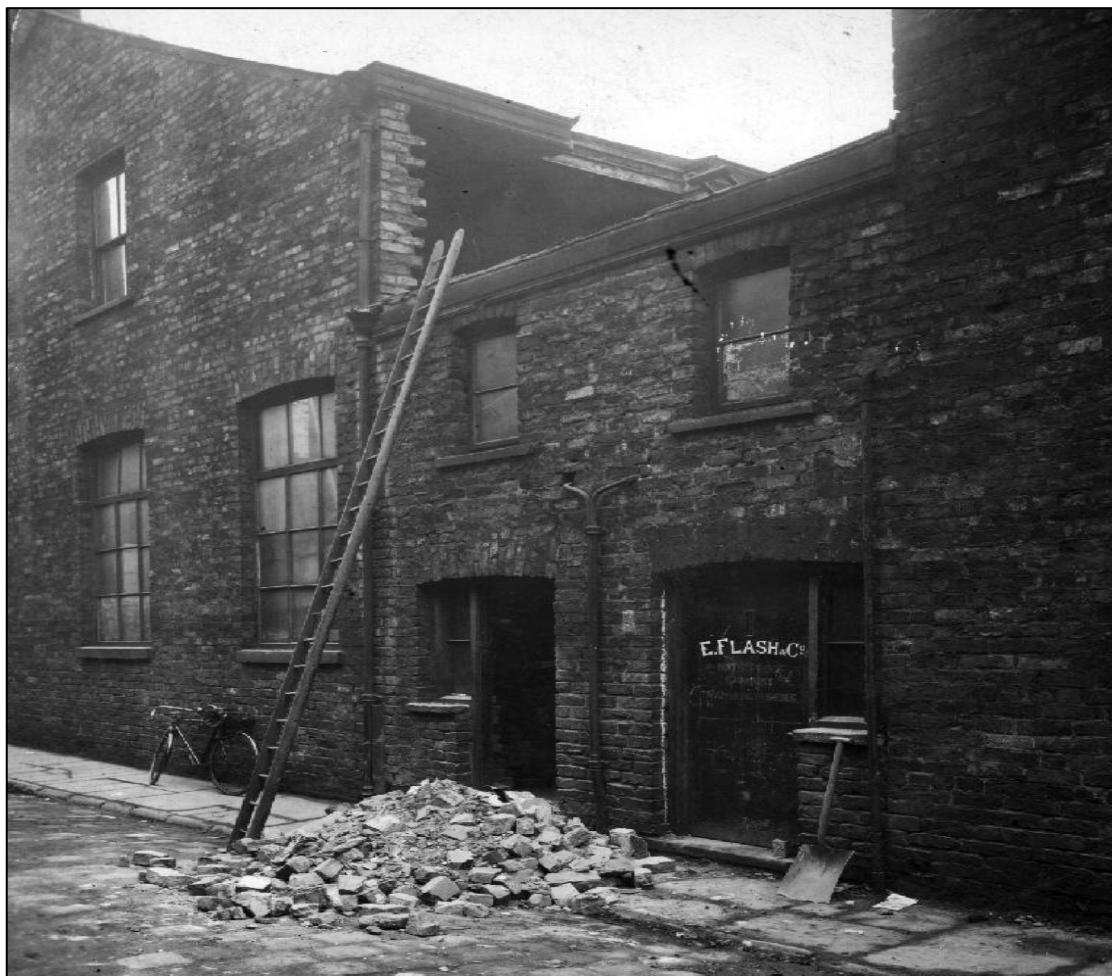
Plate 12: Photograph taken of Nightingale Street in 1920, courtesy of Manchester Local Image Collection
