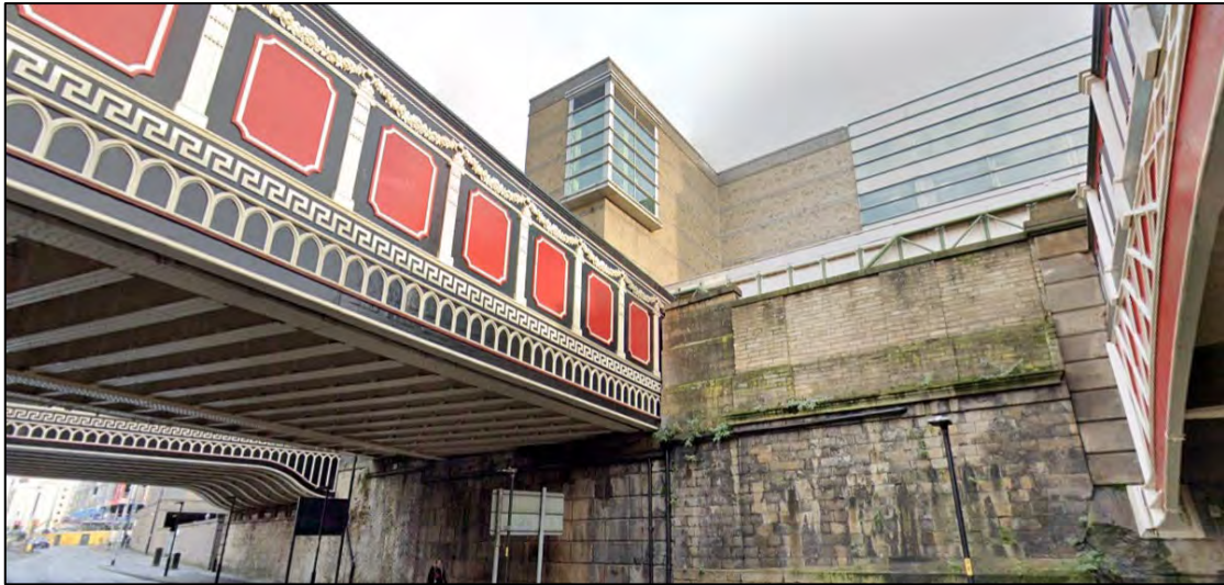
Plate 41: Middle Bridge, looking east
