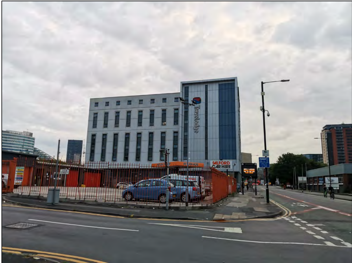
Plate 31: Looking in the direction of North Bridge from the Site
