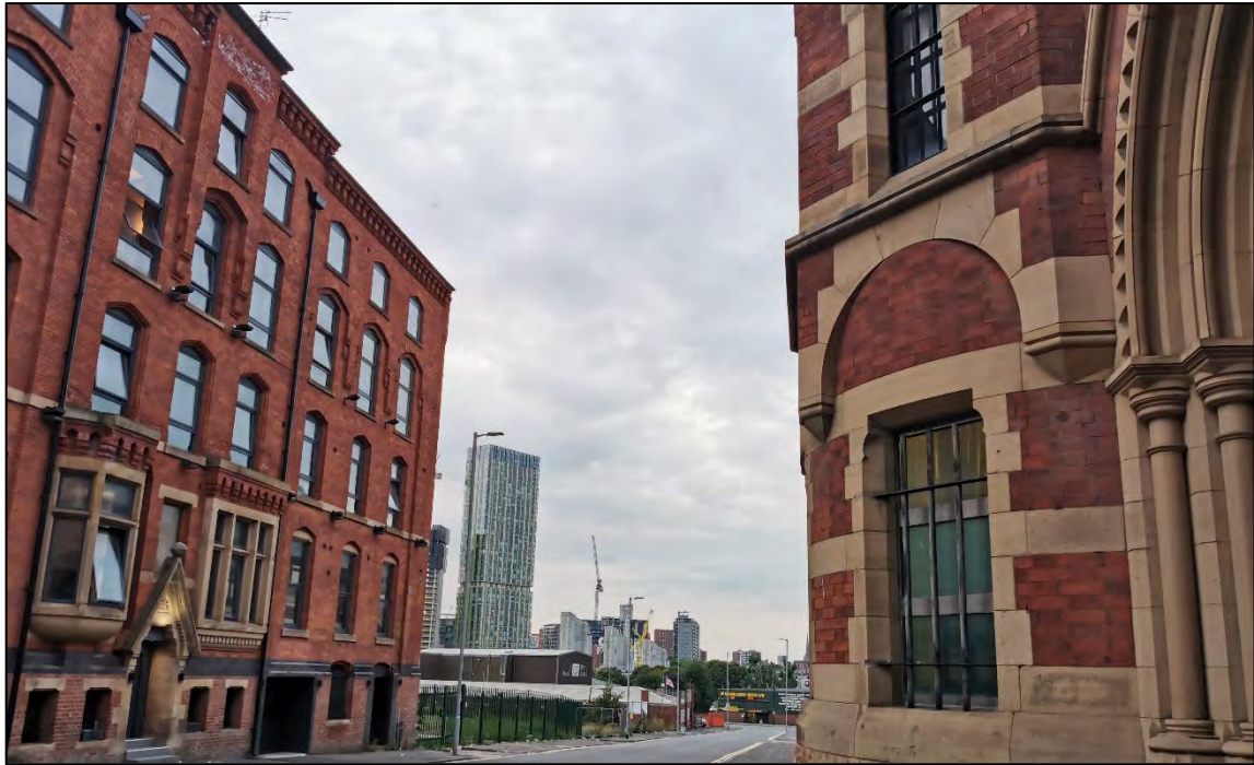
Plate 25: View of the Former Globe Works, looking west towards the Site
