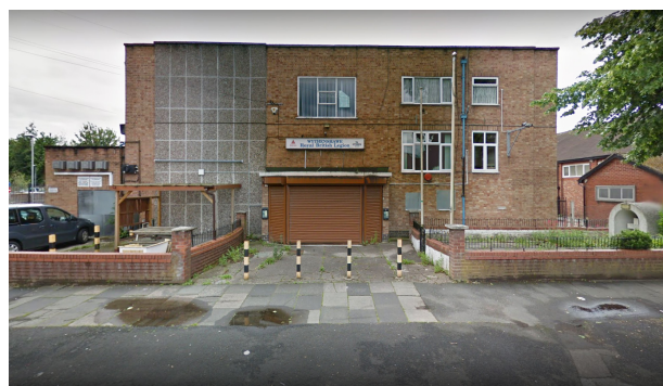
Fig 2. The Royal British Legion, prior to demolition.
