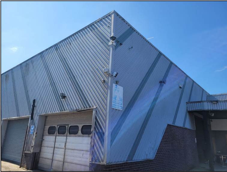
Photograph 4 Building 2 metal housing
