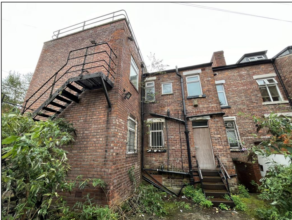
Figure 2. Rear of property
