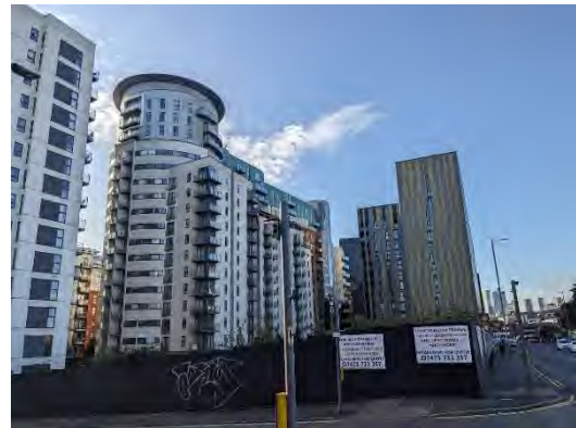
Figure 31: Tall residential development to east of the Site and within the neighbouring SRF.
