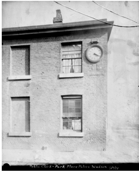
Figure 15: Clock on elevation of former residences, converted to Police and Fire Station, Park Place, 1899. Source: Greater Manchester Lives online archive Ref. m78514
