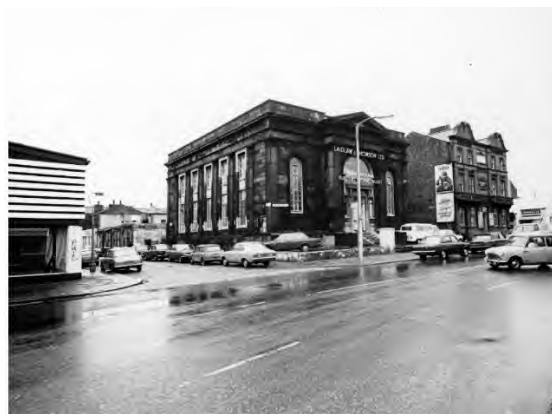
Figure 23: The Site is seen at the far right of the photograph in conjunction with the former Methodist chapel and Northern Hospital wing on Cheetham Hill Road, all apparently serving commercial purposes, 1972. Source: Greater Manchester Lives online archive, Ref. m71659.
