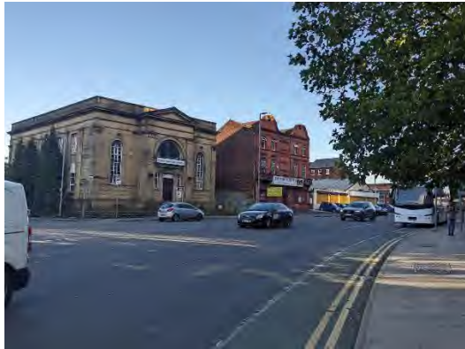
Figure 24: View of the Site from Cheetham Hill Road in conjunction with Grade II listed Former Synagogue (former Methodist chapel) and wing of the Northern Hospital at No. 21 Cheetham Hill Road.
