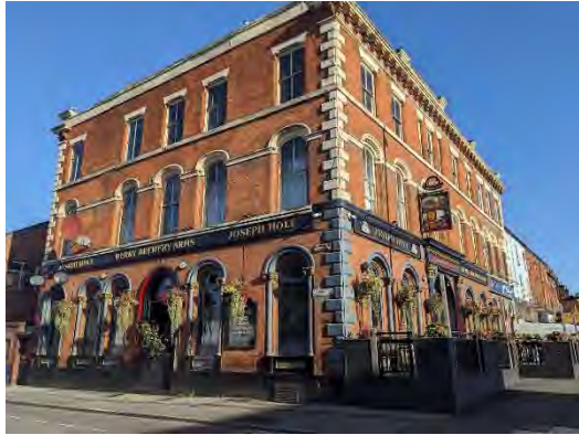
Figure 28: Grade II listed Knowsley Hotel, to the north of the Site.
