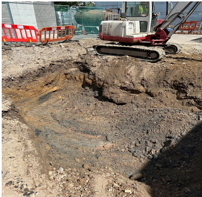
Photograph H – Image taken west of site facing north east. Image showing the clean uncontaminated ground in the location of the former tank after the excavating works.
