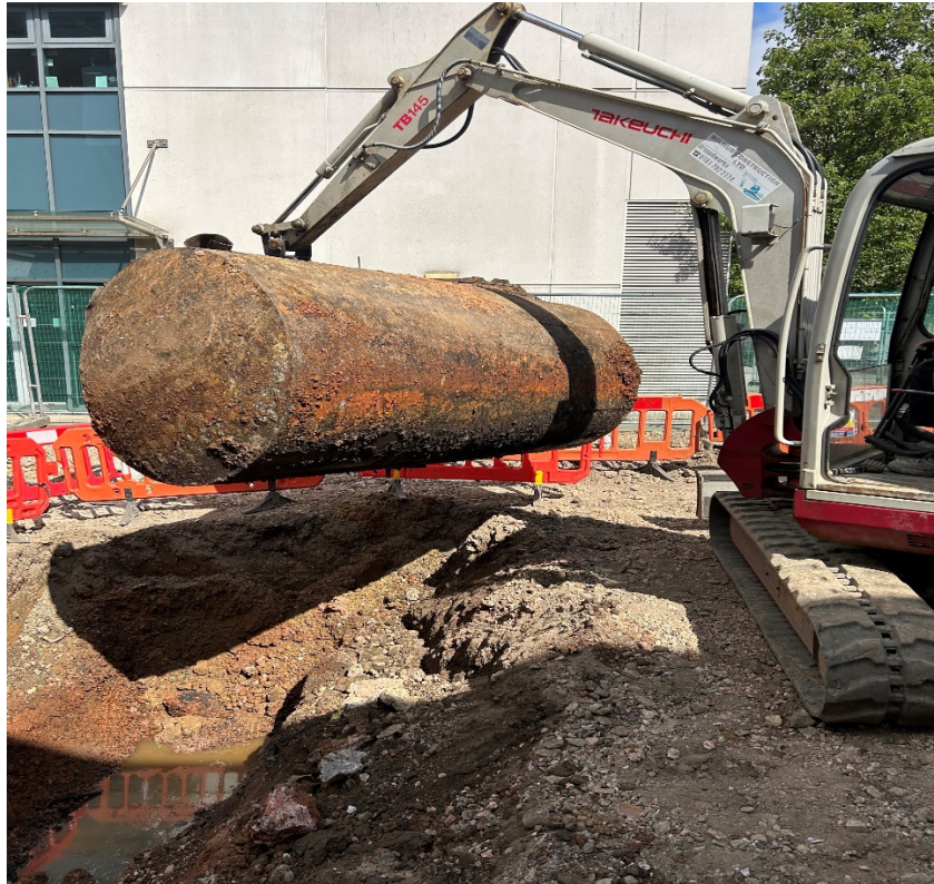
Photograph E – Image taken south of site facing north. Image showing the removal of the steel tank on site.
