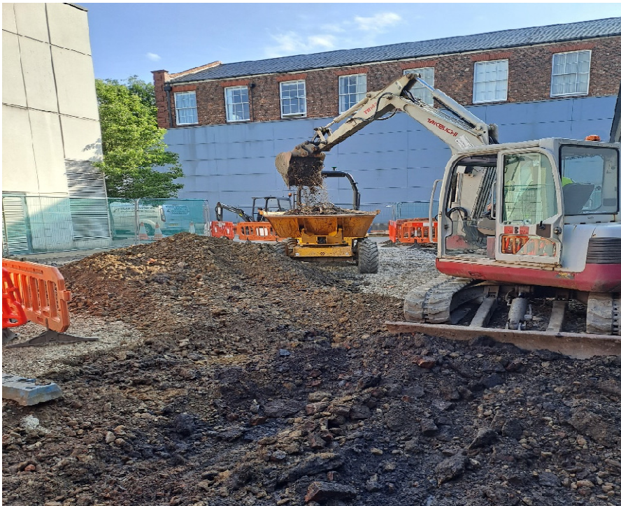
Photograph B – Image taken in the south western corner of the site facing east. Image showing the black hydrocarbon-impacted soils being excavated directly into a dumper headed for a offsite stockpile.
