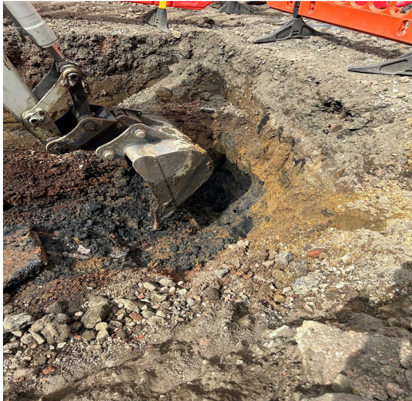
Photograph G – Image taken north east of site facing west. Image showing the resulting hydrocarbon impacted soils being excavated out after tank removal.
