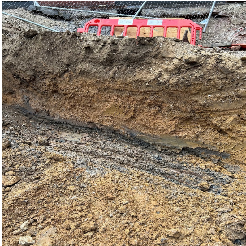
Photograph I – Image taken centre of site facing west. Image showing the clean uncontaminated ground in the location of the former tank after the excavating works.
