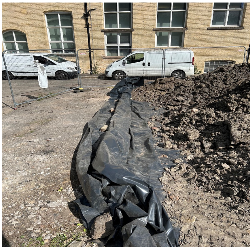
Photograph D – Image taken offsite. Image showing banded stockpile of contaminated soils ready for removal to landfill.
