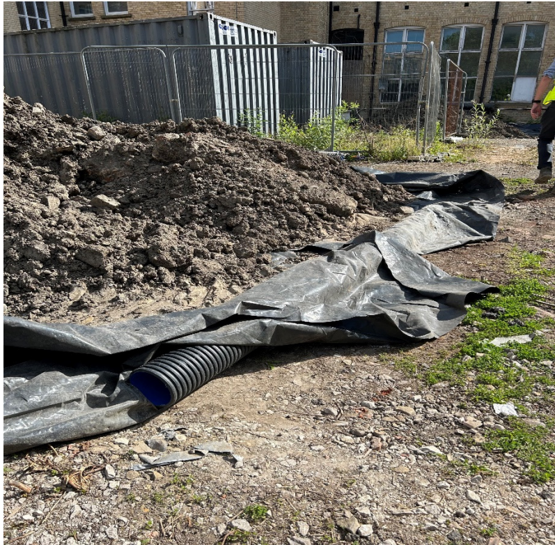
Photograph C – Image taken offsite. Image showing banded stockpile of contaminated soils ready for removal to landfill.
