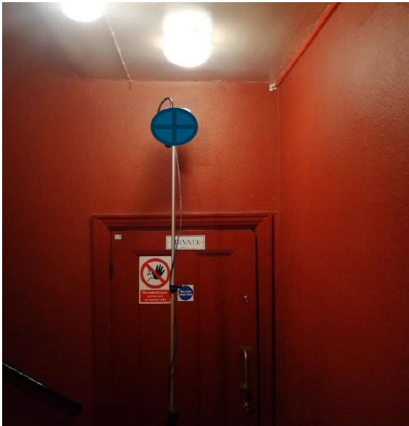
Location AP 12 - Foyer level - Unit is at high level and centered on the door.
