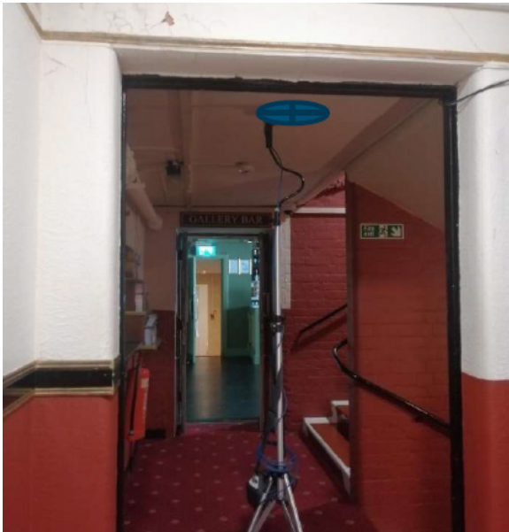
Location AP 32 - Lower Gallery Level - installed at high level and to be white. Conduit runs in close proximity.
