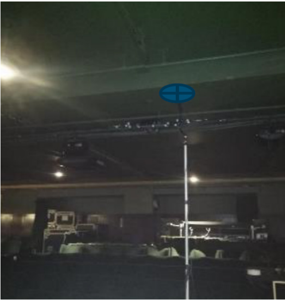
Location AP A11 - Stalls level - unit to be fixed to ceiling in close proximity to existing ceiling mounted services and cabling
