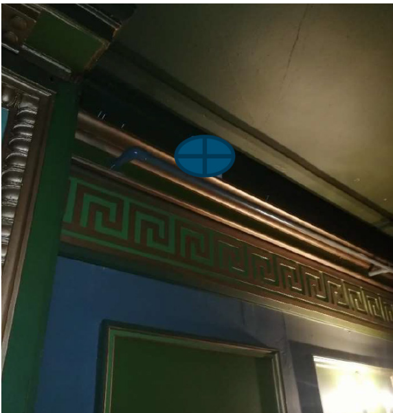
Location AP A4 - Stalls level - unit installed discreetly above cornice line. Conduit obscured.
