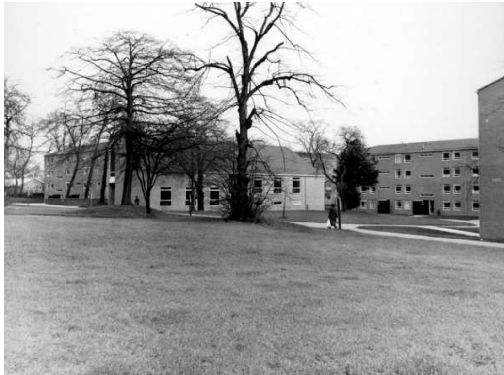
Figure 28: Accommodation blocks at Oak House, 1975
