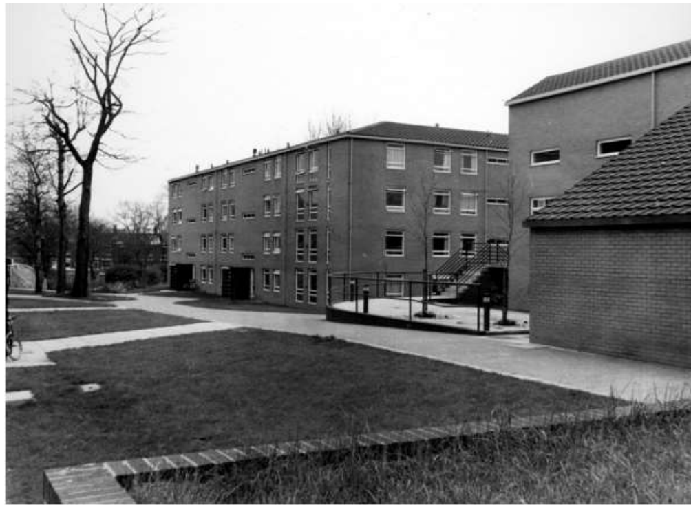
Figure 29: Accommodation blocks at Oak House, 1975
