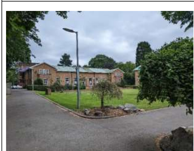
Figure 44: Buildings at Woolton Hall arranged around central green.
