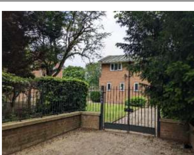
Figure 47: View across to Woolton Hall from Whitworth Lane.
