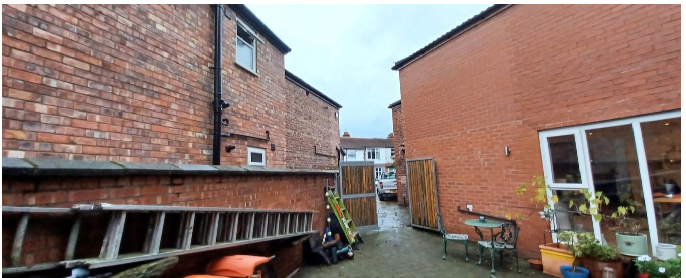
Figure 7. View along side of property.
