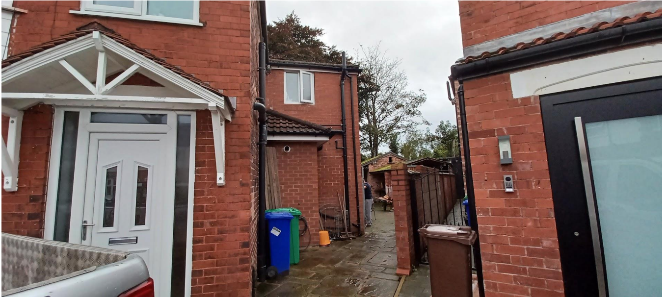
Figure 2. View along side of property.
