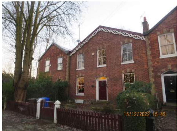
Front elevation showing adjoining houses
