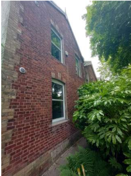
New windows in old reveals, front
