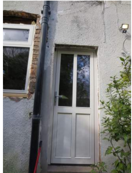
Rear kitchen door
