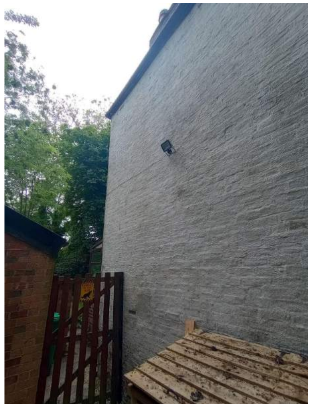
Side corner with rear elevation
