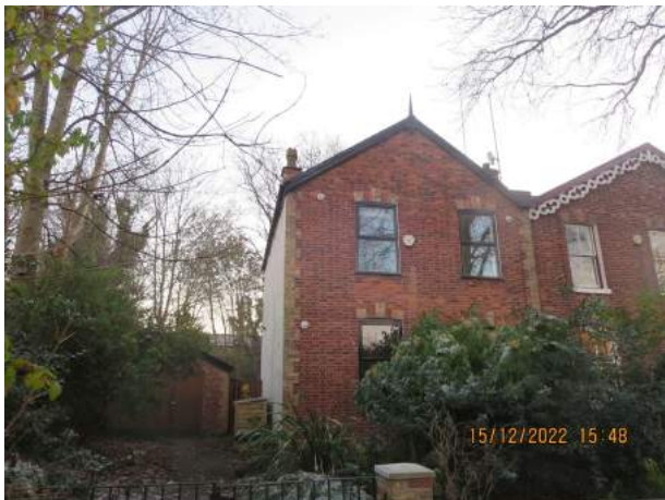
Front elevation from end of Limefield Terrace
