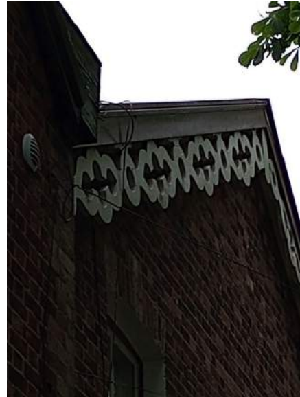
Neighbour's barge boards
