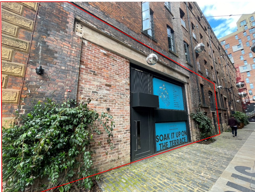
Figure 9a: The main entrance into the unit from Little David Street, showing the modern doors, windows and area of modern brickwork to the immediate left.
