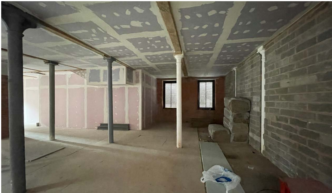
Figure 15: A view looking north-west across the northern end of the unit at upper ground floor level, showing the modern blockwork wall dividing this unit from the adjacent unit (right).
