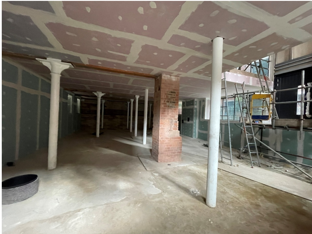
Figure 12: Another view looking north, showing the original, and modern columns supporting the upper ground floor level.
