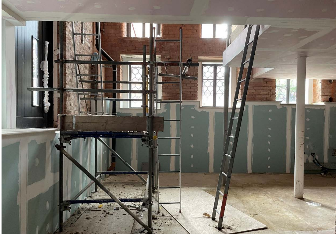
Figure 10: Current view looking south along the lower ground floor level of the Unit towards the Chorlton Street elevation, showing the modern plasterboard lining to walls, floor and ceiling.
