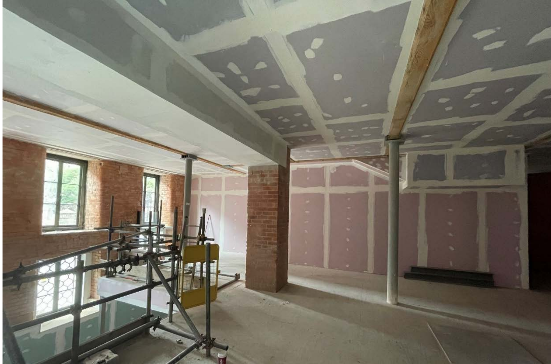
Figure 14: Looking north-west across the width of the ground floor level, showing the modern plasterboard walls and ceilings. The central brick pillar and metal columns are all modern, whilst the brickwork to the left is original.
