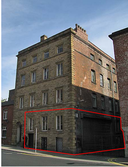
Figure 6: The south elevation on Chorlton Street, showing the c1930s roller shuttered entrance into the current unit to the right in 2017. The demise of The Site outlined red.
