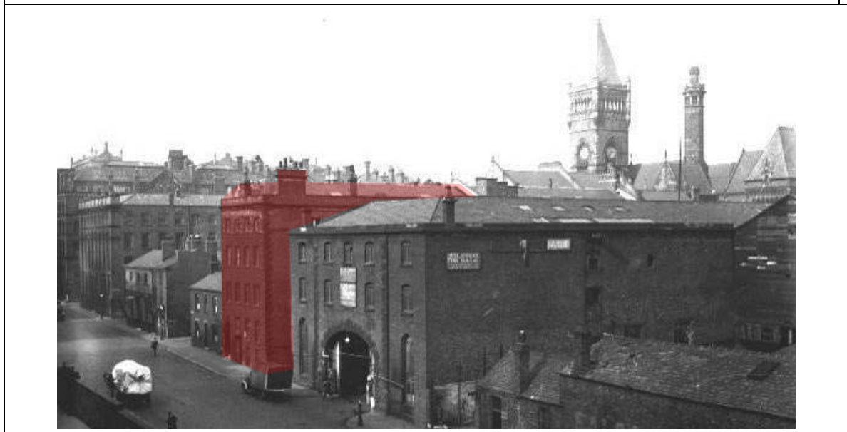
Figure 5: 1944 – Looking north across Chorlton Street towards the Minto and Turner Building (shaded red).
