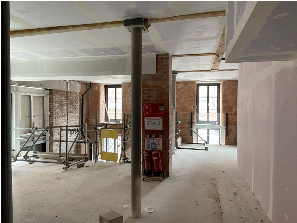
02 view of unit existing interior
