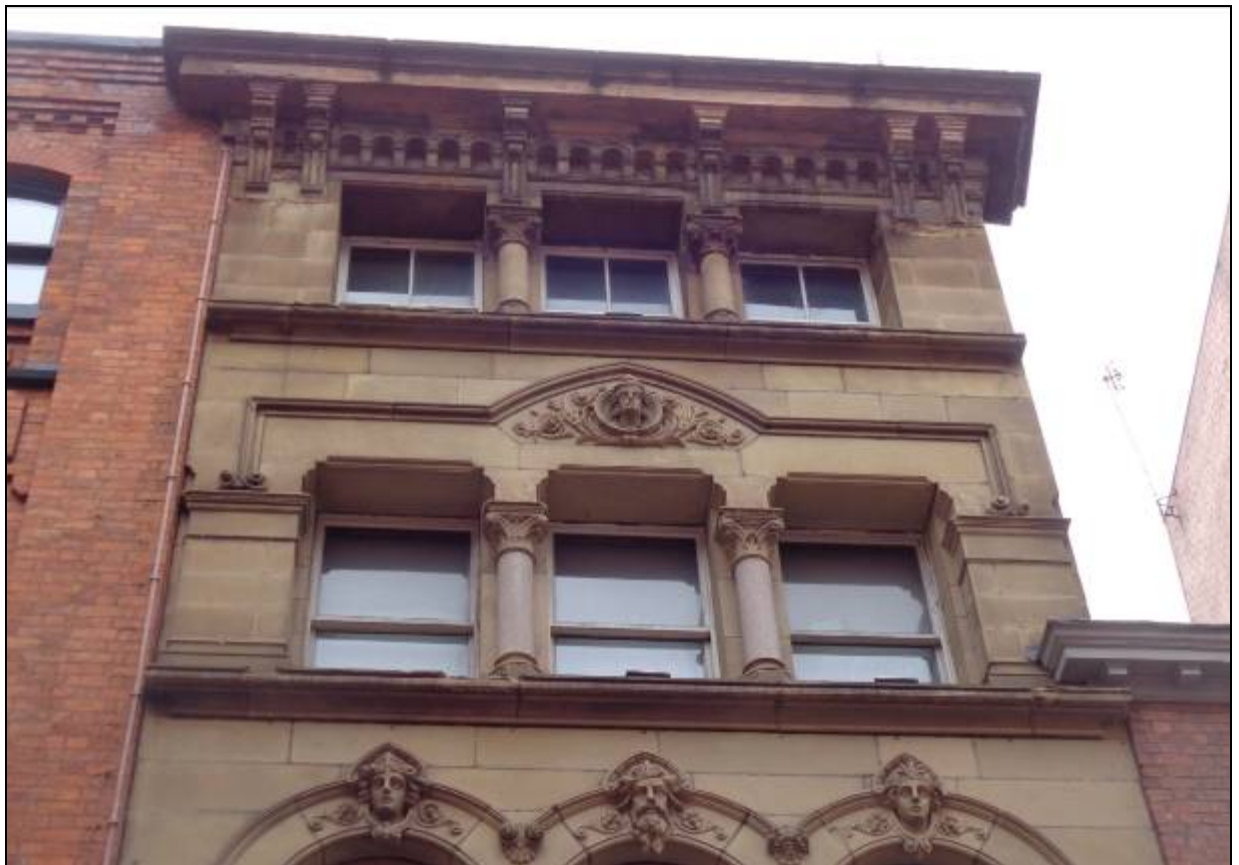
6. Timber windows on the second and third floors
