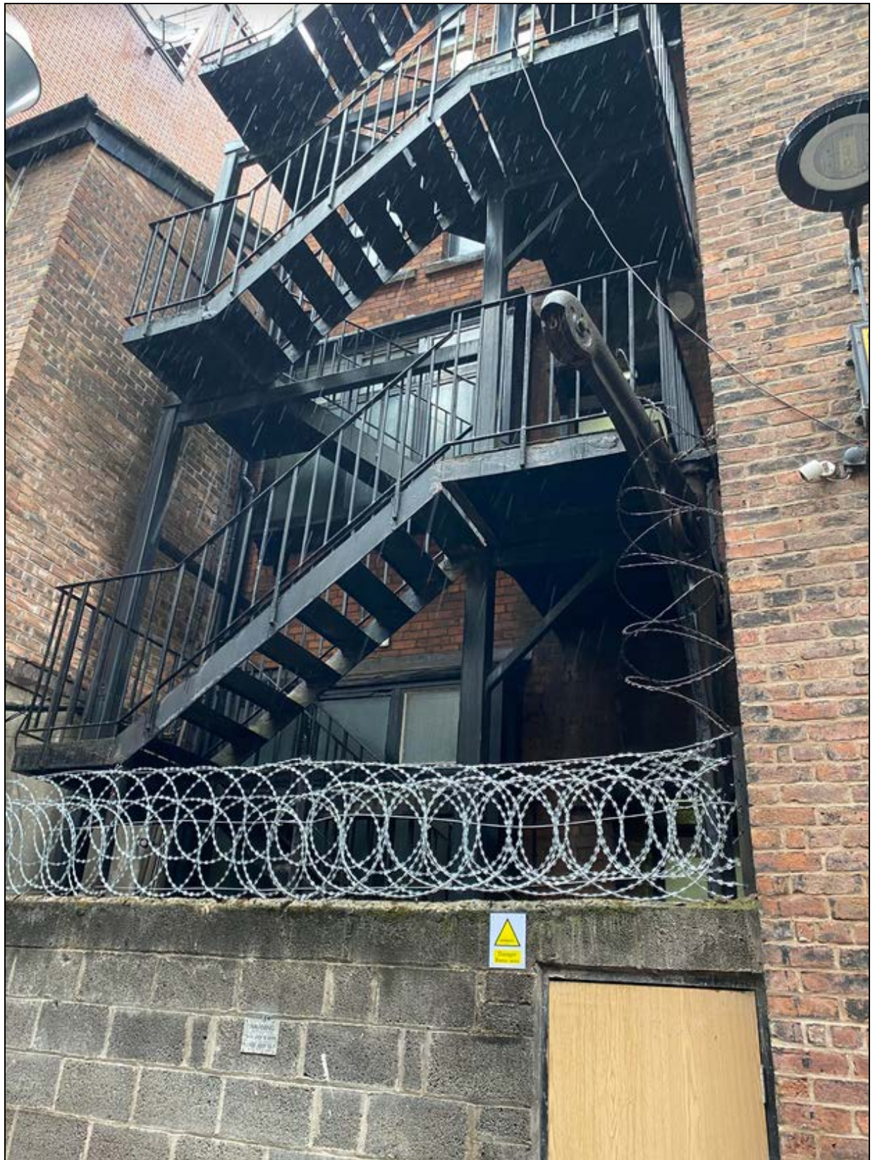
7. Rear elevation, showing blockwork wall and fire escape
