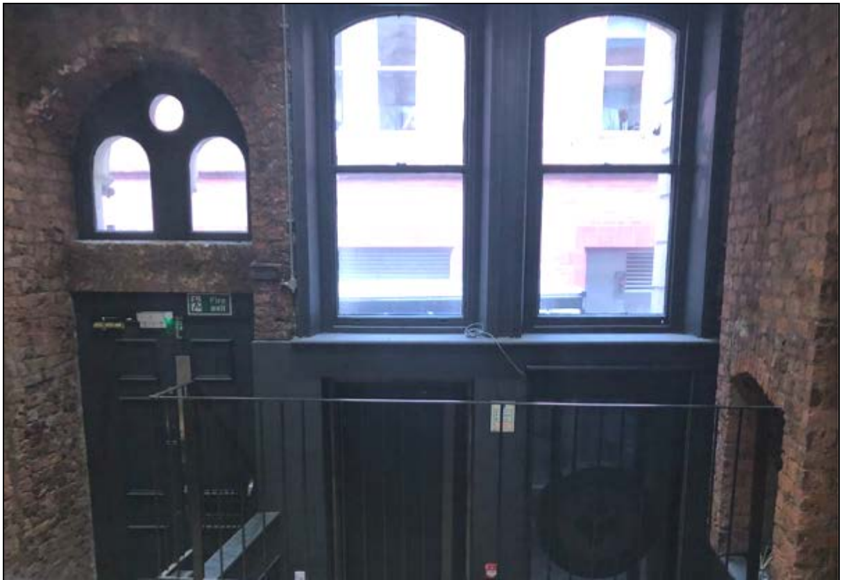
8. Upper ground floor, looking to front
