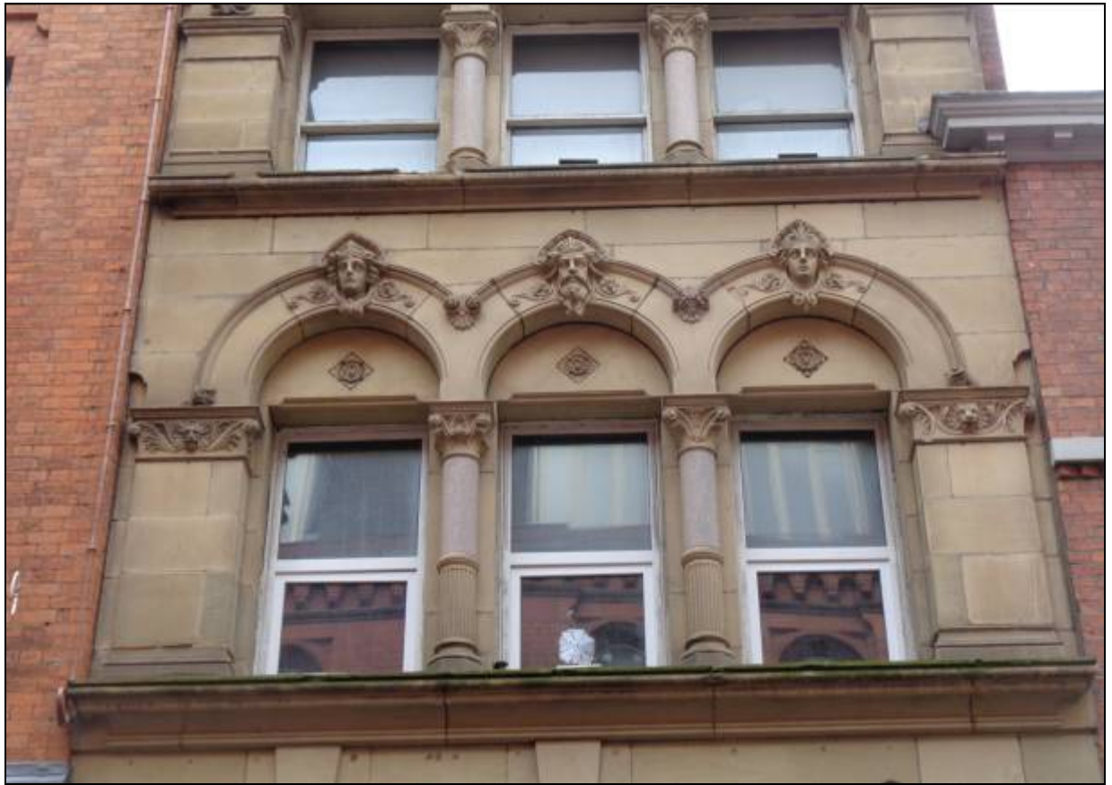
5. UPVC windows on the first floor
