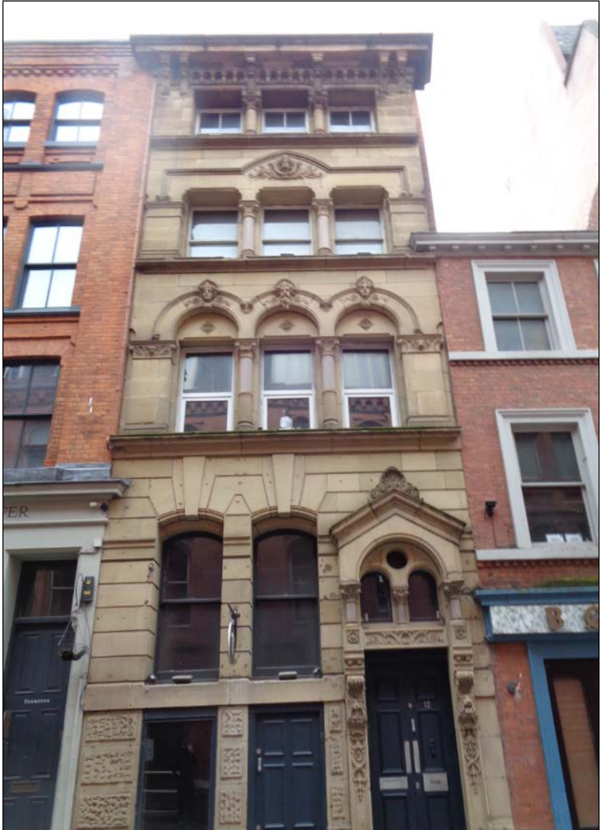
1. The listed building, built as offices in 1876
