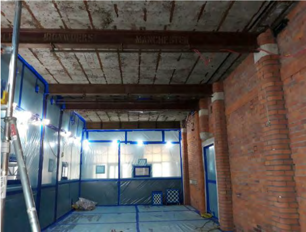
Figure 2.0 – Historical photograph of floor plate (taken 2019)
