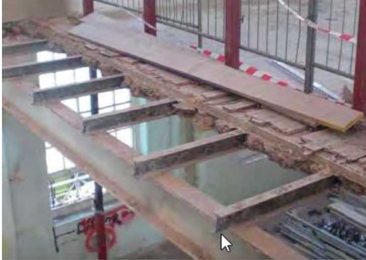
Figure 2.2 – Typical Construction of Filler Joist Floors
