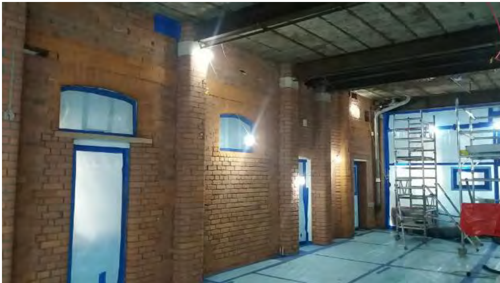
Figure 2.1 – Historical photograph of floor plate (taken 2019)
