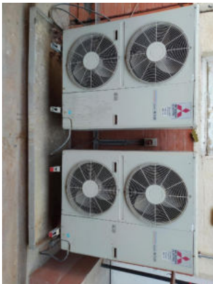
EXISTING 2x CONDENSEN UNITS TO BE STRIPPED OUT ALONG WITH ASSOCIATED PPEWORK
