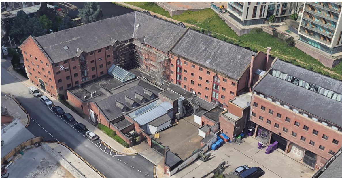
Figure 7) Aerial view from the east showing new block (right) and new single storey ancillary structures
