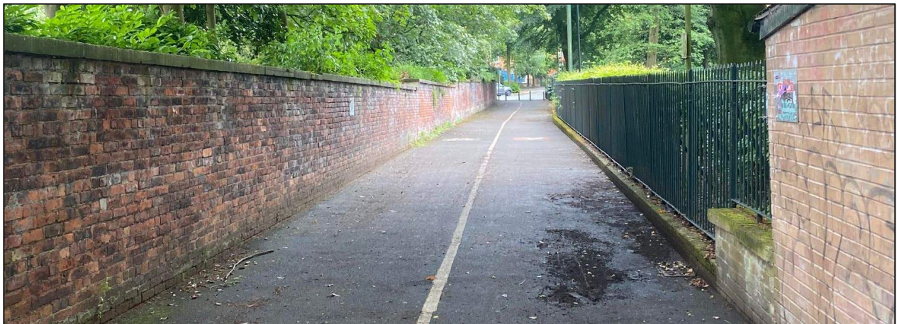
Figure 4-7 - Existing Brick Wall (Looking South on Whitworth Lane)
