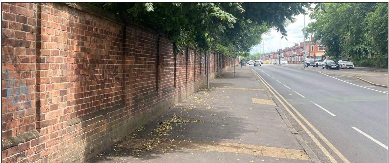
Figure 4-8 - Existing Brick Wall (Looking East on Moseley Road)
