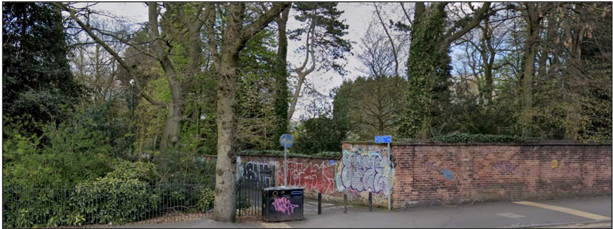
Figure 4-6 – Existing Brick Wall (At Intersection of Whitworth Lane and Moseley Road) – Google Street View
