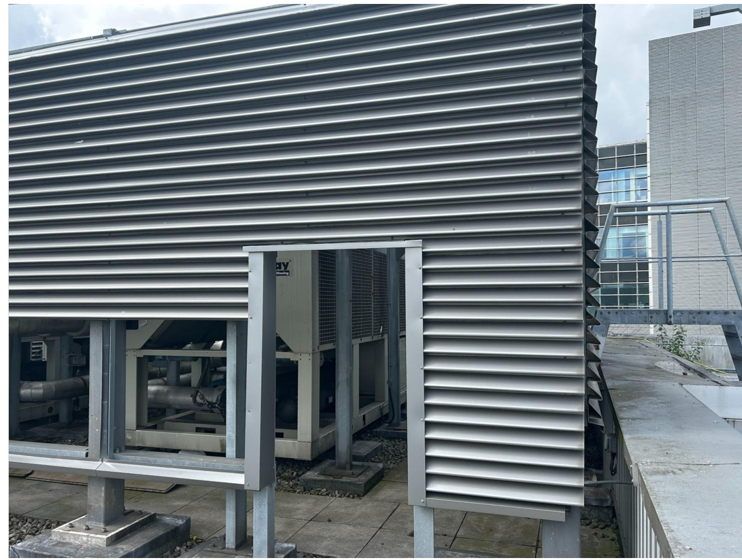
Area 3 Existing Louvres to be removed By Others
