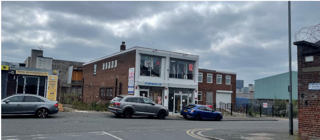
Figure 5 – Existing business in the northern part of the building
