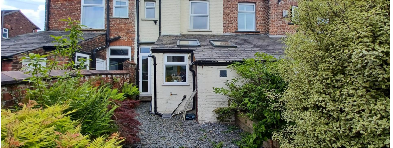
Figure 2. Rear view of property.
