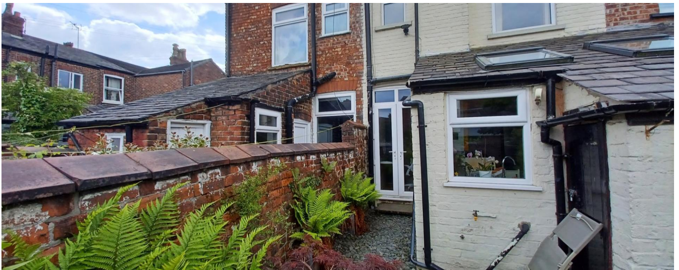
Figure 3. View of shared boundary with adjoining terrace.
