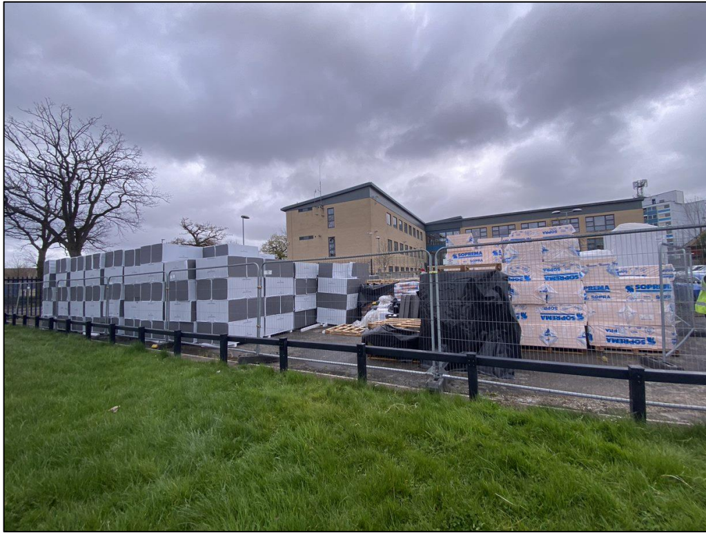
Plate 5 – Character of the hardstanding section of the application site
