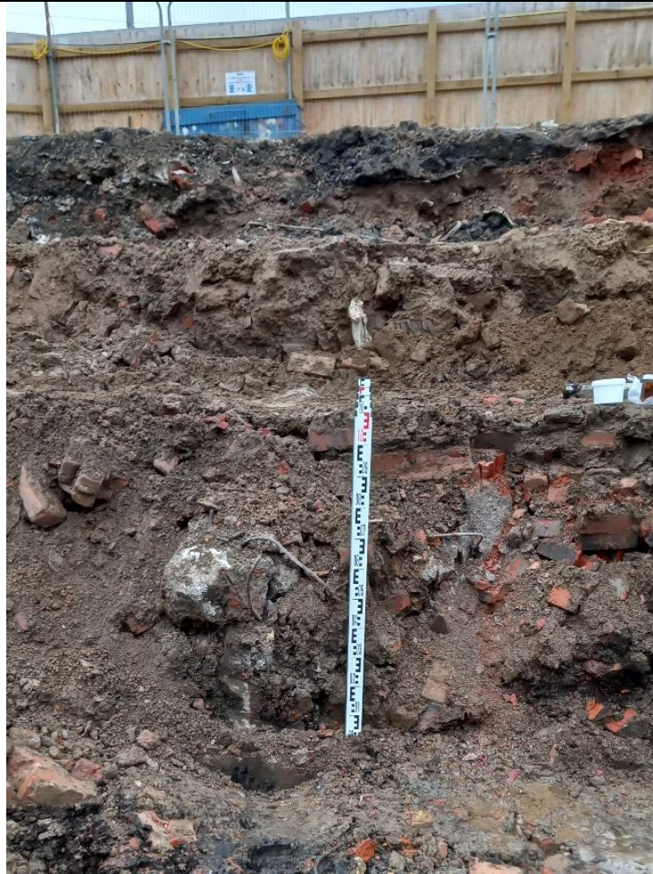
Photo 47: Ground condition along the southern basement wall – sample LR03. Photograph taken facing the south on 09/11/2021.
