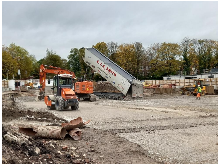
Photo 44: Imported materials used in the backfill of the excavations. Photograph taken of the upper raft, facing the north and north-west on 09/11/2021.
