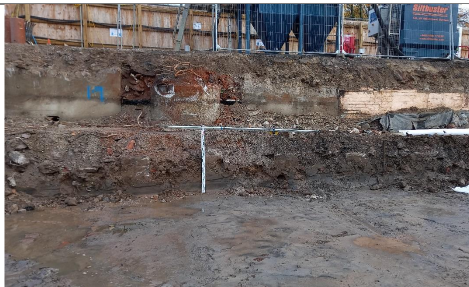
Photo 51: View of the excavation towards the eastern basement boundary. Photograph taken facing the north-east on 10/11/2021.
