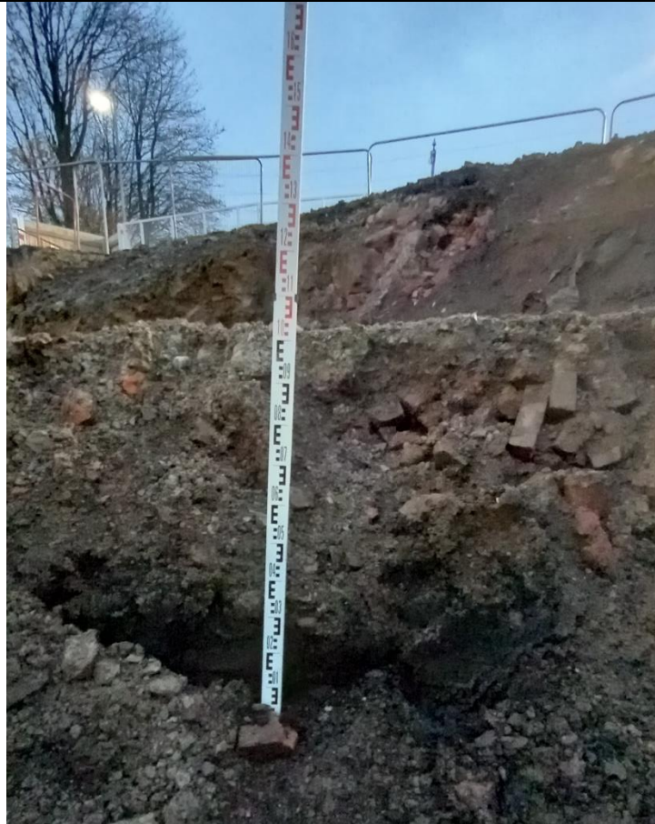
Photo 49: Ground conditions along the south of the basement wall. Sample LR04 retrieved from here. Photograph taken on 09/11/2021.
