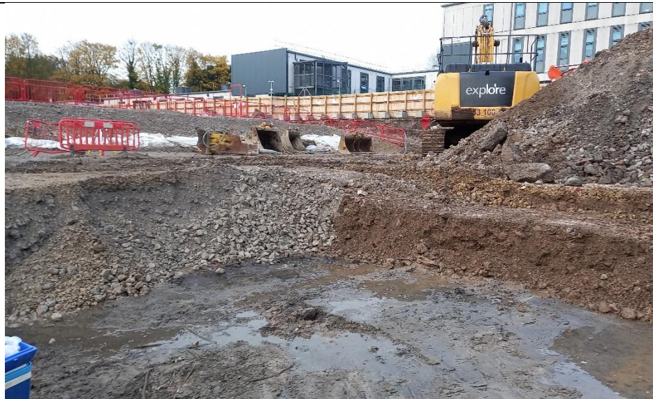
Photo 50: The excavated area where the contamination was previously encountered, south of the basement area. Stockpiled material to the right of the photograph. Samples LR05 and LR06 retrieved from base of the excavation. Photograph taken facing the north on 10/11/2021.
