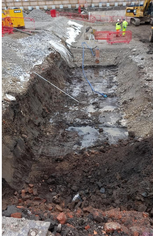
Photo 43: Ground conditions beneath the broken out concrete in the south-western basement area. Photograph taken facing the north-east on 09/11/2021.
