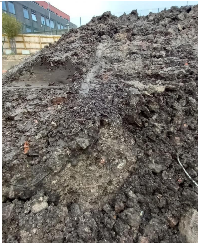
Photo 56: View of the excavated material from the southern-eastern basement area. Photograph taken on 10/11/2021.
