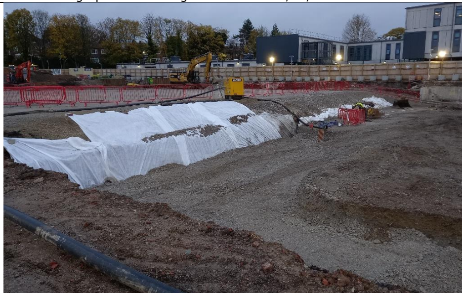
Photo 48: View of the backfill in the south-western area of the basement. Photograph taken facing the north on 09/11/2021.
