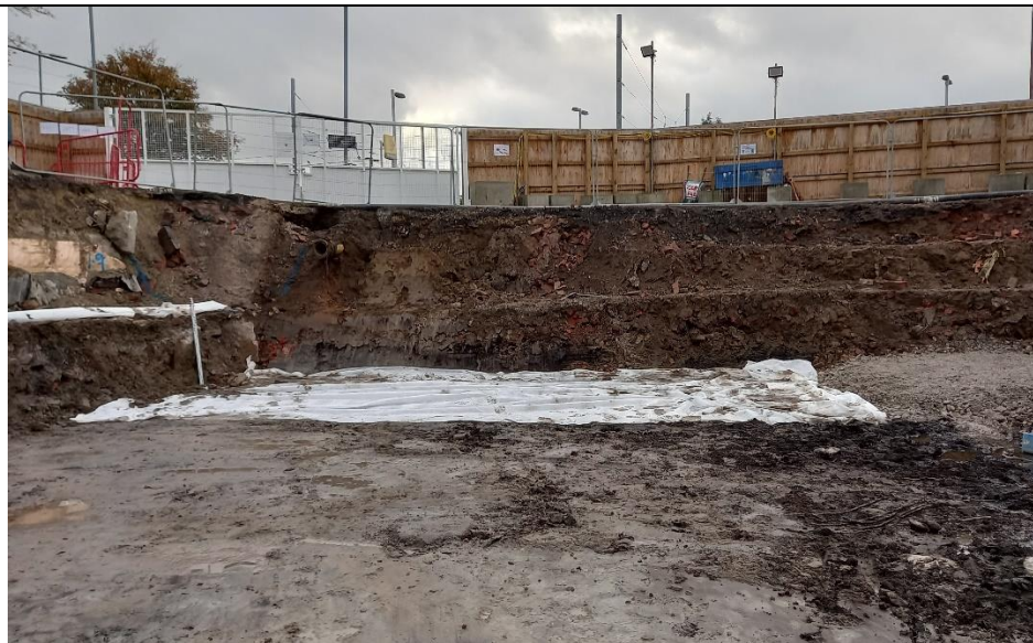
Photo 53: View of the excavation towards in the south-eastern corner of the basement boundary. Photograph taken facing the south on 10/11/2021.
