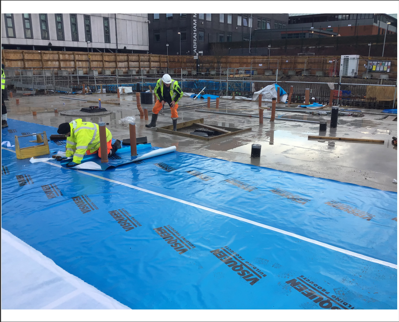
Overview photograph of the area verified during installation
