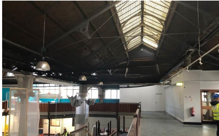
Figure 68: Looking east along the southern mezzanine.
