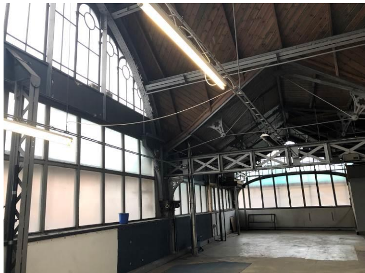
Figure 72: Looking north along the western mezzanine.
