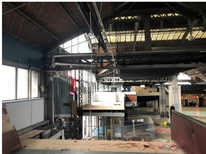
Figure 67: Looking west along the southern mezzanine
