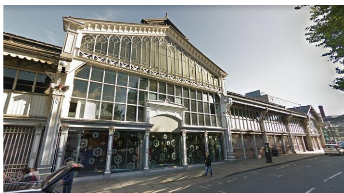
Figure 38: The central, raised portion of the southern elevation, showing original cast iron Venetian windows to gable and modern glazed openings to lower portions in the place of removed original cast iron railings. (2018)
