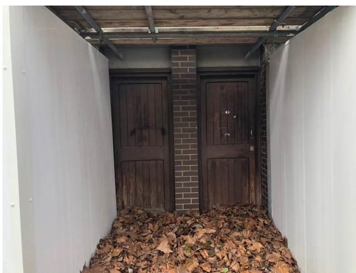
Figure 47: Examples of 1980-3 doors to the east elevation.
