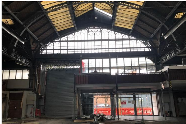
Figure 49: The central section of the south elevation.
