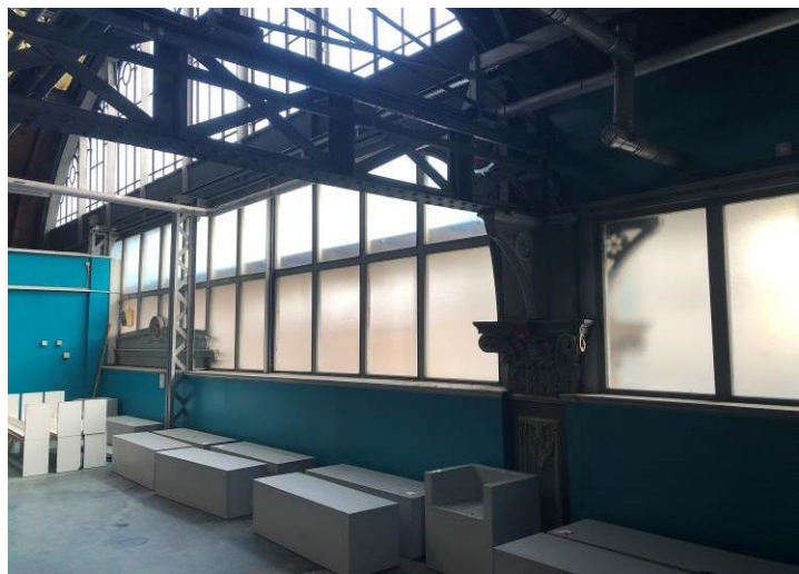
Figure 69: The eastern side of the southern mezzanine.
