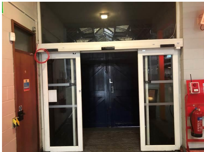
Figure 57: The modern entrance vestibule to the west elevation.
