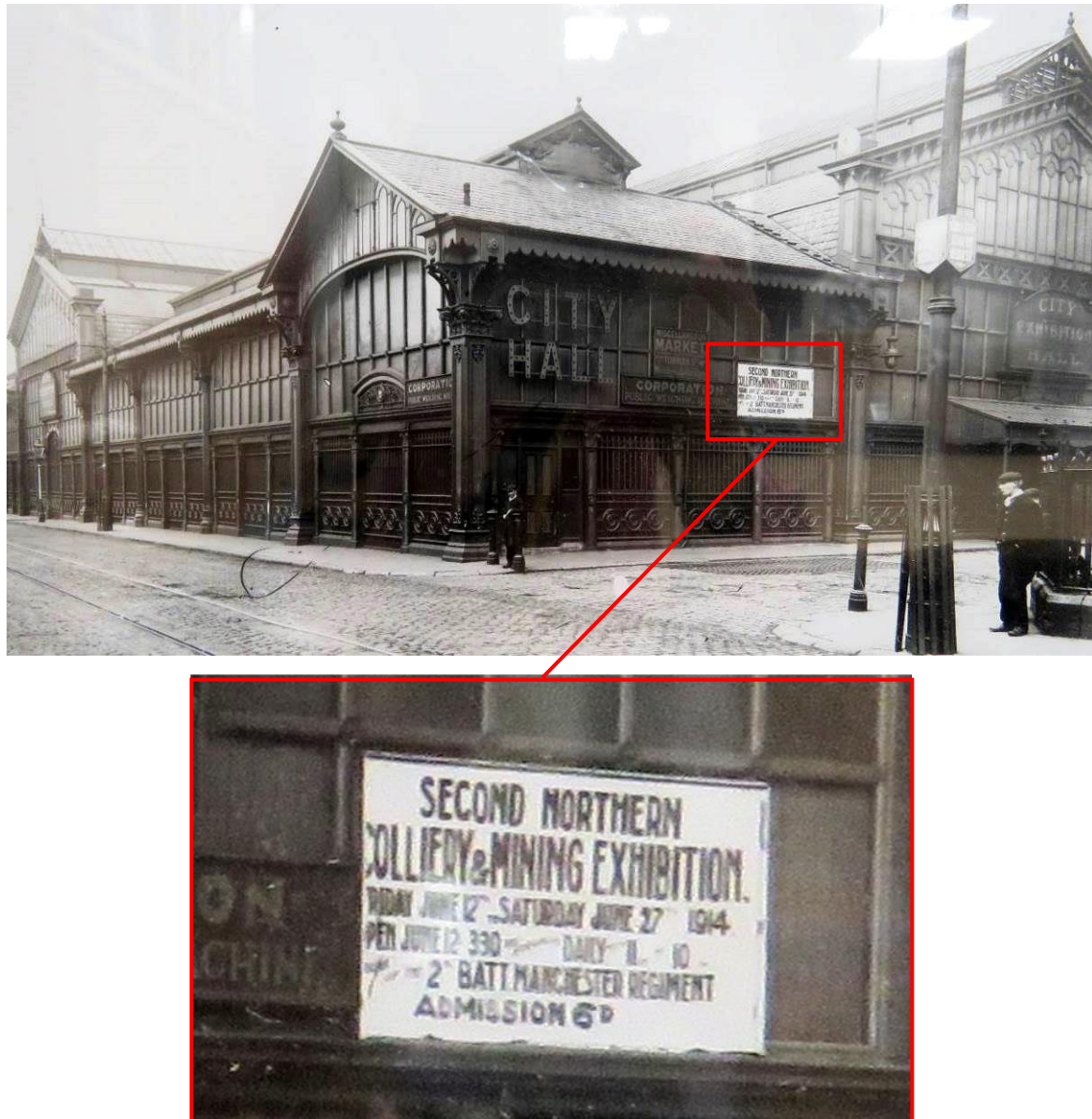
Figure 24: The Liverpool Road (left) and Byrom Street (right) elevations of the City Exhibition Hall (formally the Lower Campfield Market) in 1914. The sign on the east elevation of the hall advertises the second northern colliery and mining exhibition. (Source: Manchester Archives)
