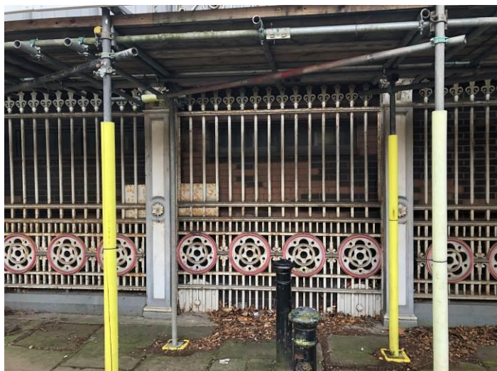
Figure 40-41: Examples of the original sliding gates to the north elevation. Note the wheels (bottom) and lock protection plates (centre).
