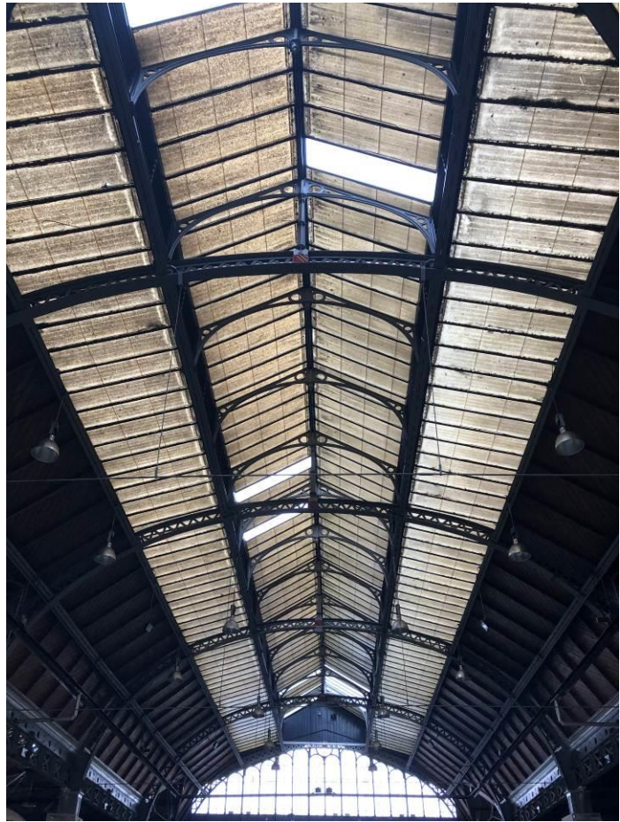
Figure 66: Looking west along the length of the roof structure.
