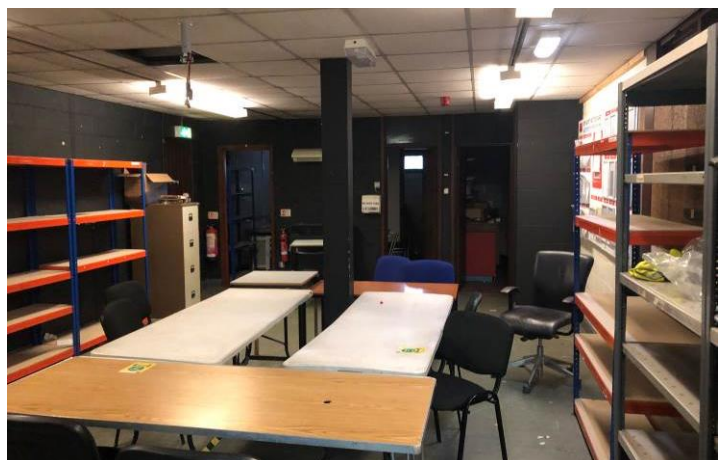
Figure 61: The modern 1980s rooms to the south-east corner of the ground floor.
