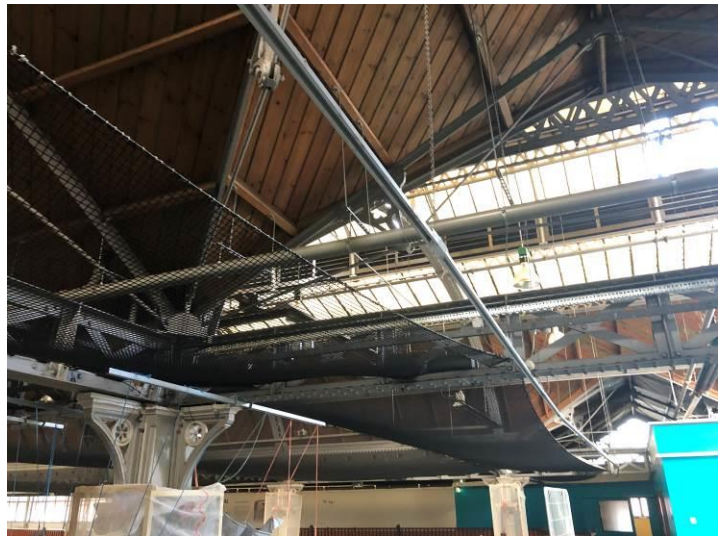
Figure 63: Central section of the eastern side of the roof structure, showing the 1980s timber boarding replacements.
