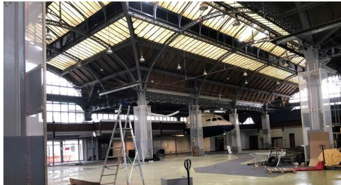
Figure 48: Looking south-west across the building towards the southern elevation.
