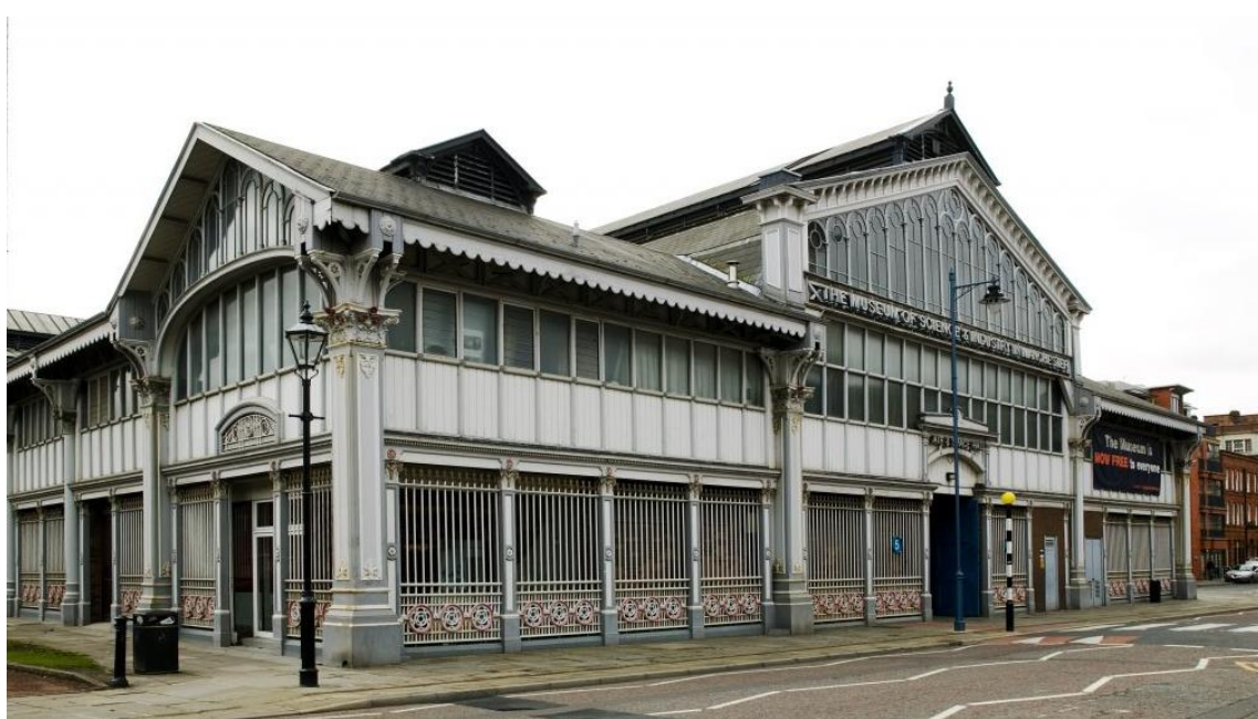
Figure 1: The western elevation of the building as it appears today.
