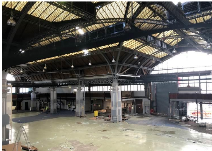
Figure 50: Looking south-east across the building towards the southern elevation.
