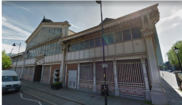
Figure 42: The southern elevation as seen from Lower Byrom Street. (2018)
