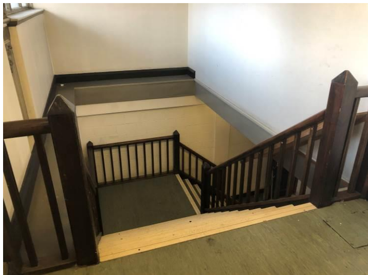
Figure 74: An example of one of the four 1980s mezzanine staircases located to each corner of the building.
