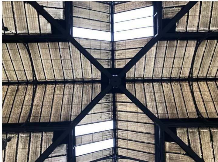
Figure 65: An example of the modern 1980s fibreglass panels (discoloured) and more recent clear coverings to the centre of the roof.
