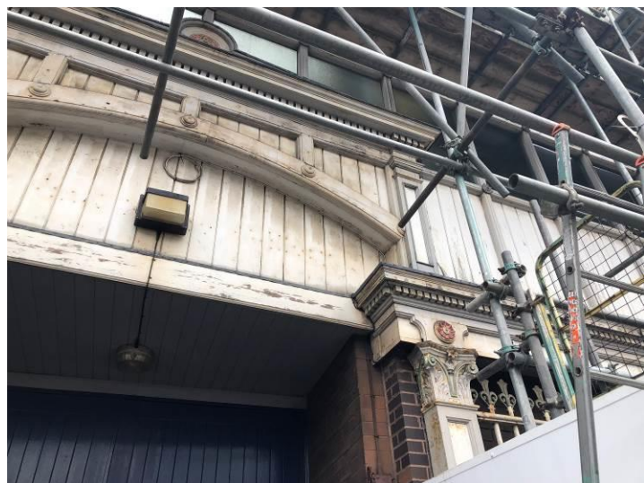
Figure 44: The lower parts of the west elevation.
