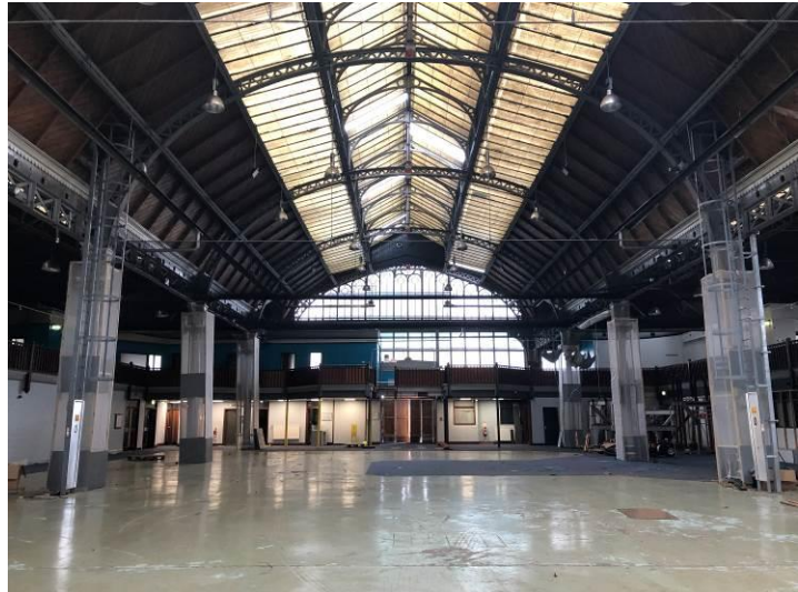
Figure 59: Looking east across the building towards the east elevation.
