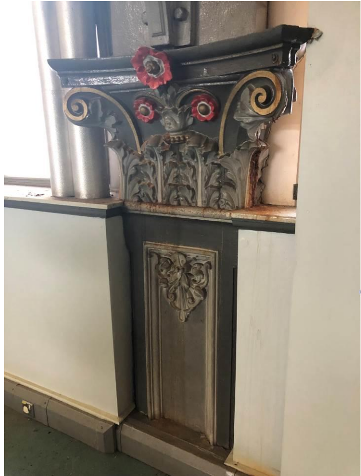
Figure 73: An example of one of the original decorative cast iron external columns, showing a representation of a Lancashire rose to the capital.
