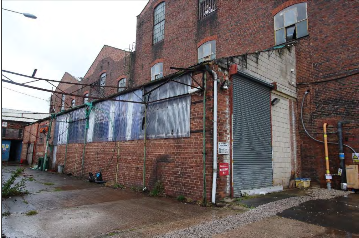
Plate 92: General view of Shed 3, facing north-west
