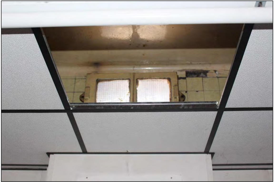
Plate 64: Detail of the obscured window within the northern wall of Room 6
