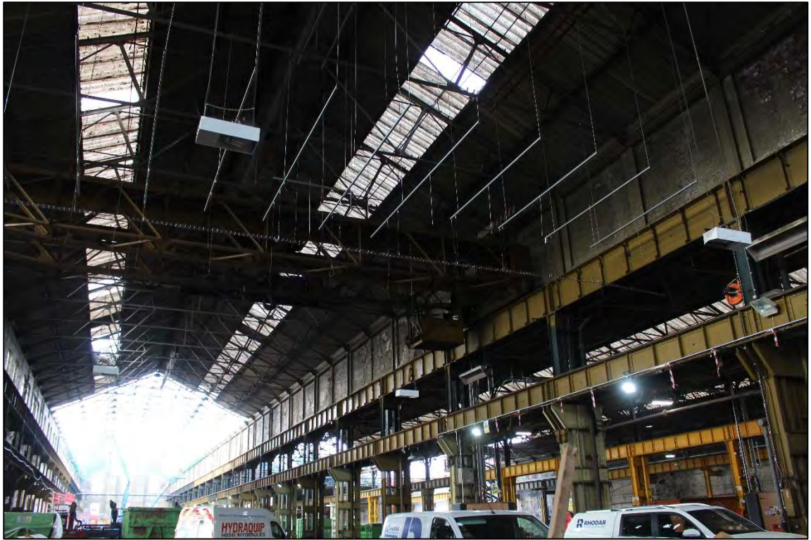
Plate 102: The retained traveling crane within the eastern bay
