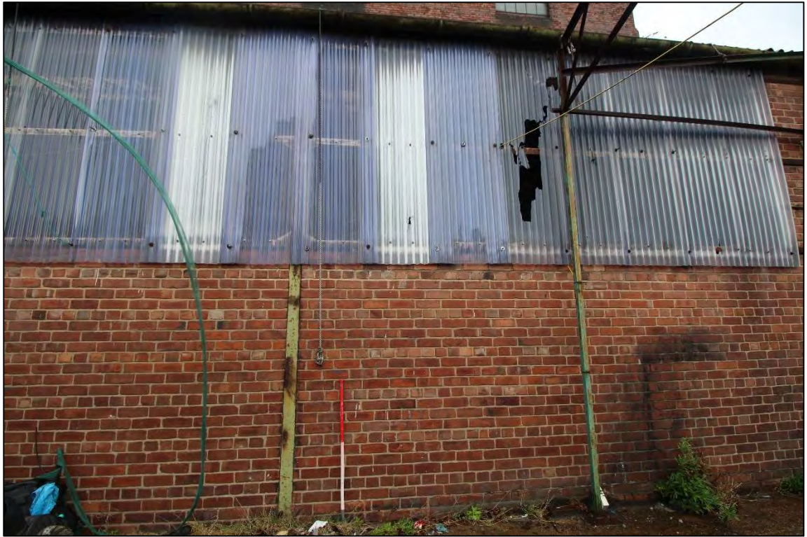
Plate 94: Detail of the modern inserted horizontal window within the southern elevation, looking north
