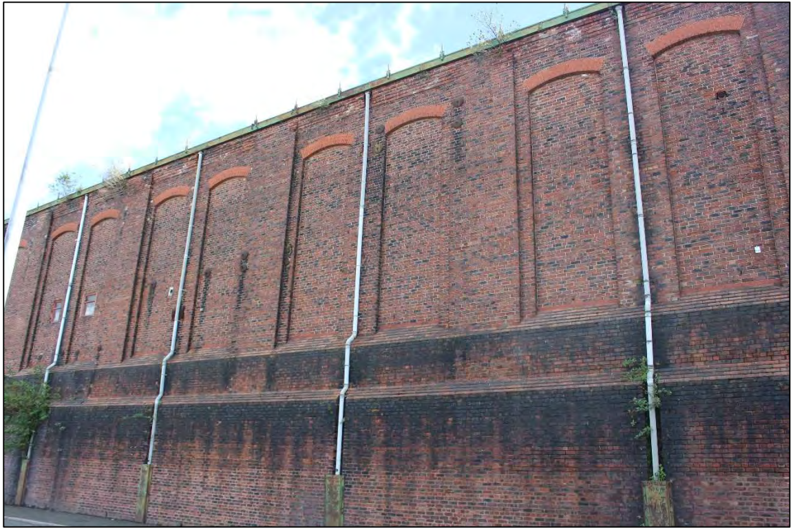
Plate 74: The western elevation of the boiler shop
