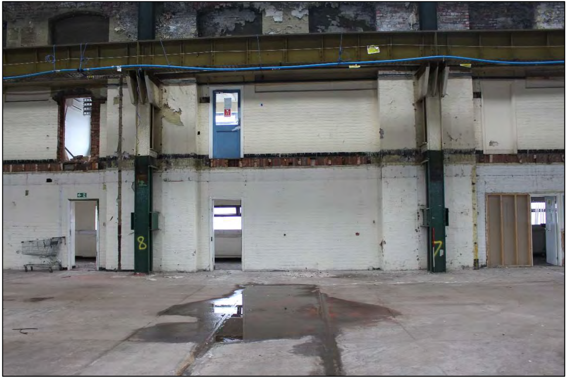
Plate 85: The infilled wagon doorway to the eastern wall of the eastern bay
