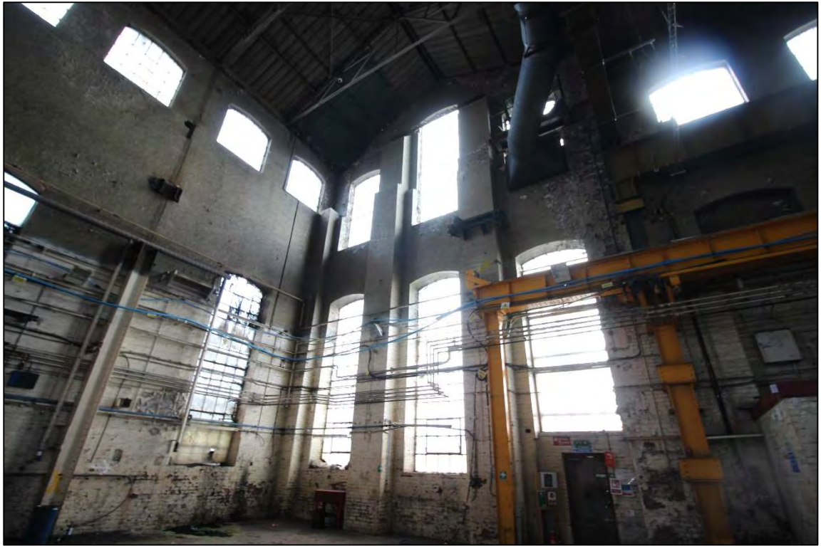
Plate 90: The eastern wall of the riveting bay
