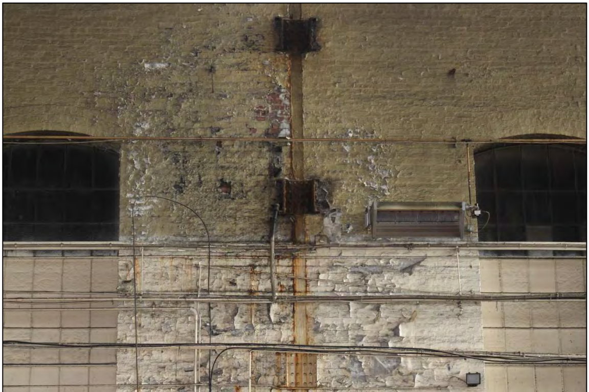
Plate 89: The remains of riveted steel beams within the northern wall of the riveting bay
