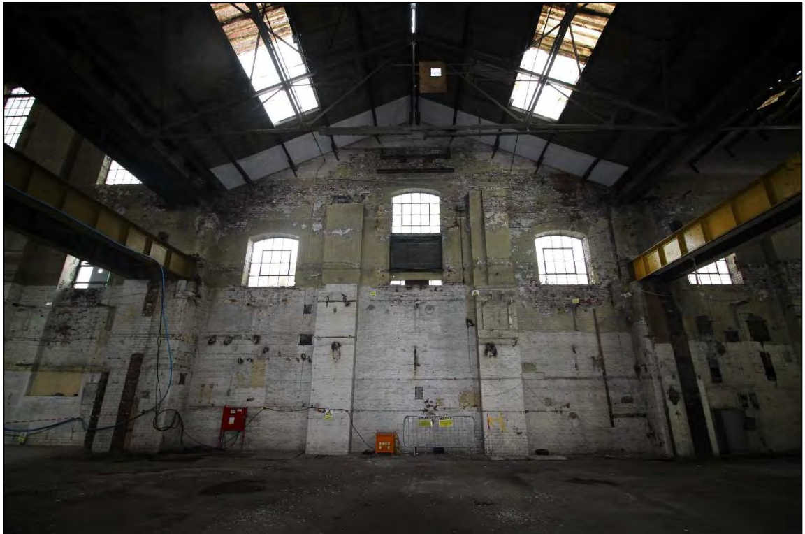
Plate 83: The southern wall of the central bay
