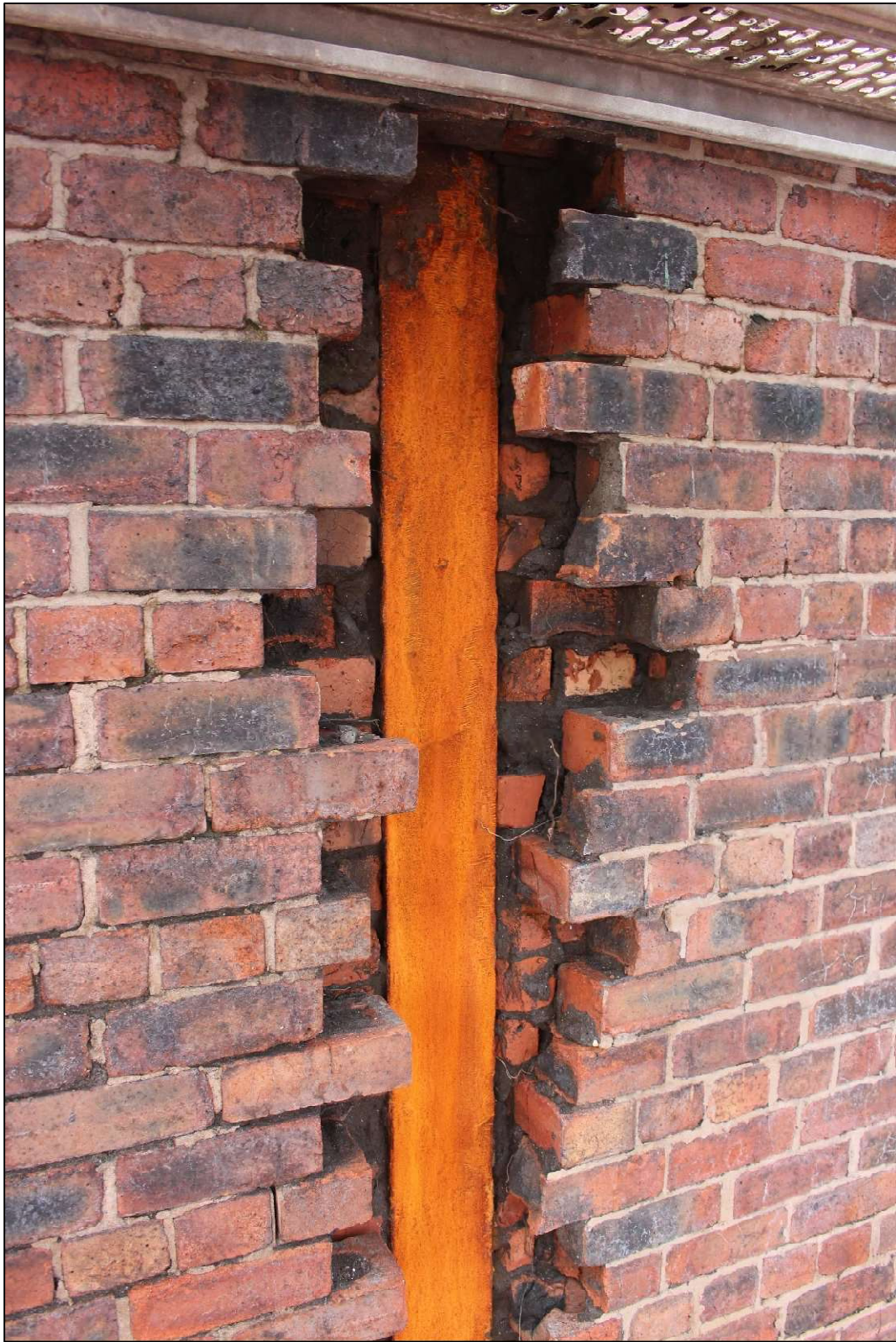
Plate 69: The steel I-section beam core within the piers to the eastern elevation
