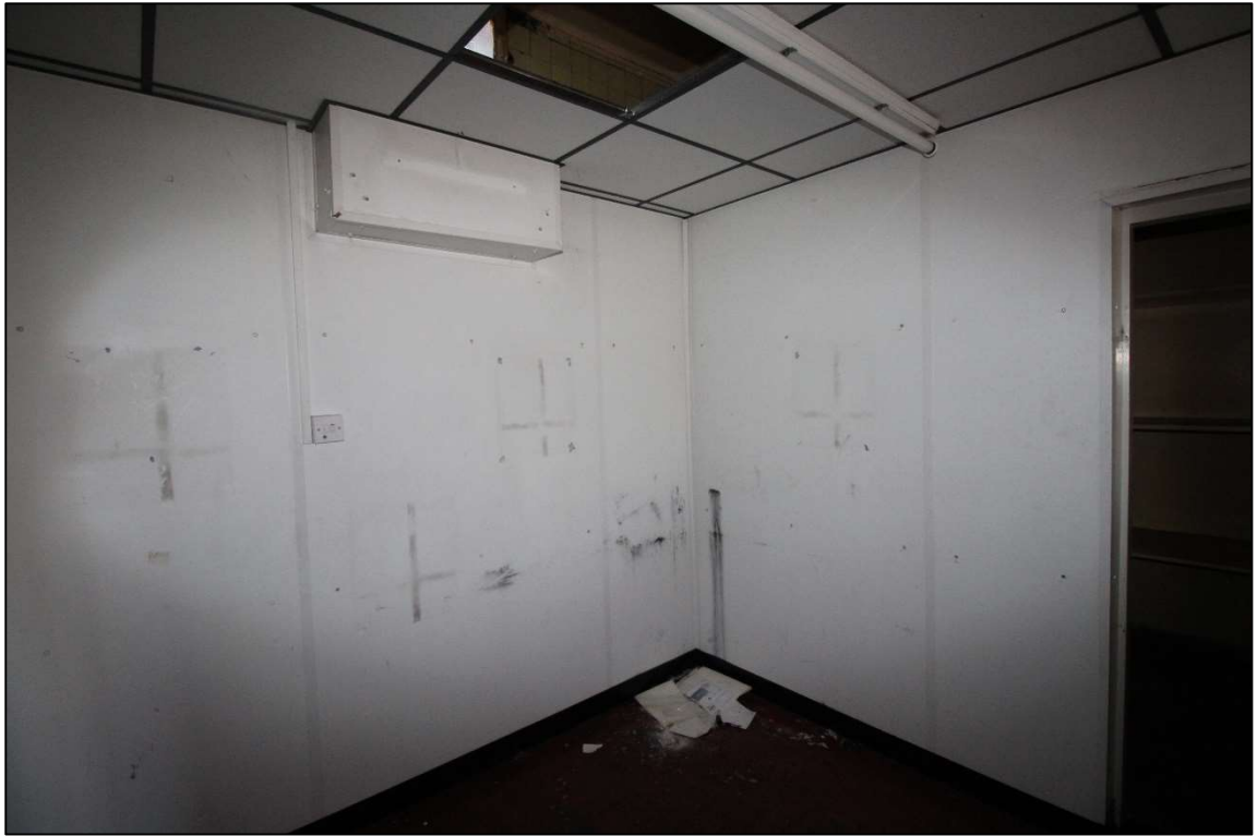
Plate 61: General view of Room 4
