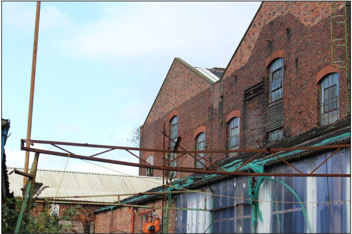
Plate 73: The southern gable wall of the central and western bays of the boiler shop
