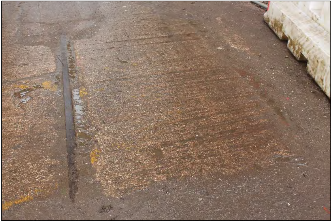
Plate 67: The retained rail tracks within the opening of the northern doorway
