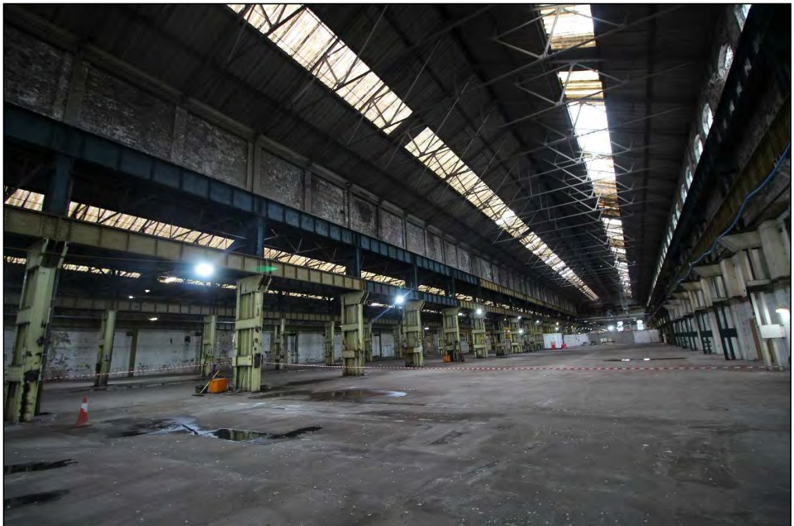
Plate 79: Internal view of the boiler shop, looking north-west
