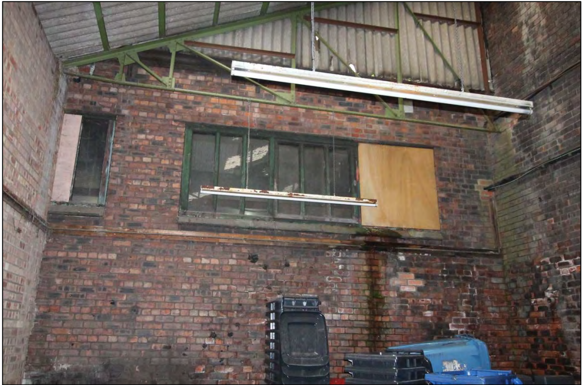
Plate 100: The eastern elevation of the substation that formed the western wall of the lean-to
