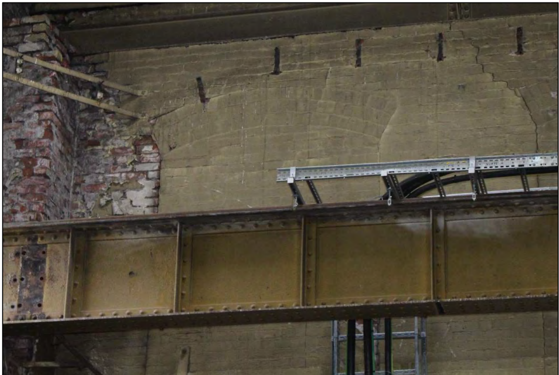
Plate 86: The infilled recesses within the western wall of the western bay
