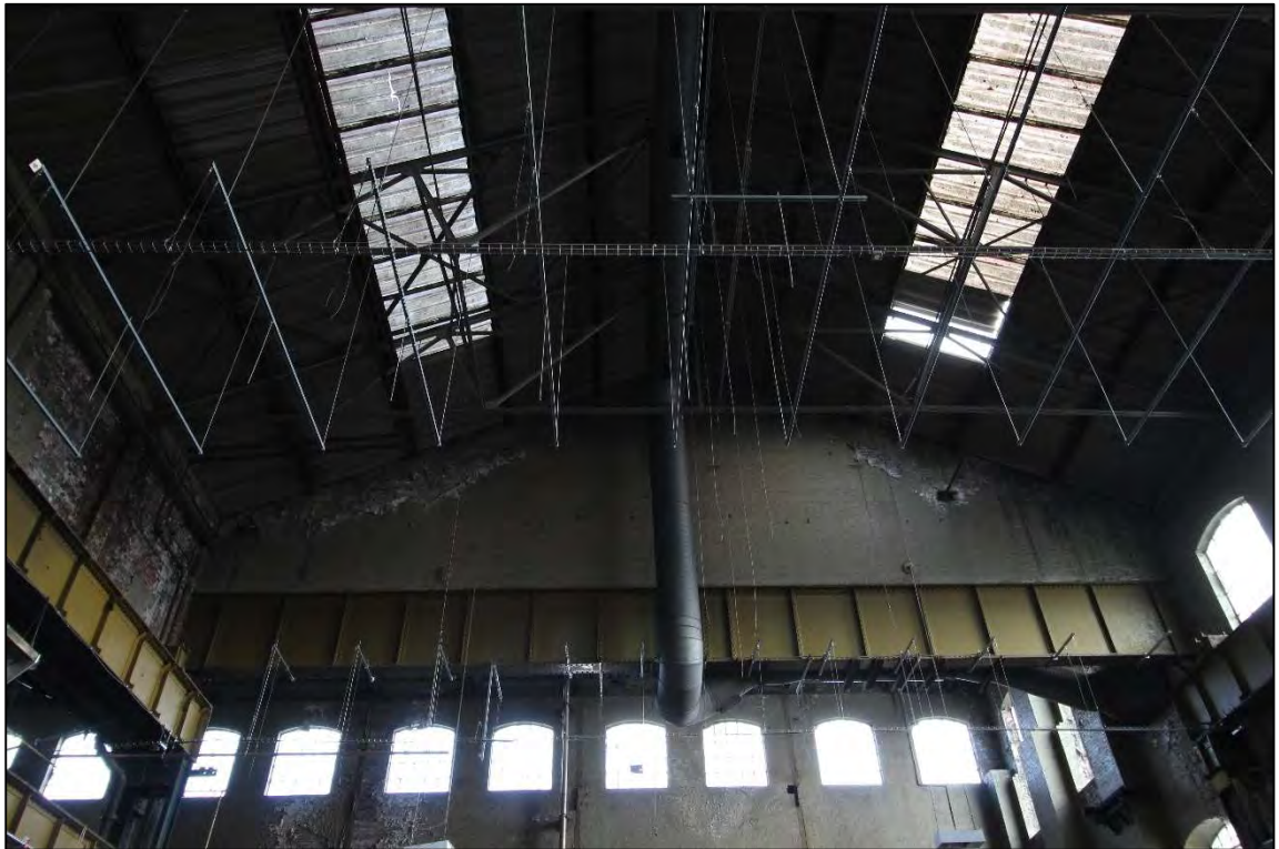
Plate 84: The northern wall of the eastern bay
