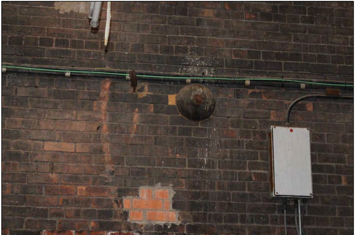
Plate 99: Detail of the tie rod plates within the northern wall of the shed
