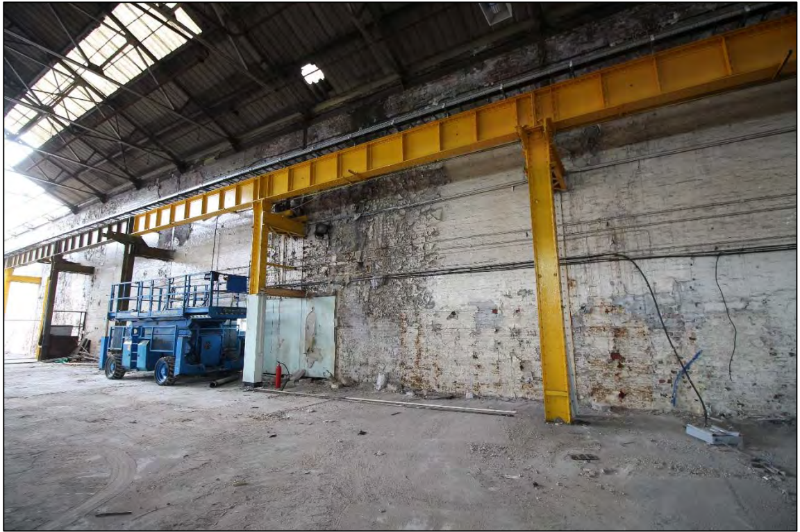
Plate 81: The western riveted steel beam and supporting stanchions to the western bay
