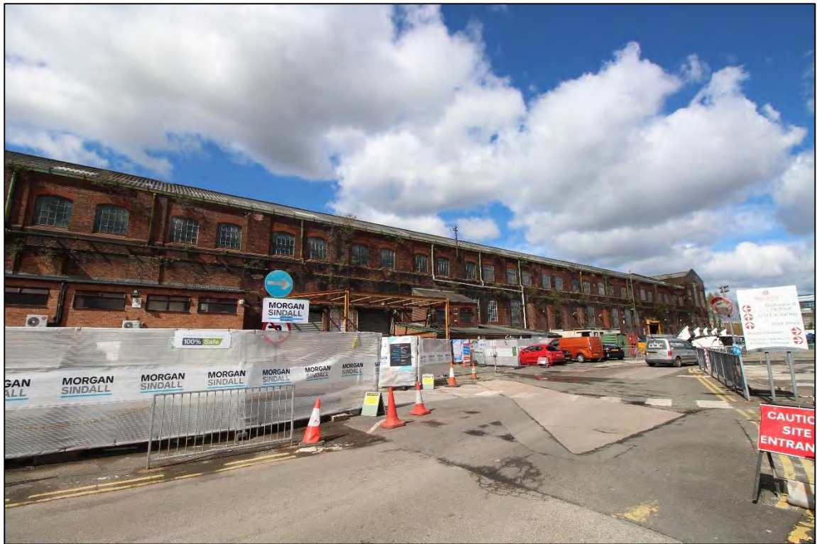
Plate 65: General view of eastern elevation of the boiler shop, facing north-west
