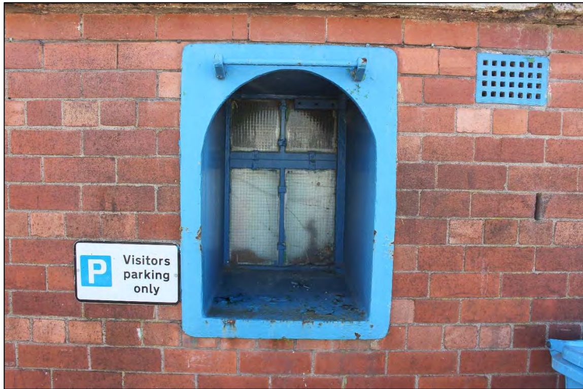
Plate 53: Detail of the cast-iron surround window to the northern elevation, looking south
