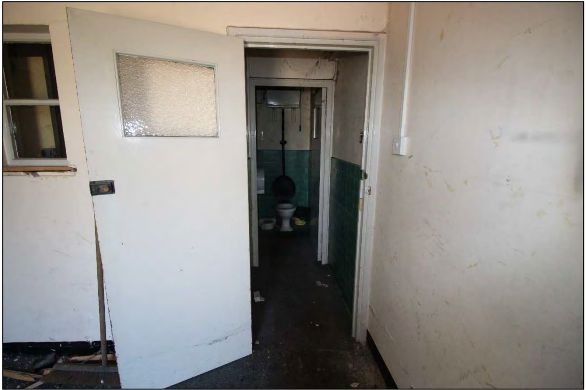
Plate 57: General view of Room 2, looking north
