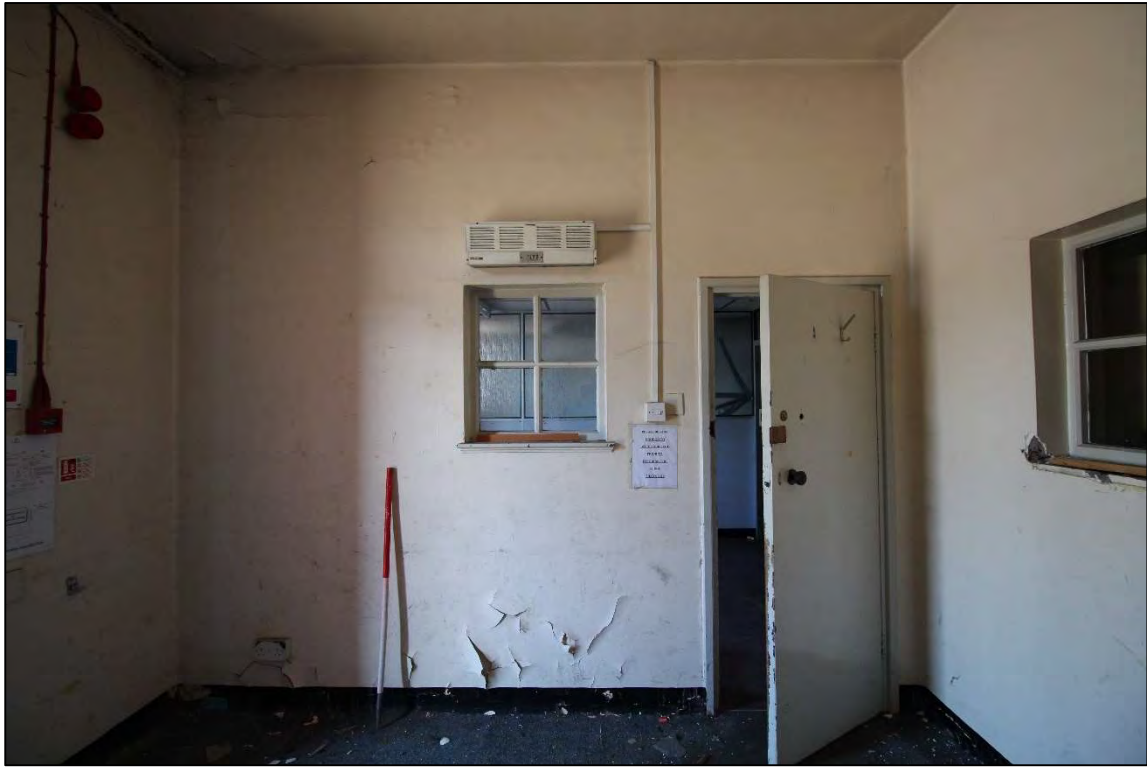
Plate 56: The western wall of Room 1, detailing the central window and doorway affording access to Room 3, looking west
