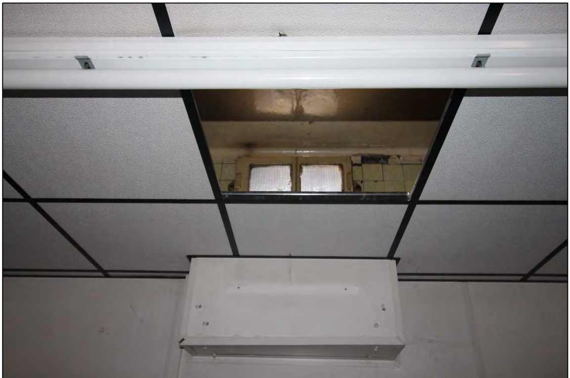
Plate 62: Detail of the obscured window within the northern wall of Room 4
