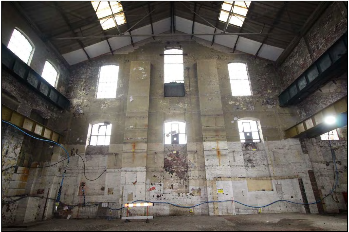
Plate 82: The southern wall of the eastern bay
