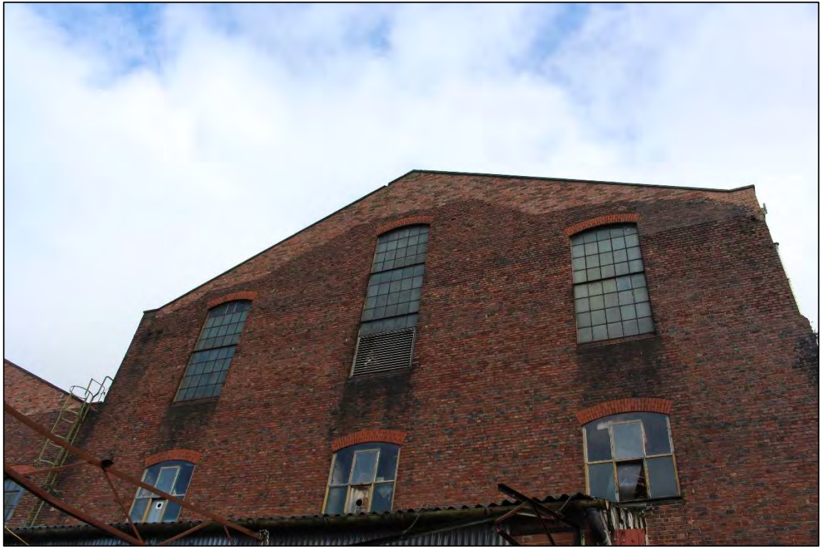
Plate 72: The southern gable wall of the eastern bay of the boiler shop
