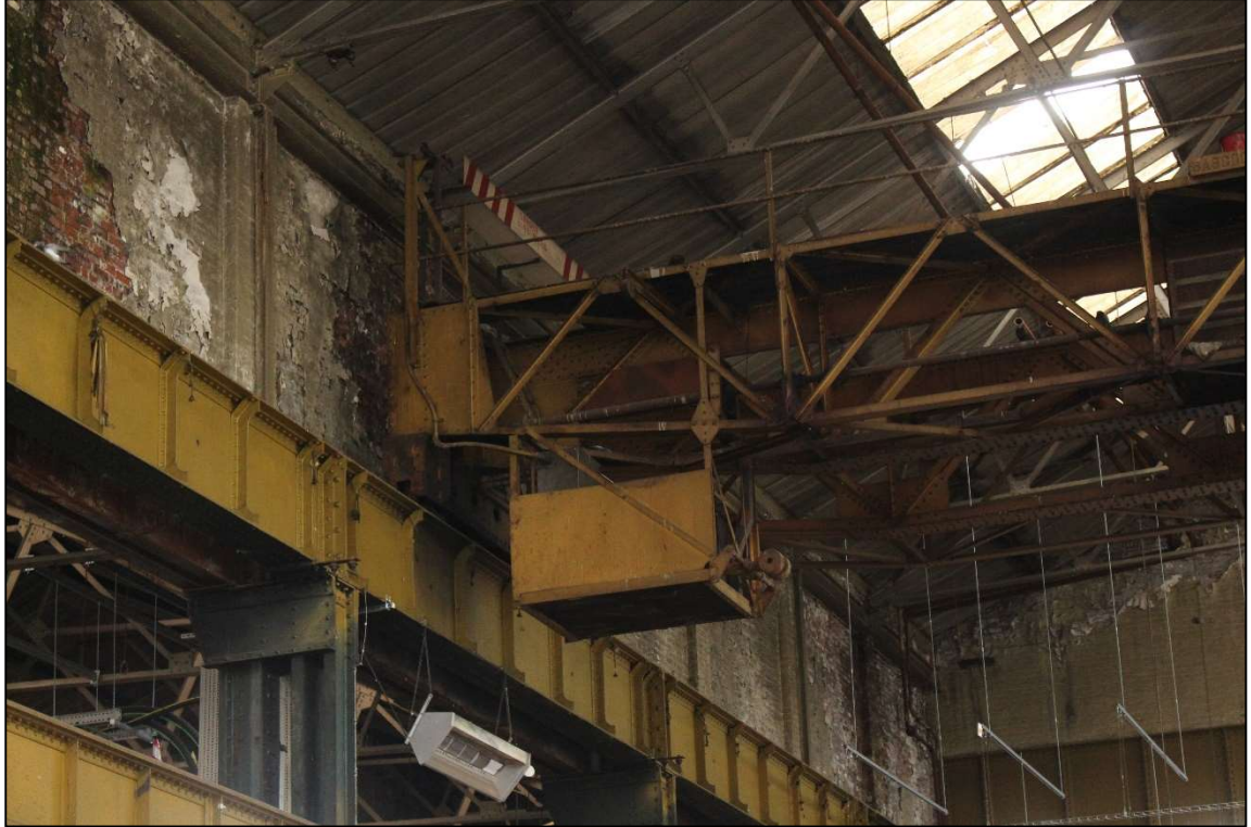
Plate 80: Detail of the retained travelling crane within the eastern bay of the boiler shop
