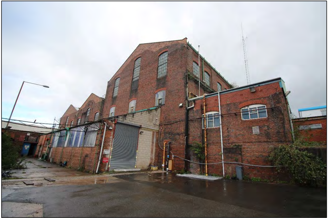
Plate 71: The southern elevation of the boiler shop, looking north-west
