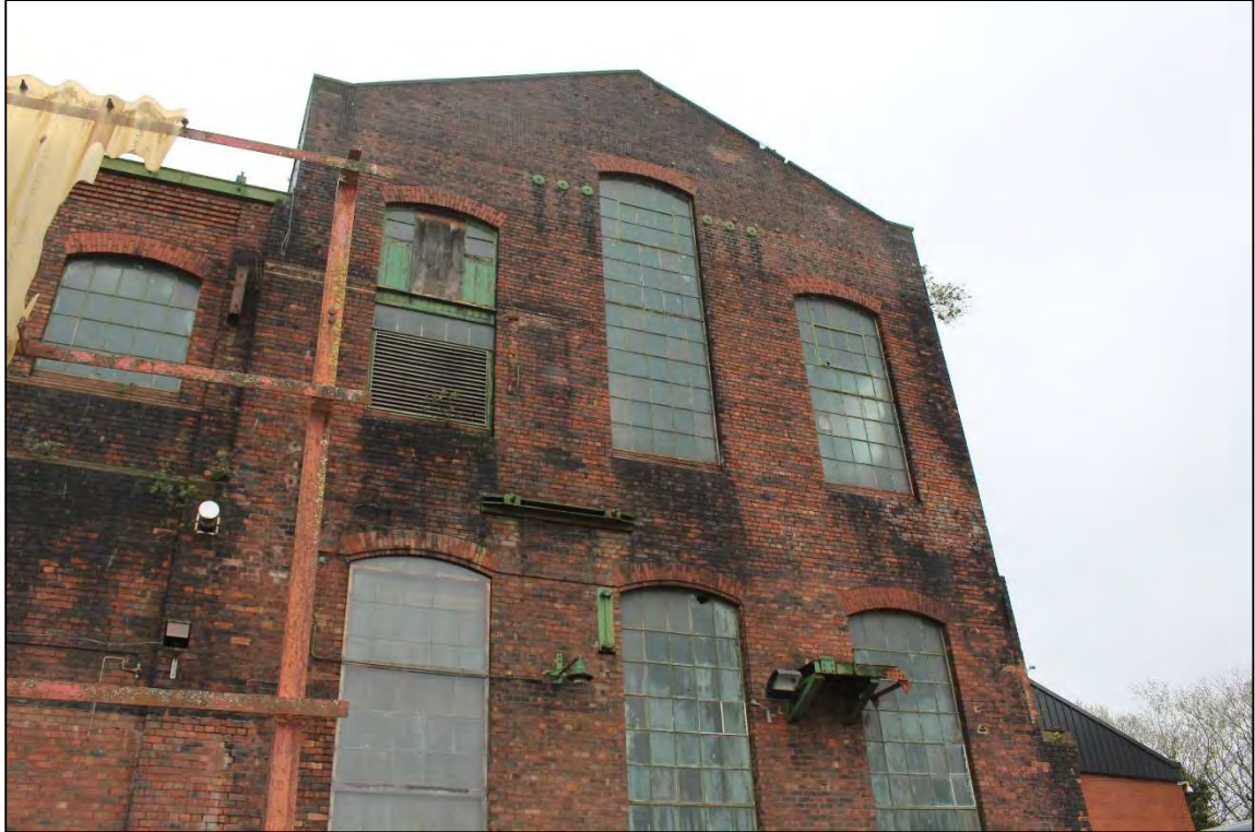
Plate 70: The eastern gable wall of the riveting bay at the northern end of the boiler shop
