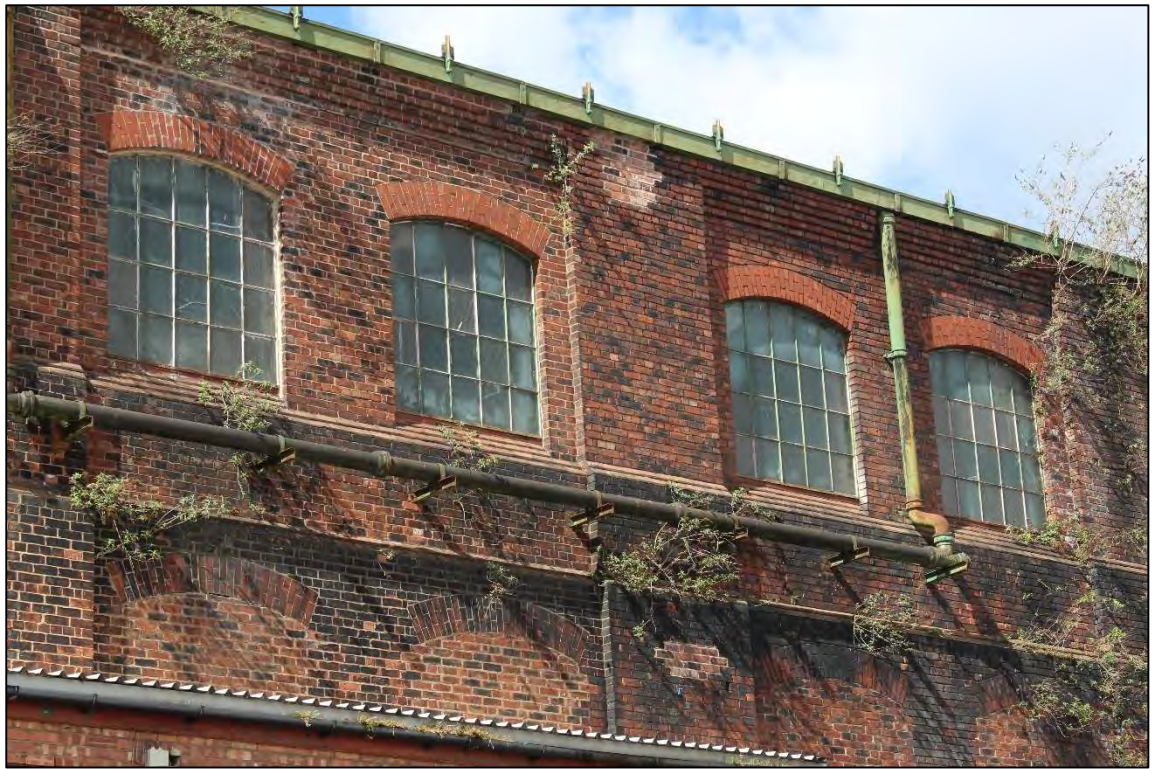
Plate 68: Detail to the upper windows on the eastern elevation of the boiler shop
