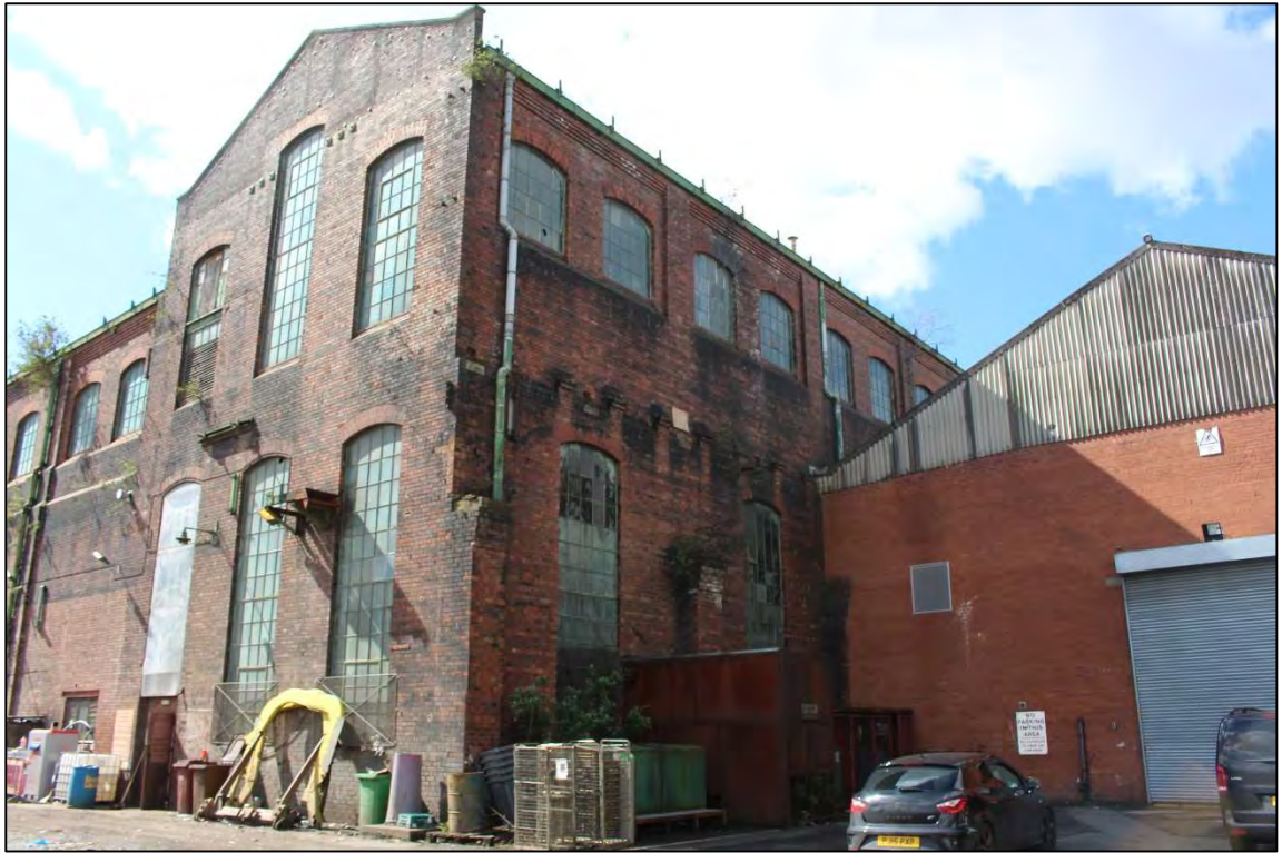
Plate 78: The northern elevation of the riveting bay, facing south-west
