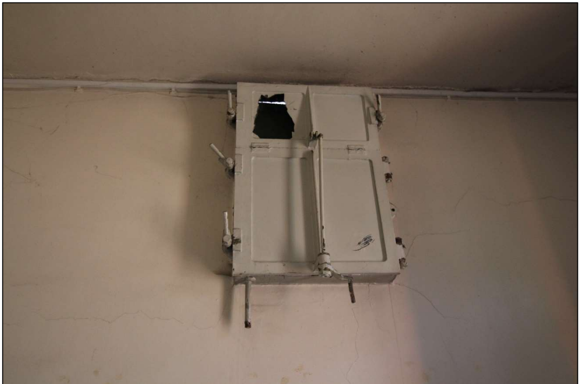
Plate 55: Detail of the cast-iron hatch within the eastern wall
