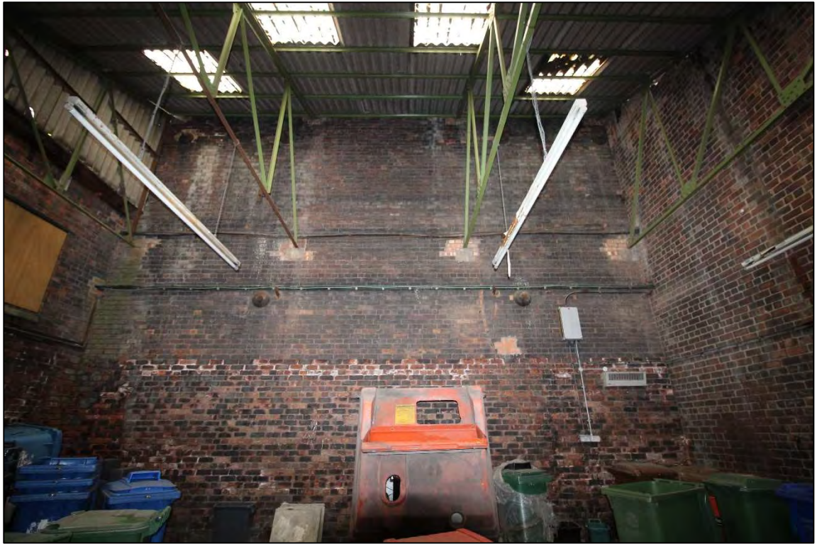
Plate 98: General view of Room 2 within the lean-to, facing north
