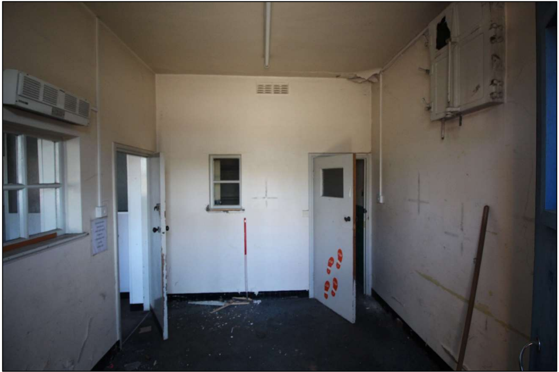
Plate 54: General view of Room 1, facing north
