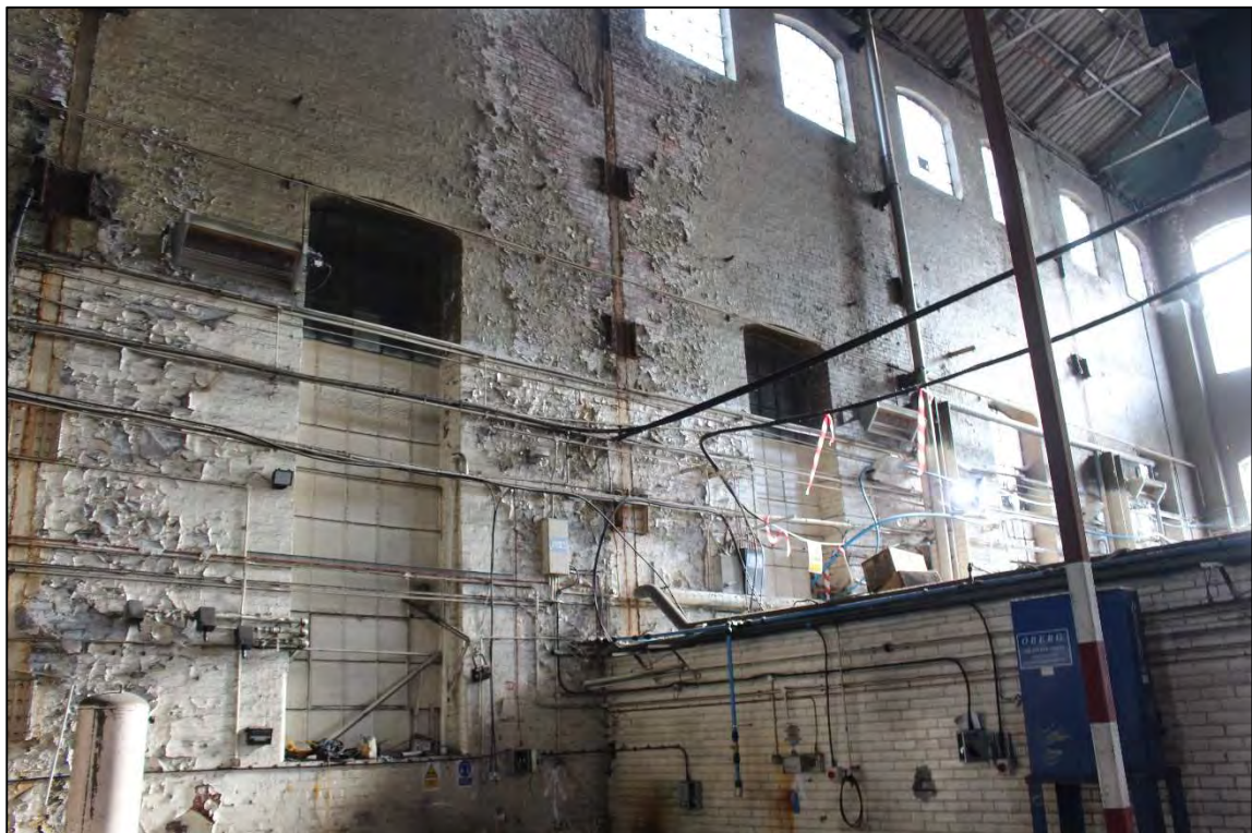
Plate 87: The infilled windows within the northern wall of the riveting bay
