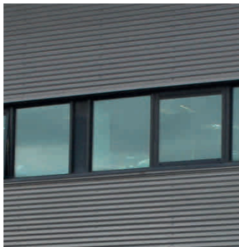
Double glazed window in polyester powder-coated aluminium frames
