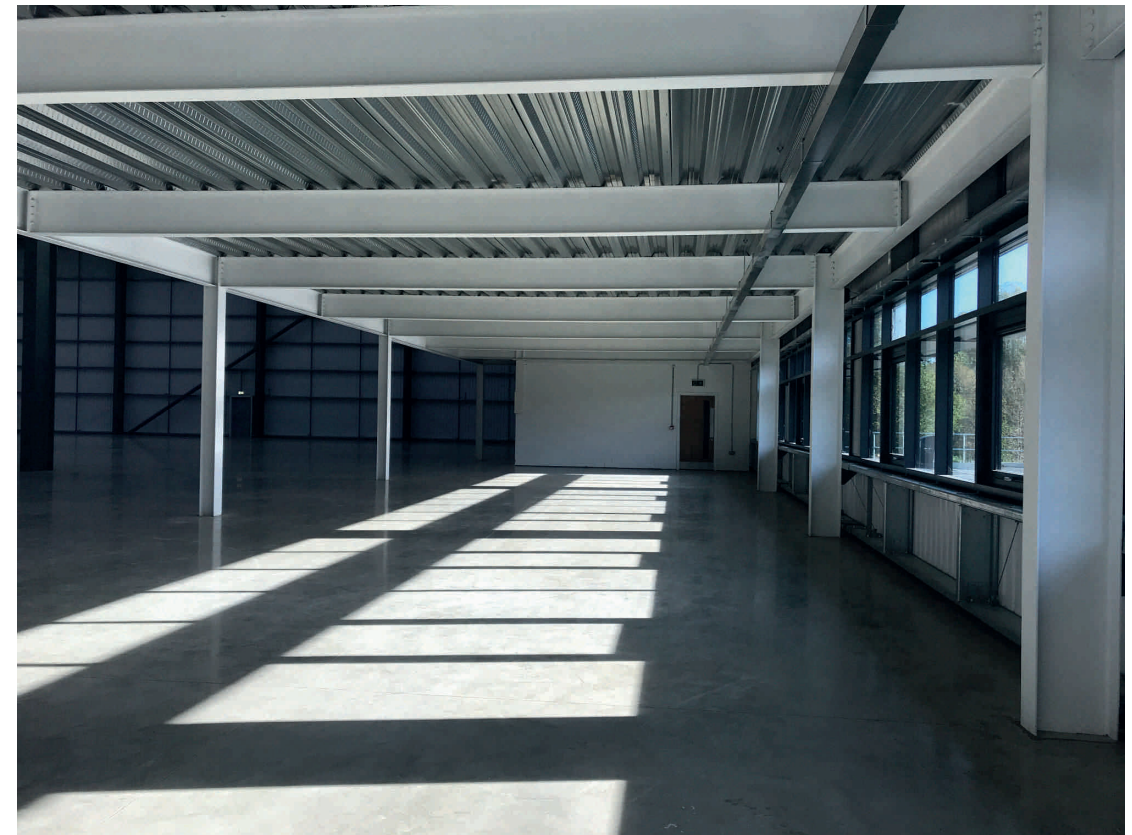
Typical office undercroft area within warehouse
