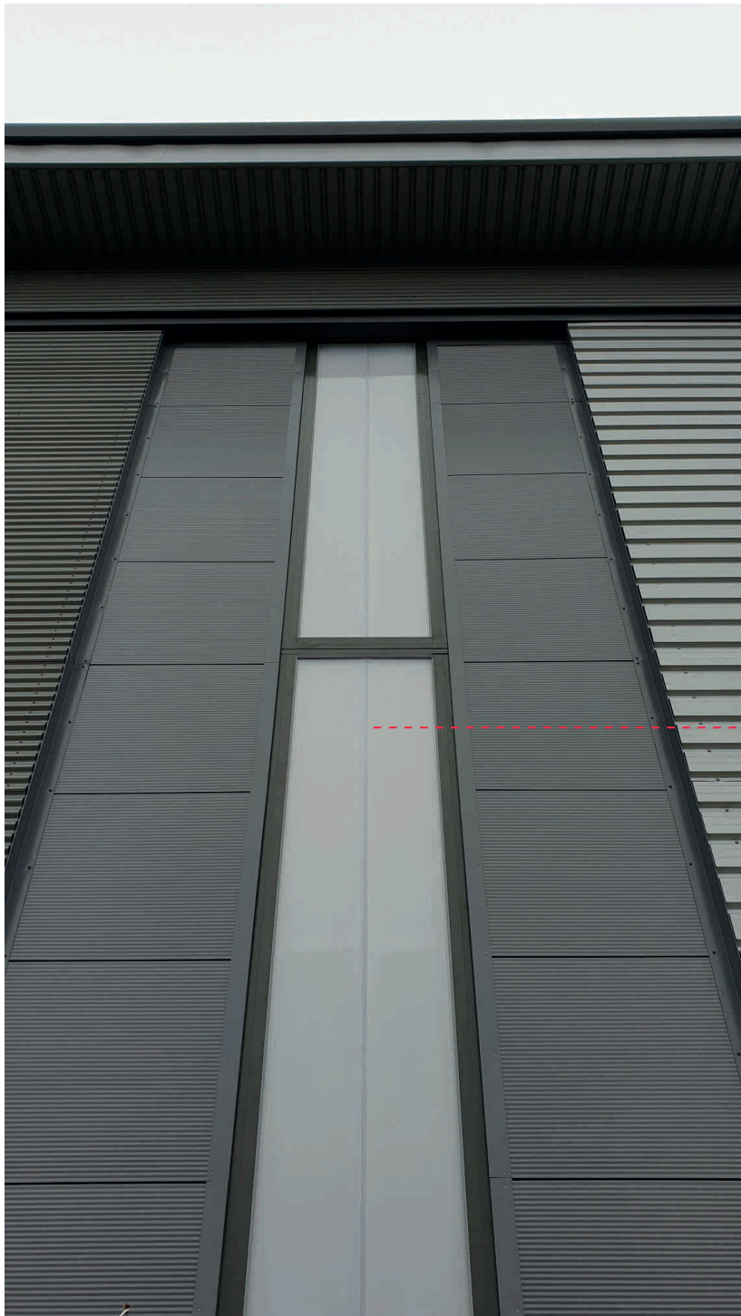
External view of translucent Feature Panel (Kingspan “Day-Lite” or similar)
