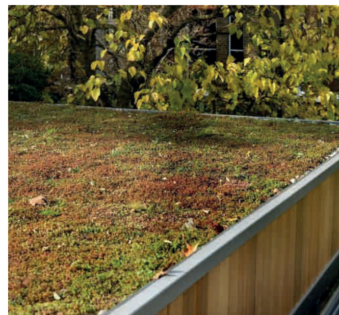
Sedum roofs above cycle shelters and projecting office areas
