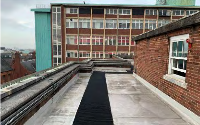
ABOVE: THE EXISTING UN-INSULATED ROOF (WITH PARAPET) ABOVE THE THIRD FLOOR BELOW: ILLUSTRATION OF THE BAUDER TOTAL ROOF SYSTEM BUILD-UP AS PROPOSED FOR ALL FLAT ROOF REPLACEMENTS AT THE ZOCHONIS BUILDING
