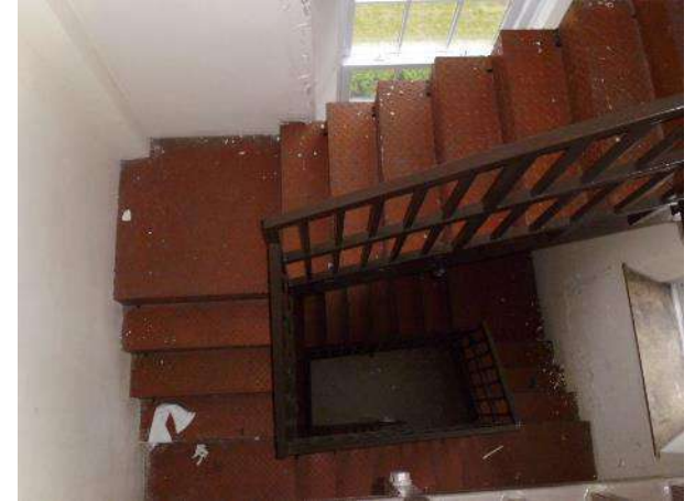
Escape Stair to South East corner of Zochonis Building
