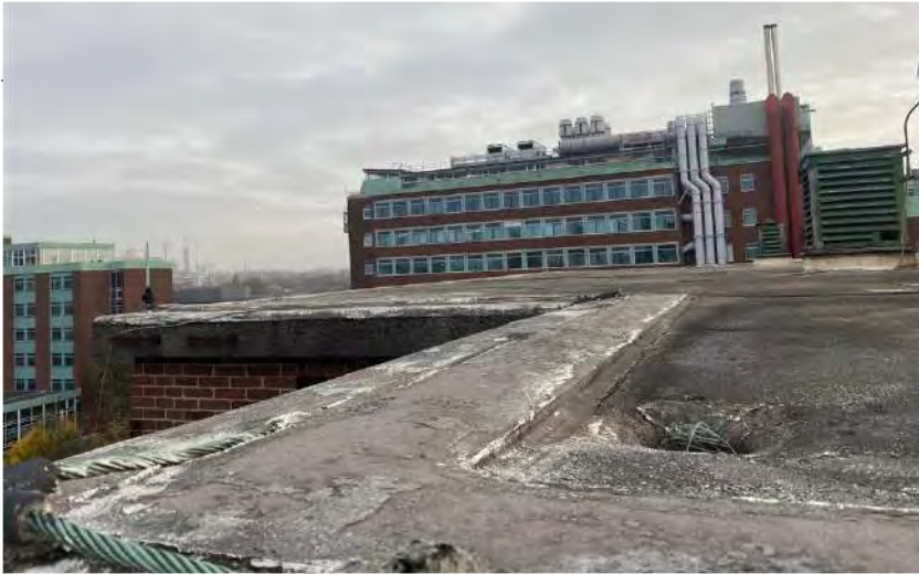
ABOVE: THE EXISTING UN-INSULATED ROOF (NO PARAPET) TO THE PLANT ROOM BELOW: A PREVIOUS INSTALLATION OF THE BAUDER TOTAL ROOF SYSTEM AND BAUDERSOLAR TOGETHER WITH EDGE PROTECTION
