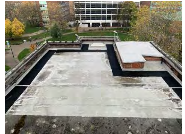
Area of flat roof to North-East corner of Zochonis Building showing ancillary rooftop accommodation
