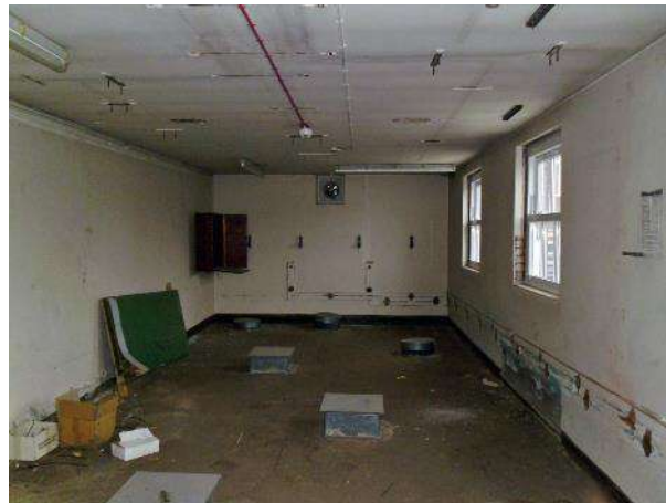
Store room adjacent to Central Plant Room
