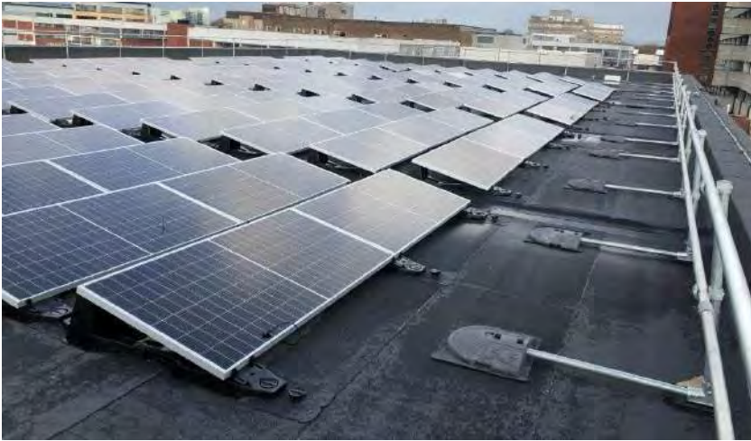
ABOVE: THE EXISTING UN-INSULATED ROOF (NO PARAPET) TO THE PLANT ROOM BELOW: A PREVIOUS INSTALLATION OF THE BAUDER TOTAL ROOF SYSTEM AND BAUDERSOLAR TOGETHER WITH EDGE PROTECTION
