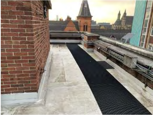
Existing roof covering adjacent to plant room
