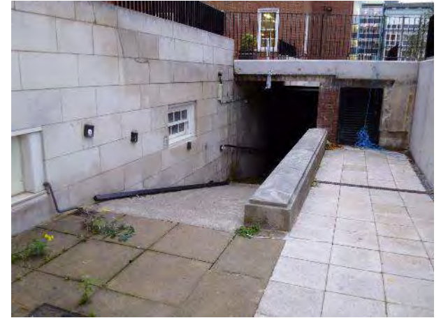
Access to High Voltage Sub-Station at Basement Level
