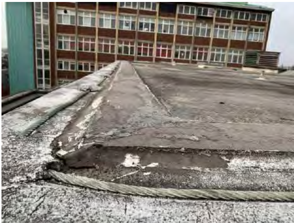
Existing roof covering to edge of upper plant room roof including lightning protection cable
