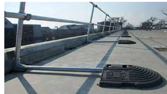
BELOW: 'KEEGAURD' TYPE EDGE PROTECTION FORMED FROM GALVANISED TUBES AND COUNTER-WEIGHT CONNECTIONS
