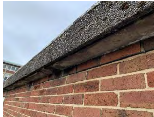
Existing 'eaves/soffit' detail to edge of upper plant room roof
