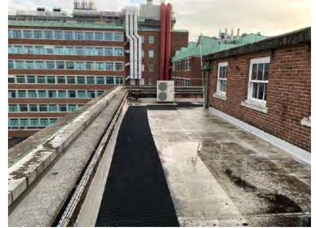
Existing AHU units as located on existing roof adjacent to plant room wing to be demolished
