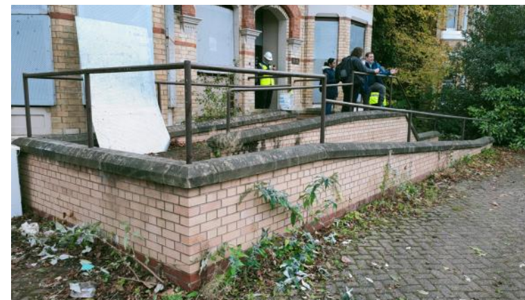
Ramp and steps at front of building
