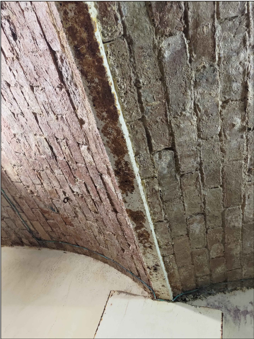
EXISTING CONDITION PHOTO SCALE N.T.S
