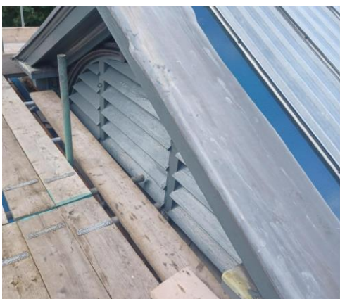
Redecoration work to roof level joinery
