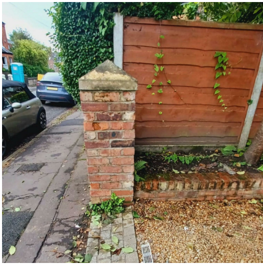
EXISTING BRICK PIER
