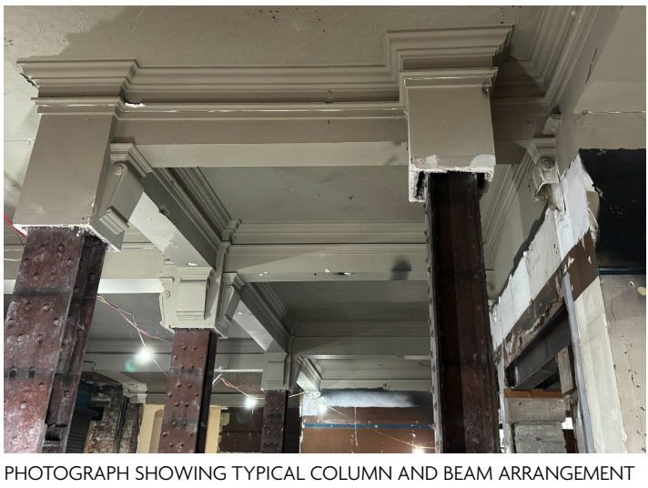
PHOTOGRAPH SHOWING TYPICAL COLUMN AND BEAM ARRANGEMENT
