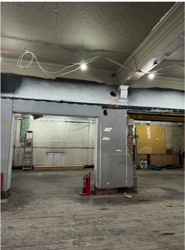
PHOTOGRAPH SHOWING TYPICAL OPENING ARRANGEMENT
