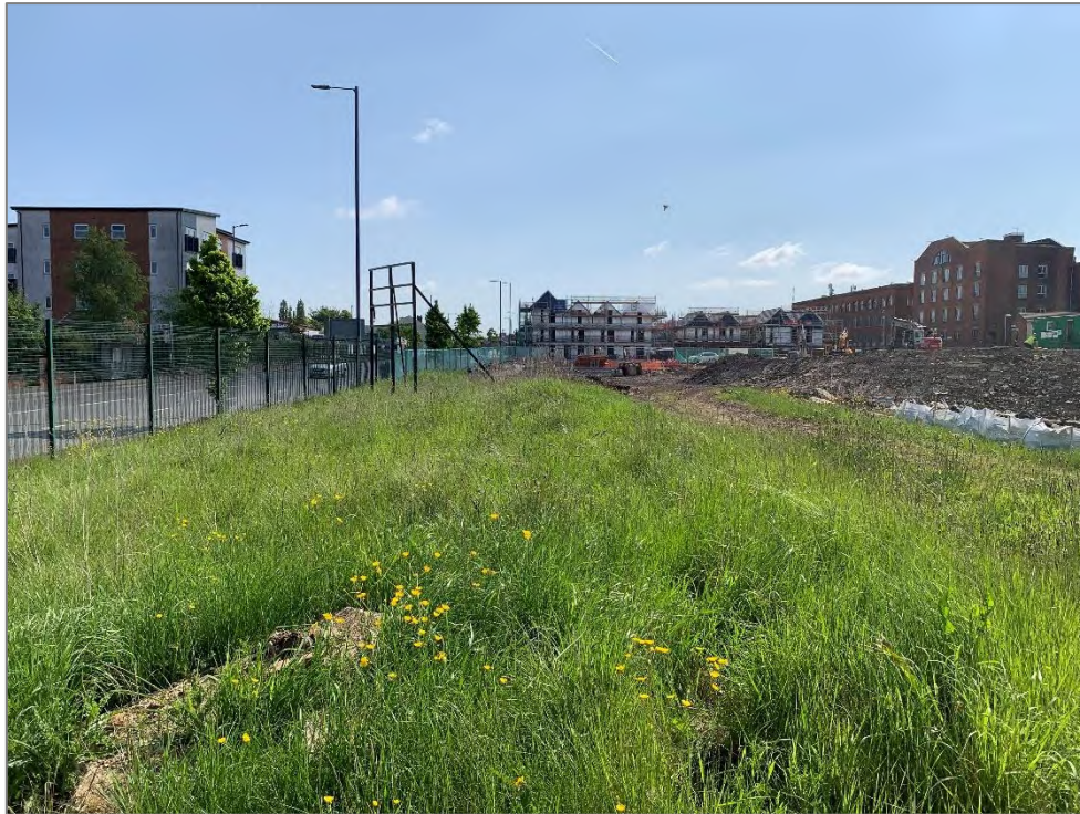
Photograph 3: View east across Phase 2, from northwest corner
