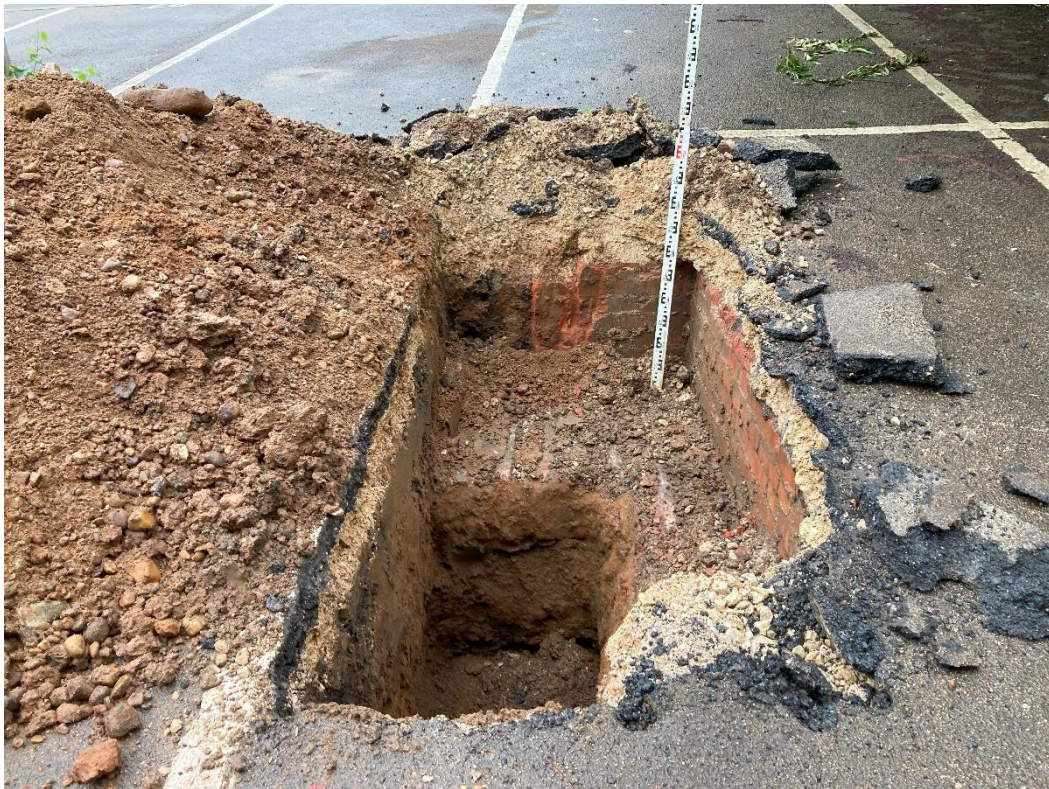
Plate 4 - TP02 relic in-situ brick wall and footing.
