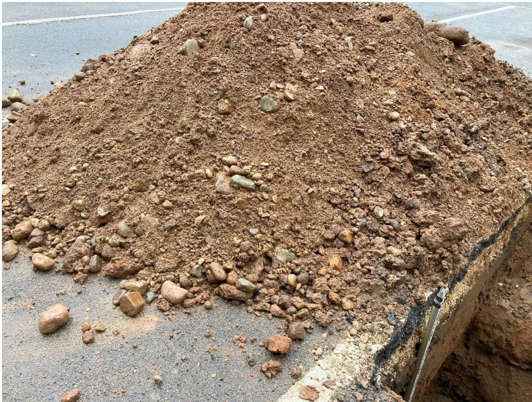
Plate 1 – Trial Pit (TP) 02 arisings.
