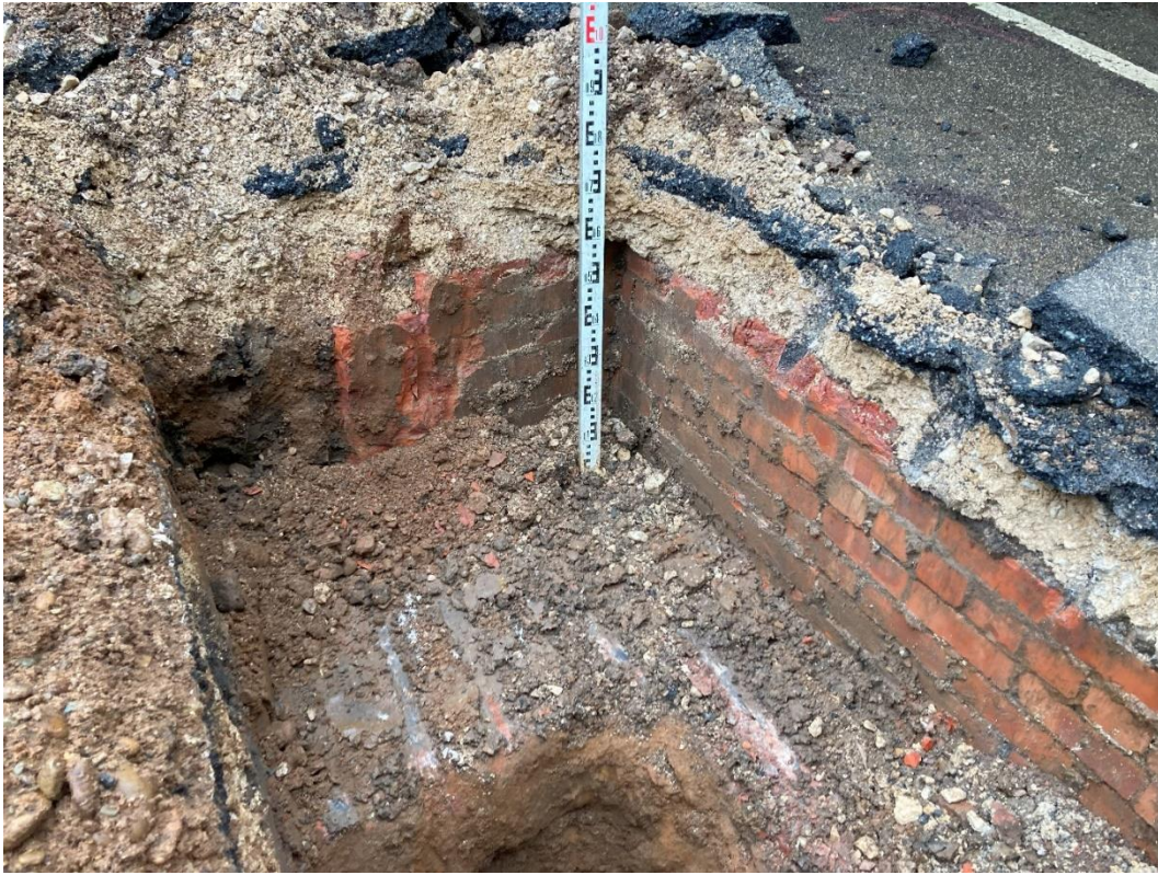
Plate 3 – TP02 relic in-situ brick wall, gl to 0.8m bgl.
