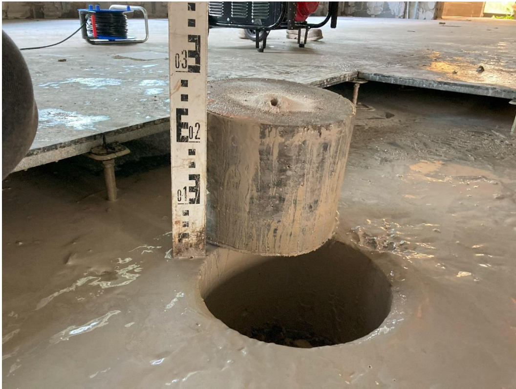
Plate 25 - WS13 concrete core, gl to 0.25m bgl.
