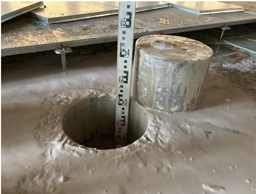
Plate 28 - WS15 concrete core, gl to 0.22m bgl.
