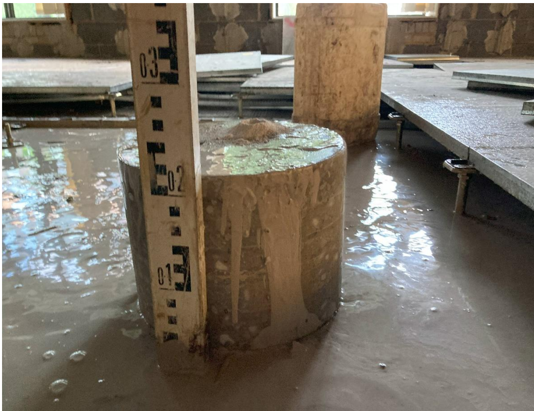
Plate 30 - WS16 concrete core, gl to 0.22m bgl.
