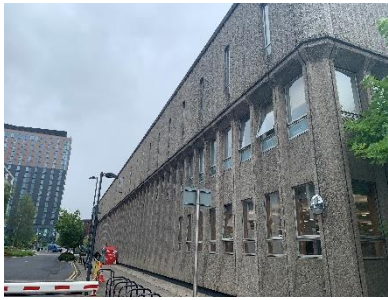
Photograph 1 – The building's Exterior
