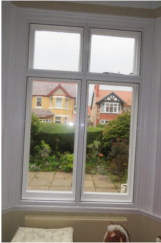
*Example of a white aluminium 'click out' secondary glazed system
