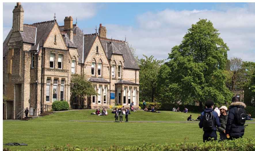
Marylands Building at Xaverian (Grade II Listed)
