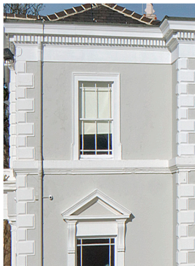
Tall symmetrical narrow windows. High level dentilled cornice banding detail . Mid level sill-band
