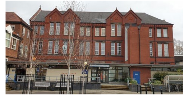
Firwood Building (Grade II Listed) on Xaverian College Campus
