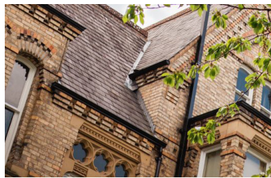
Red brick banding with feature window headbanding and protruding corbell details.
