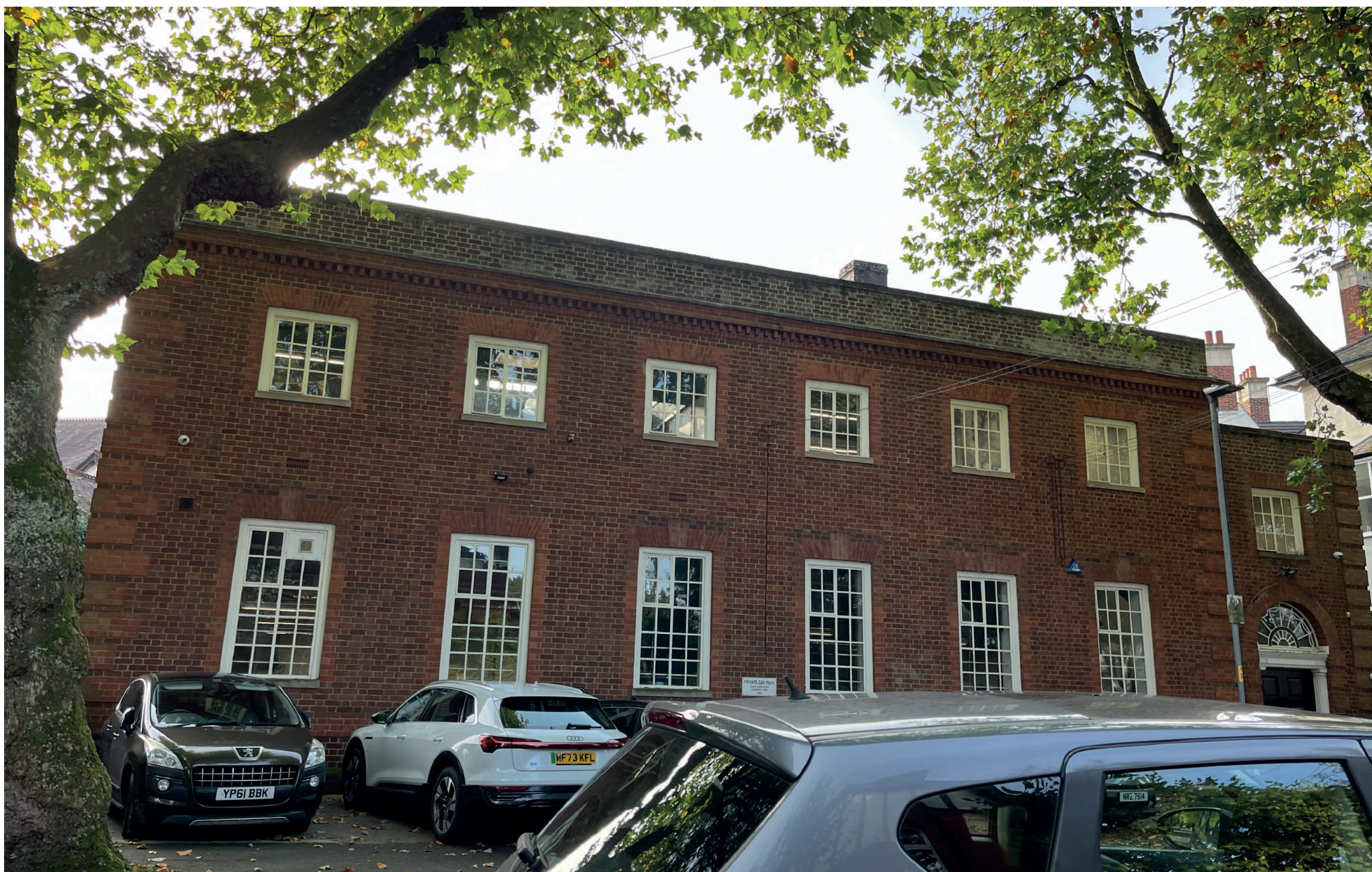
Ballbrook Avenue elevation to Craig House
