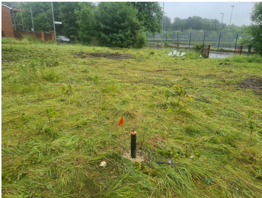
PLATE 10 WS104 MONITORING WELL
