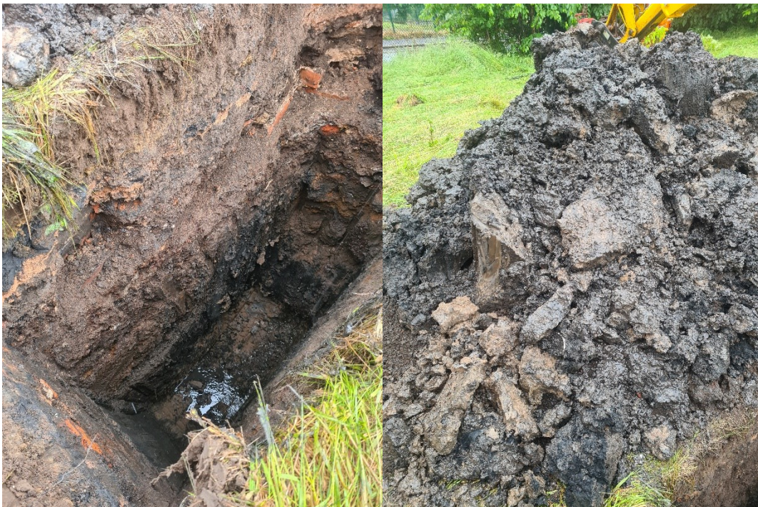
PLATE 6 TP103 EXCAVATION AND ARISING
