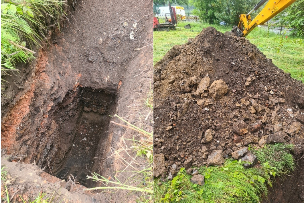
PLATE 5 TP104 EXCAVATION AND ARISING
