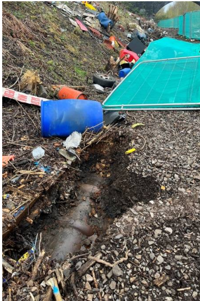
B. Clay pipe work of culverted section of drain
