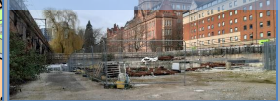
The western elevation of Bainbridge House adjoins the eastern edge of the site
