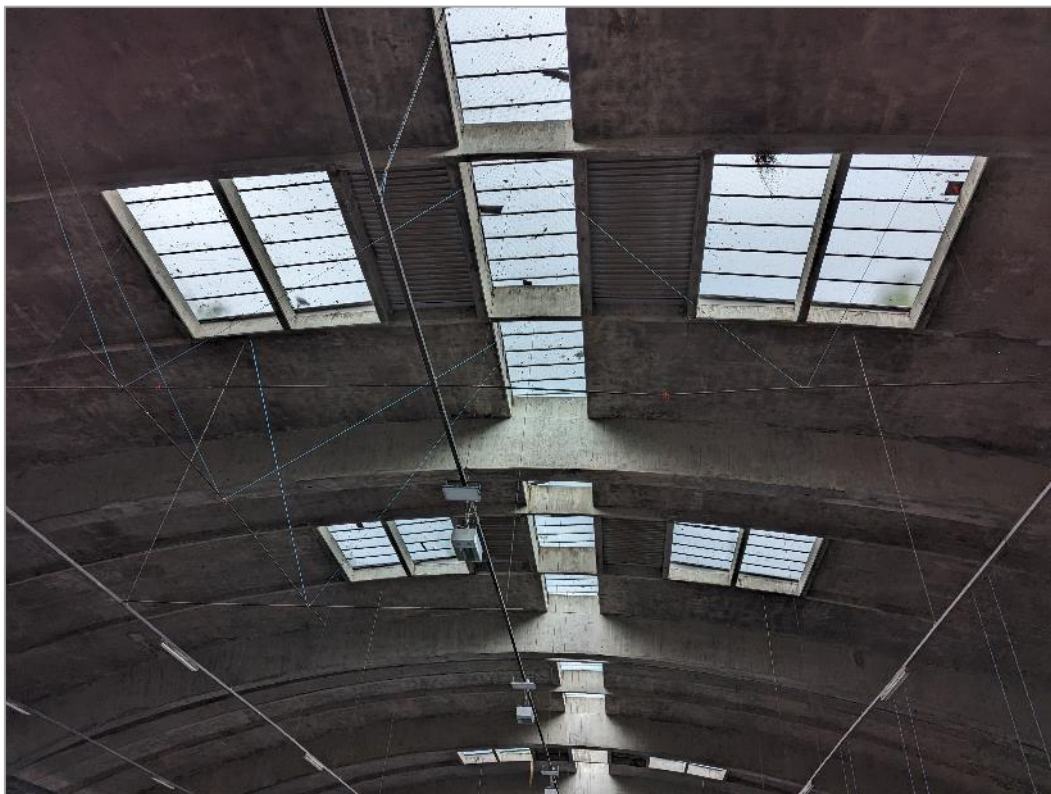
Plate 2 – Nature of the roof underside with prism sunlights
