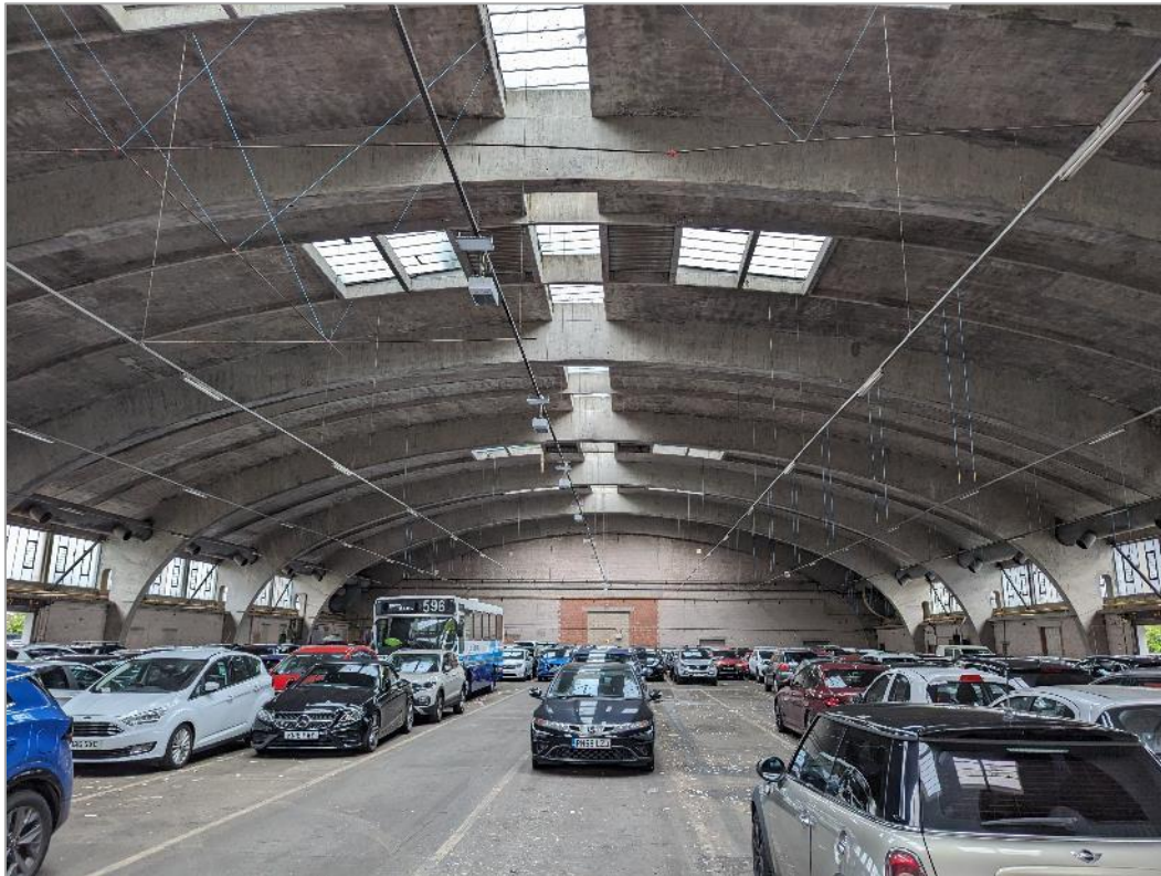
Plate 1 – Interior of bus garage from south looking north to bricked up area
