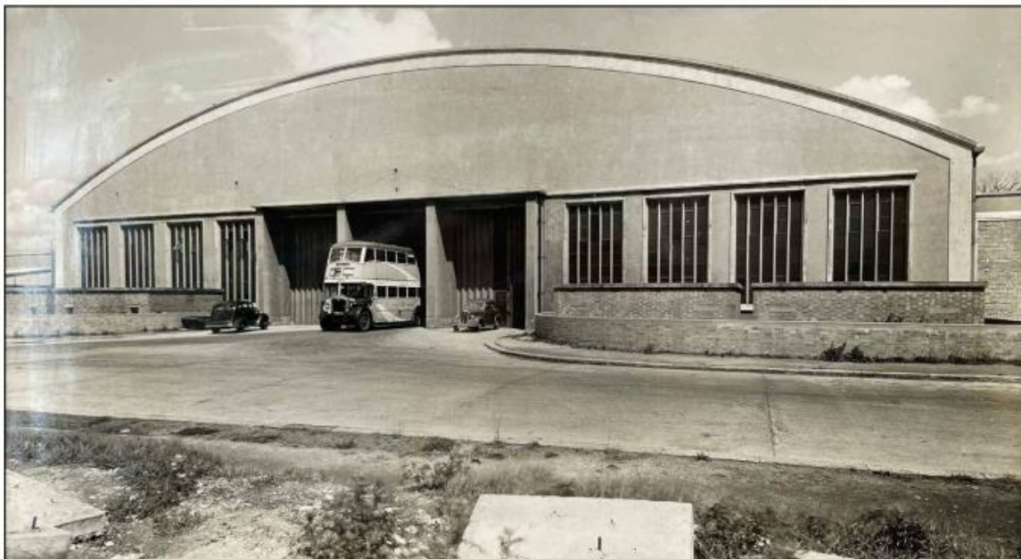
Figure 1.1 - Wythenshawe bus garage, historic image from 1950s
