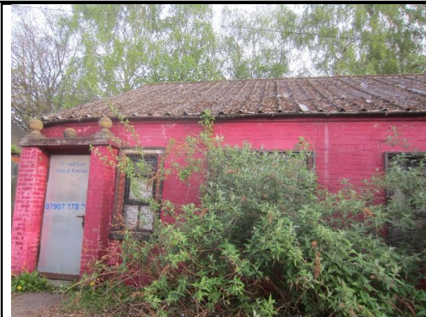
Photo 13: Northern elevation of B3
