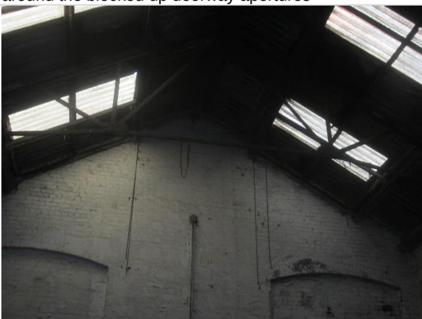
Photo 29: skylights create a light interior at B4
