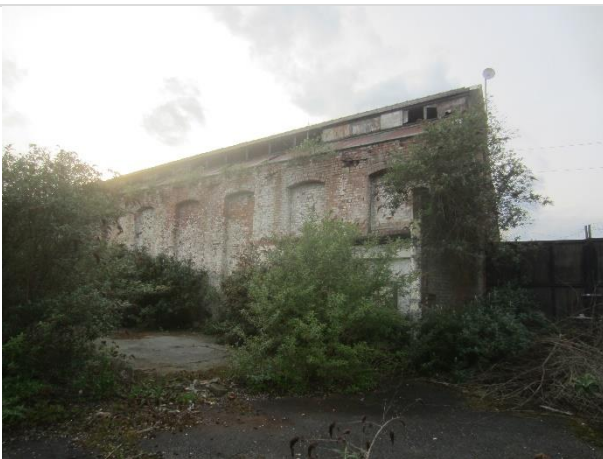
Photo 21: Southern elevation of B4
