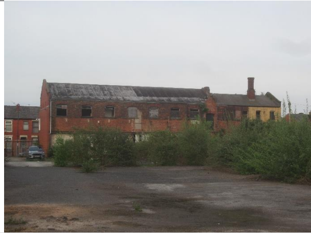
Photo 1: Western elevation of B1
