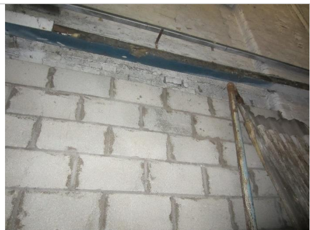
Photo 30: Well-pointed walls in interior of B4
