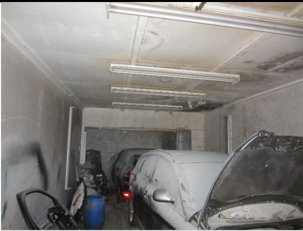
Photo 19: Interior of B3
