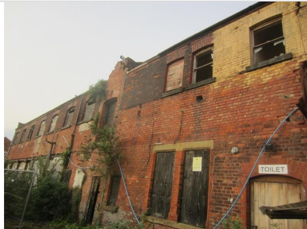
Photo 3: Western elevation of B1
