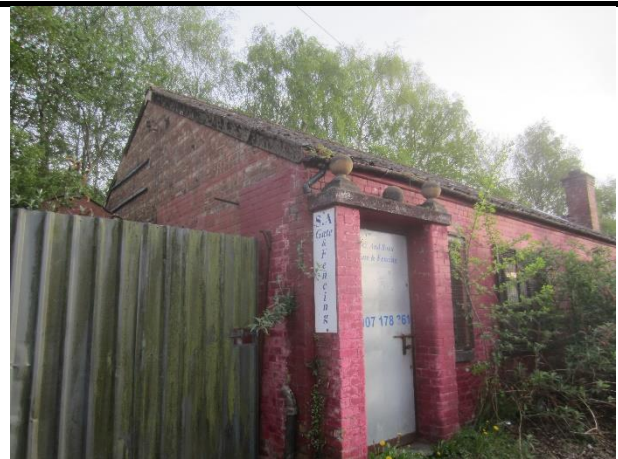
Photo 14: Eastern and southern elevations of B3 showing overlapping fascia at gable end
