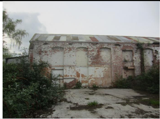
Photo 20: Southern elevation and roof of B4
