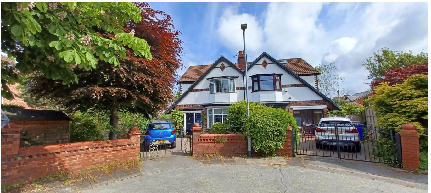
Figure 1. Principal elevation of No.24 Mayville Drive.
