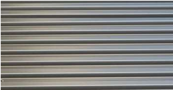
2. Corrugated/Louvred metal panels
