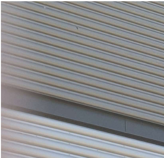
2. Louvre/corrugated metal panel
