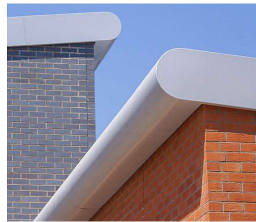
1. Standing seam roof
