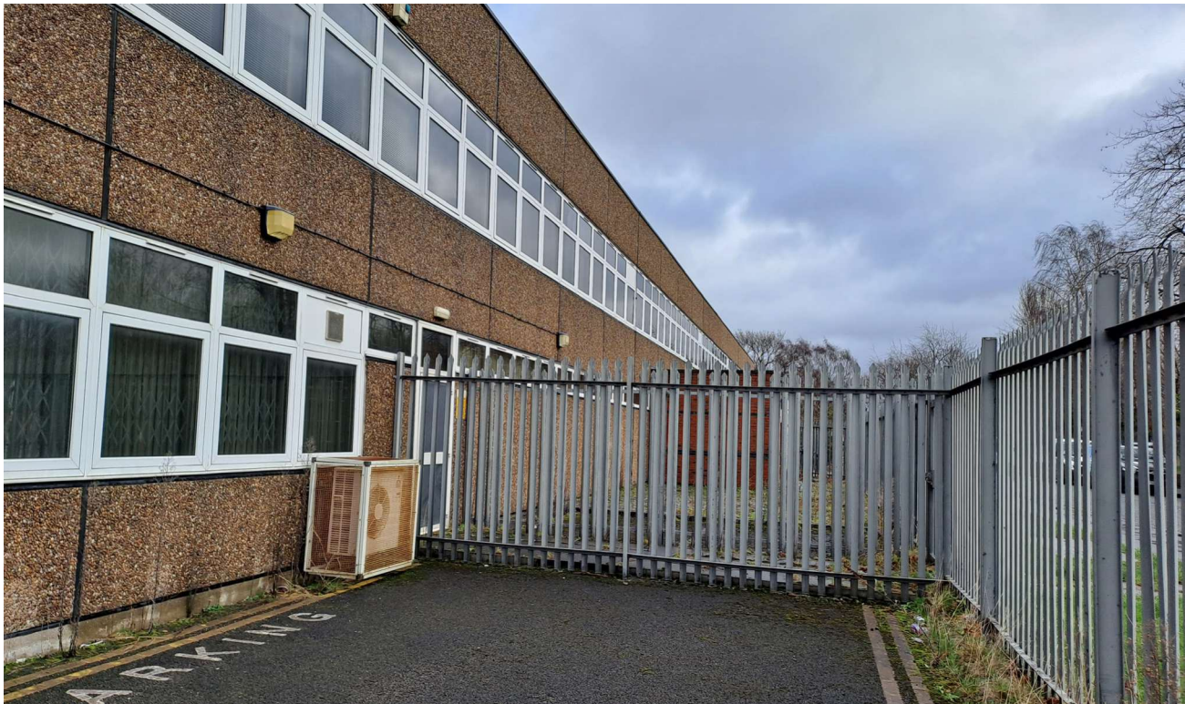
View of existing Southern elevation and fencing
