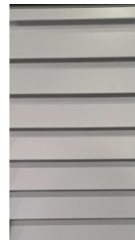
2. Corrugated/Louvred metal panels
