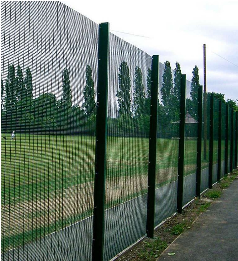
Image of security rated anti climb fencing
