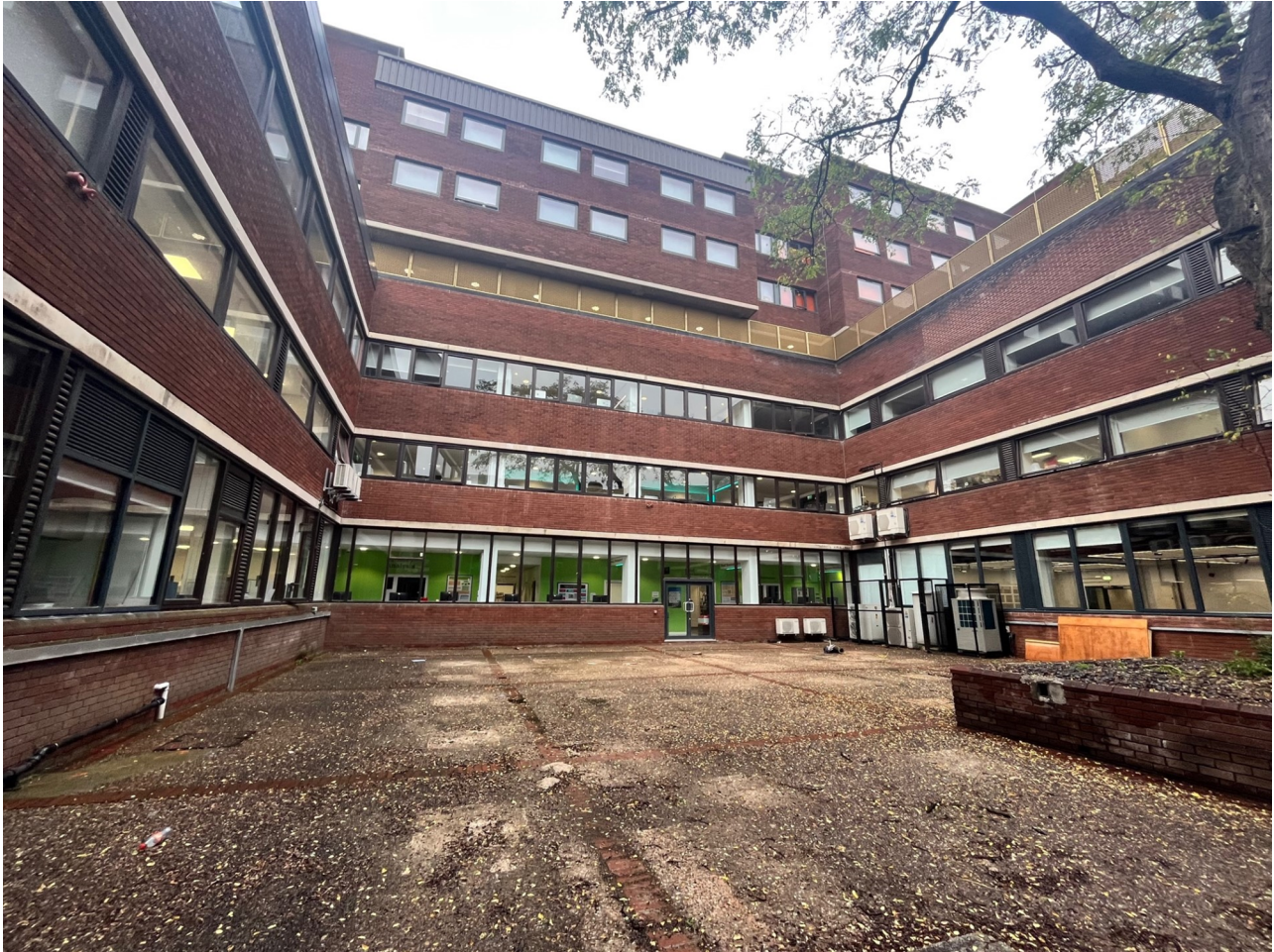
Existing Site (Following Removal of Structures Approved under 106313/FO/2014/C1)
