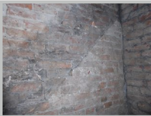
Plate 14. Shadow line of former staircase
