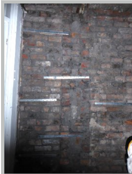
Plate 11. Straight joints
