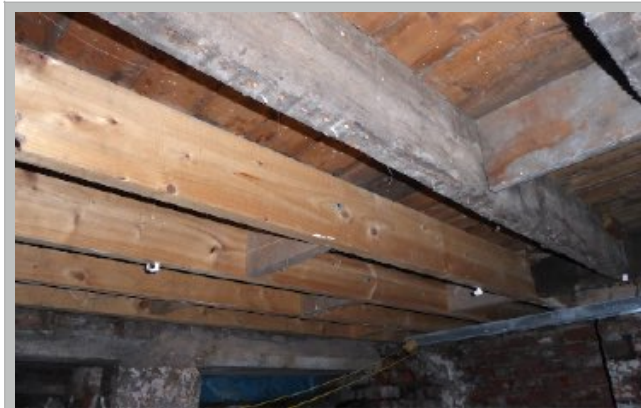
Plate 13. New floor joists in N front room
