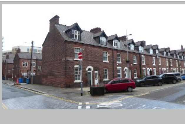
Plate 18 Terrace houses further N
