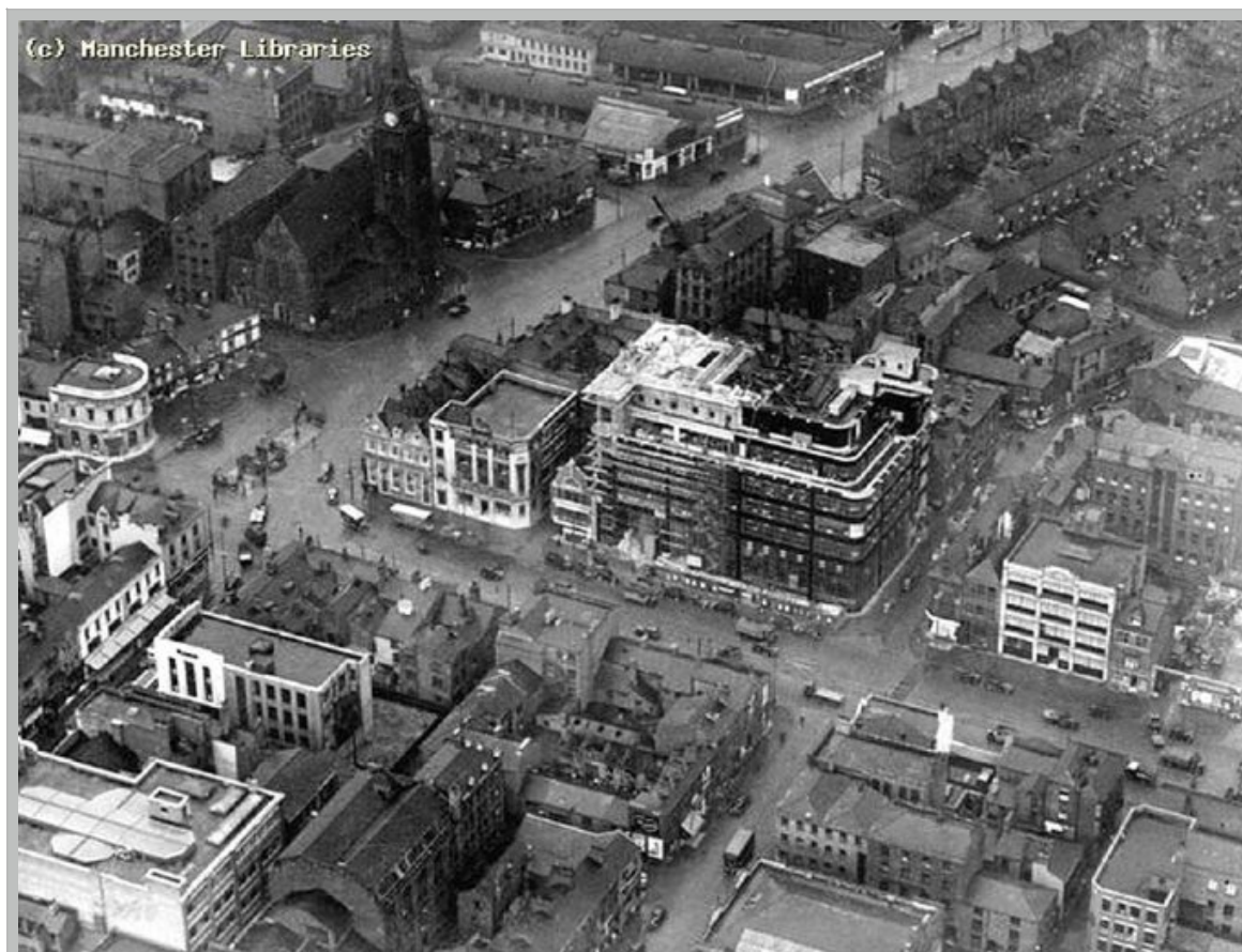
Plate 36. Aerial photo with no. 39 in bottom R with dormer
