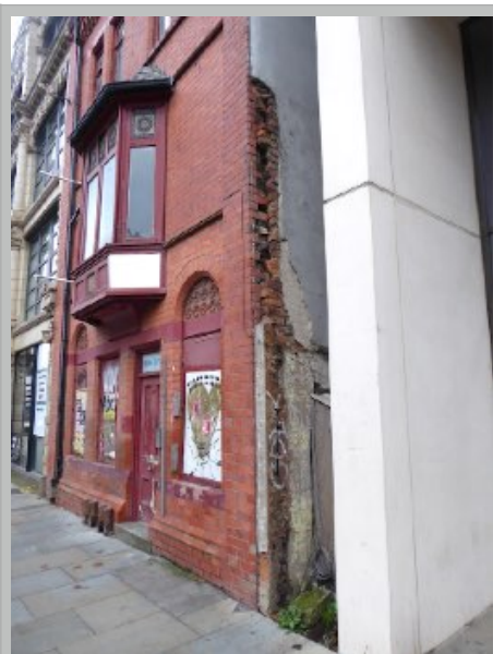
Plate 6. Front elevation not fully keyed into the side elevation
